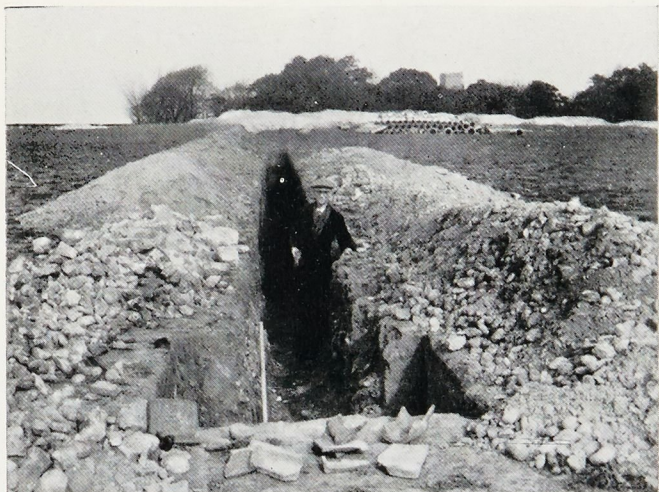
Looking eastward along the first trench dug. April, 1935.
