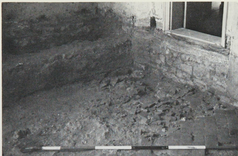
PLATE G.1 Remains of tiled floor, scale in feet. Photo D. Sherlock
