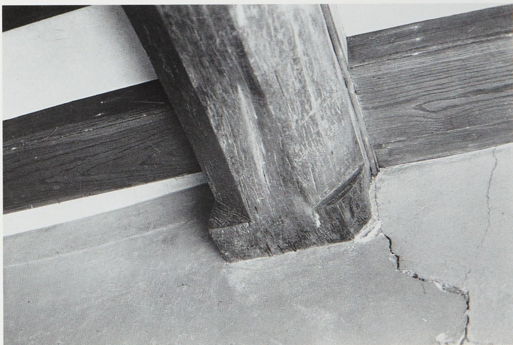
Plate XVI Detail of transverse joist in central room showing straight chamfer stop.
