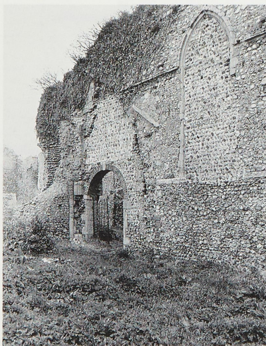
Plate II Chancel and former south transept from south-east showing position of eastern aisle and the partly encased crossing pier. In the foreground first phase masonry.
