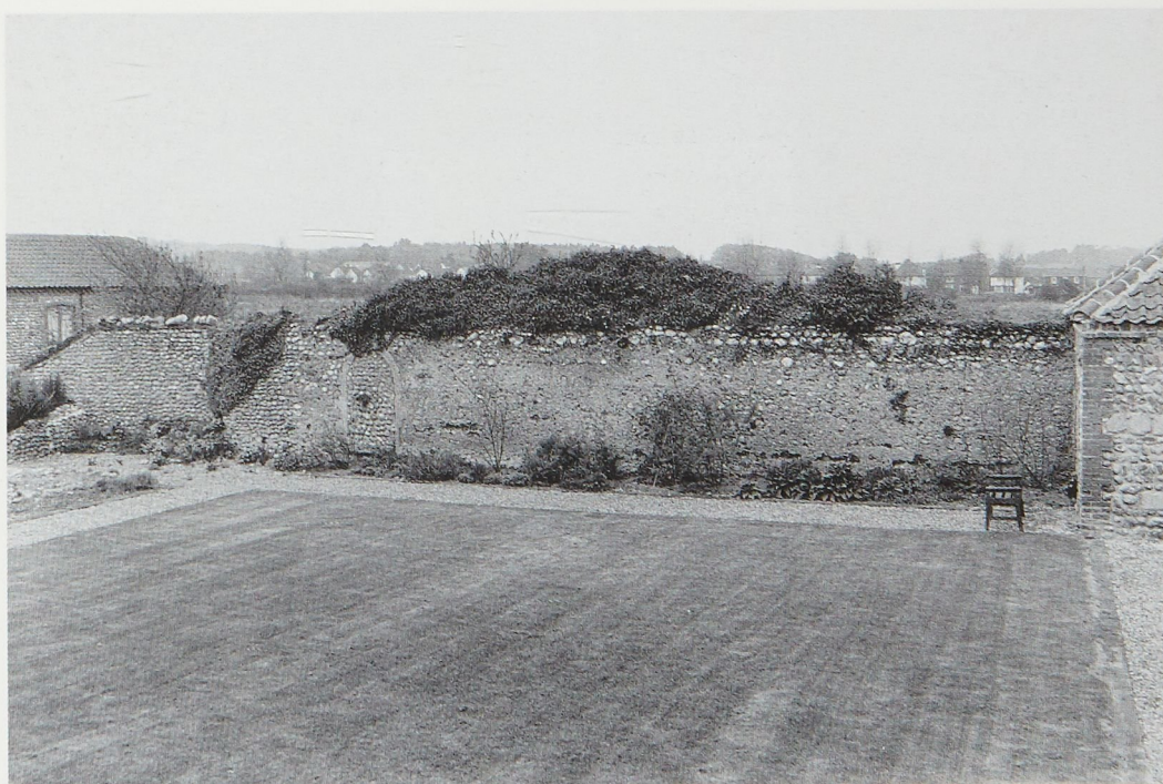
Plate XII East wall of west range of former cloister from east.
