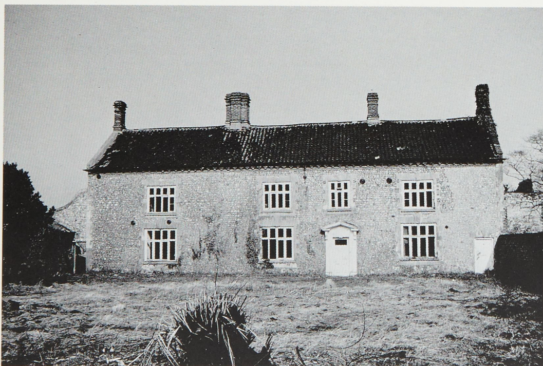
Plate XIV Facade of farmhouse before restoration.
