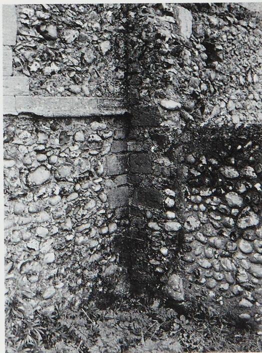
Plate IV Internal quoins of brick in north-east corner of chancel.
