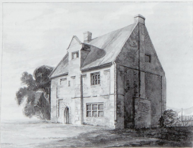
Figure 4. View of Winnold House from the south-east by George Cattermole (1800-1868). BL Add MS 23047, f.189.
