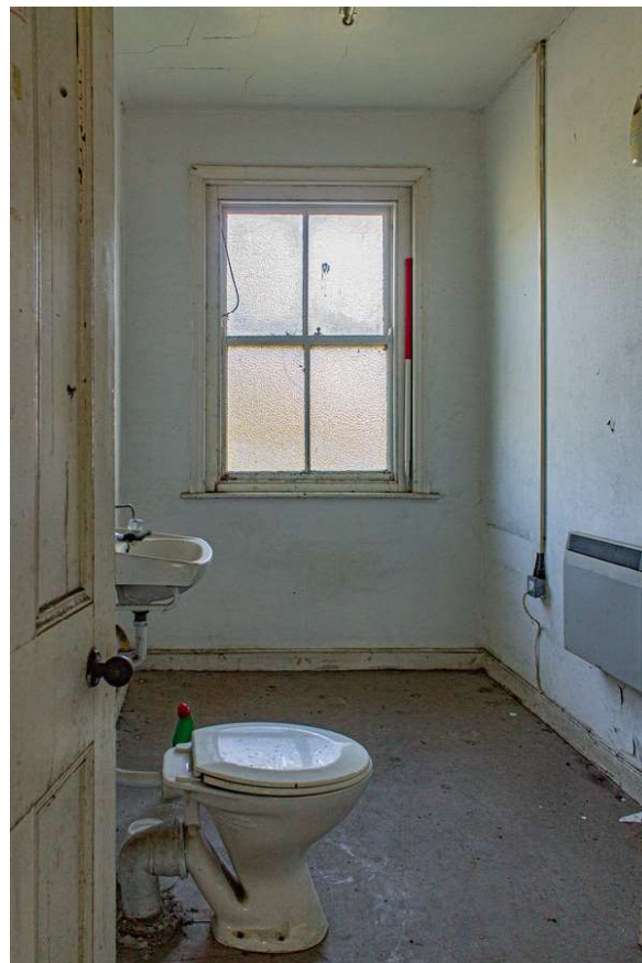
Plate 20 (20): Building A (Cottage), general view of Room A3 from the south-west
