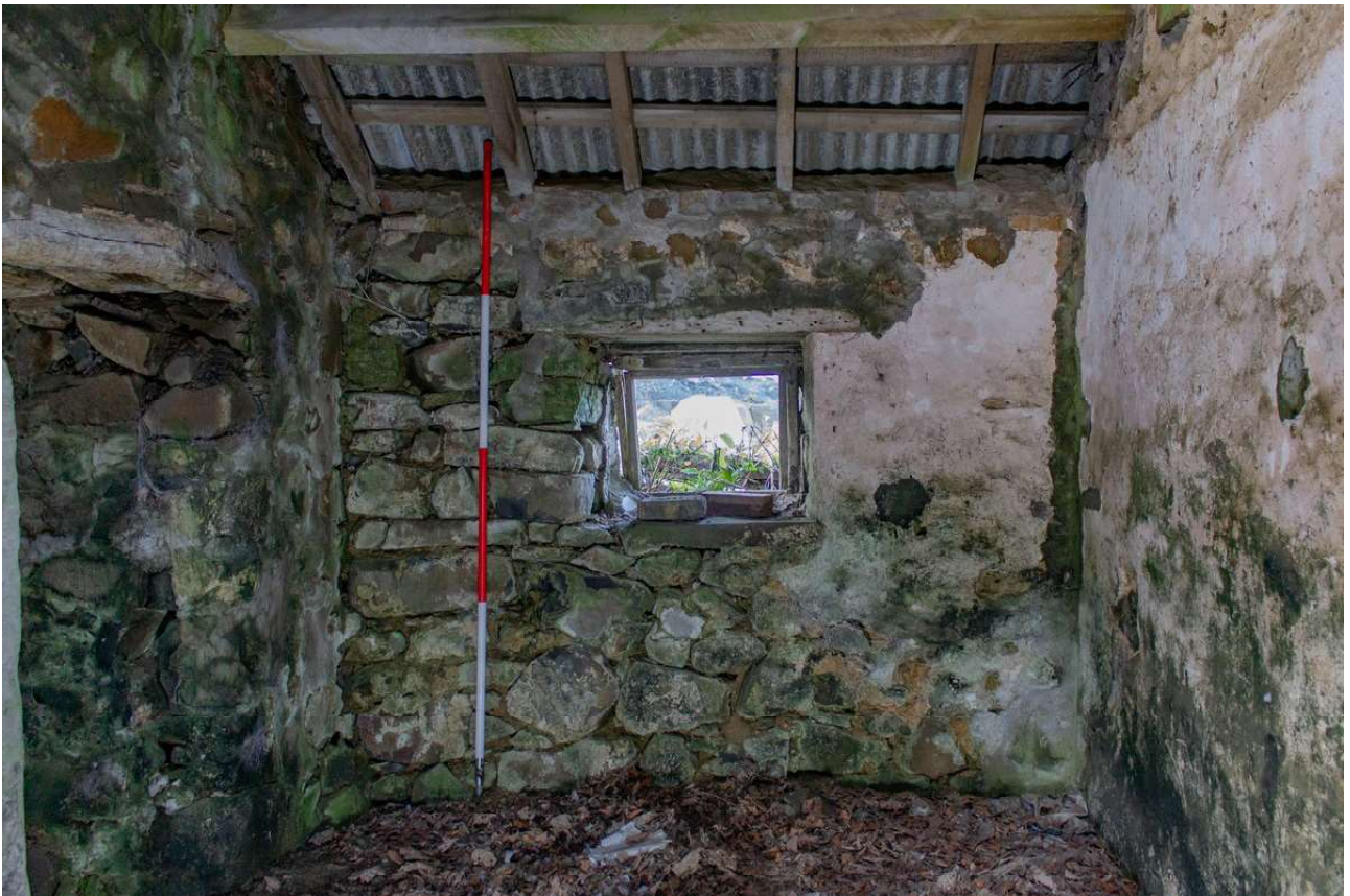
Plate 68 (68): Building B (Barn), Barn B3, general view from the south-west
