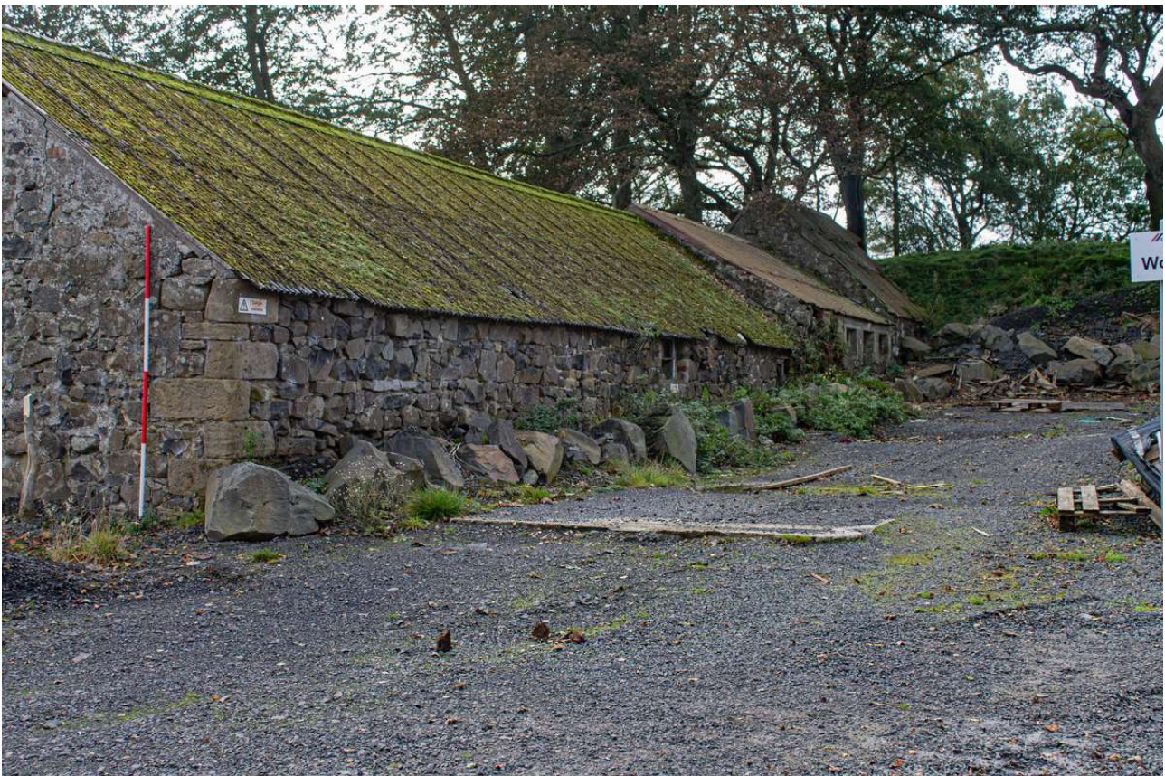
Plate 36 (38): Building B (Barn), general view of the north-west elevation from the north
