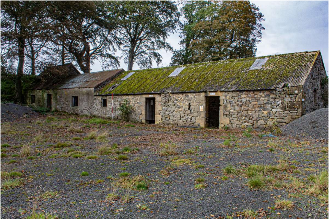
Plate 29 (29): Building B (Barn), general view from the east
