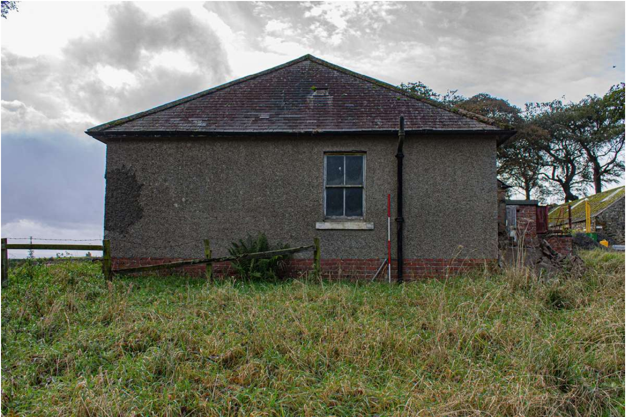
Plate 9 (04): Building A (Cottage), general view of the north-east elevation, from the north-east
