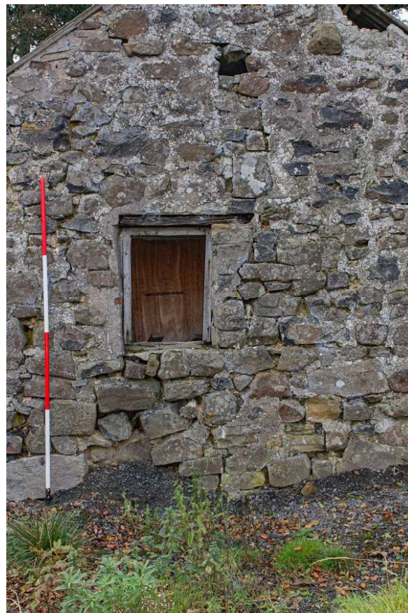
Plate 46 (36): Building B (Barn), detail of the boarded window in the north-east gable, from the north-east
