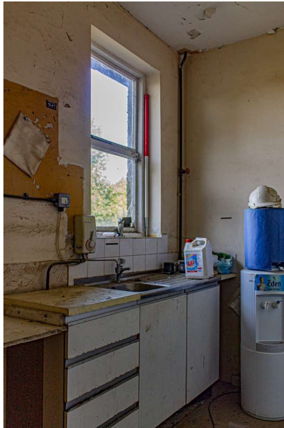
Plate 21 (21): Building A (Cottage), general view of Room A4 from the WSW
