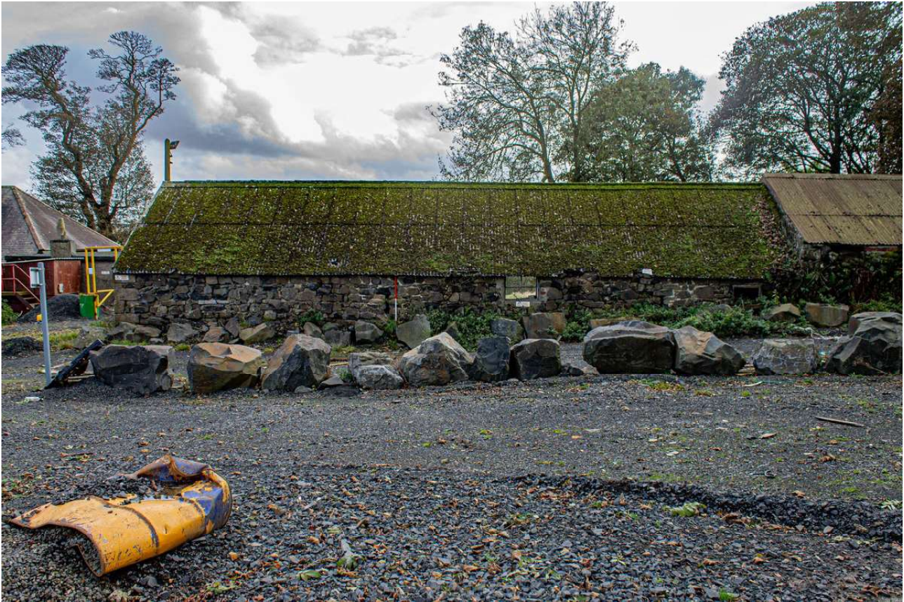
Plate 37 (39): Building B (Barn), general view of the north-east side of the north-west elevation, from the north-west
