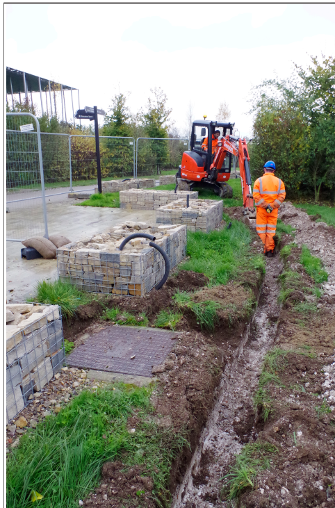
Plate 2: Working shot of cable trench excavation, view from the north
