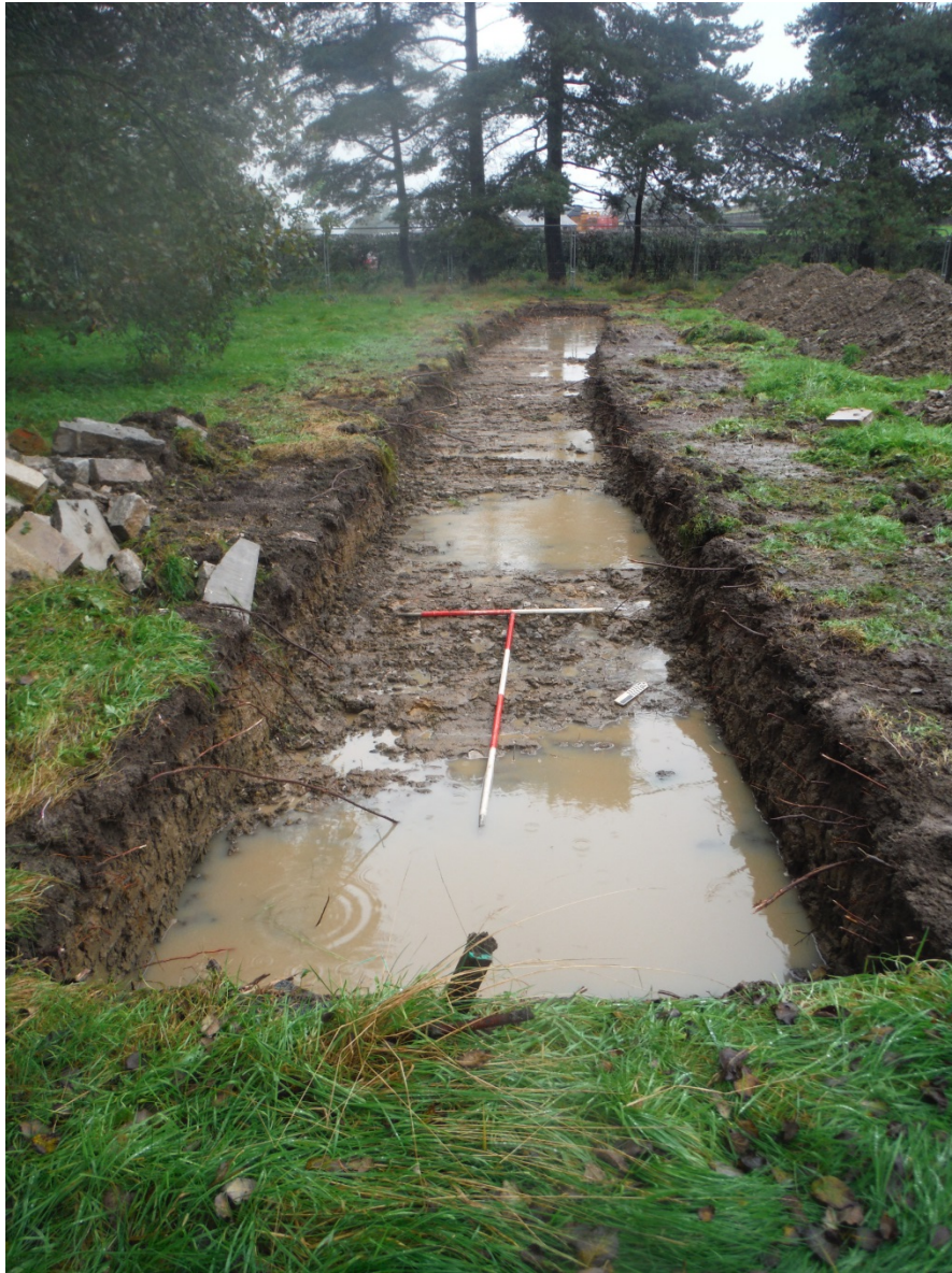
Figure 9. Trench 1. View to NW
