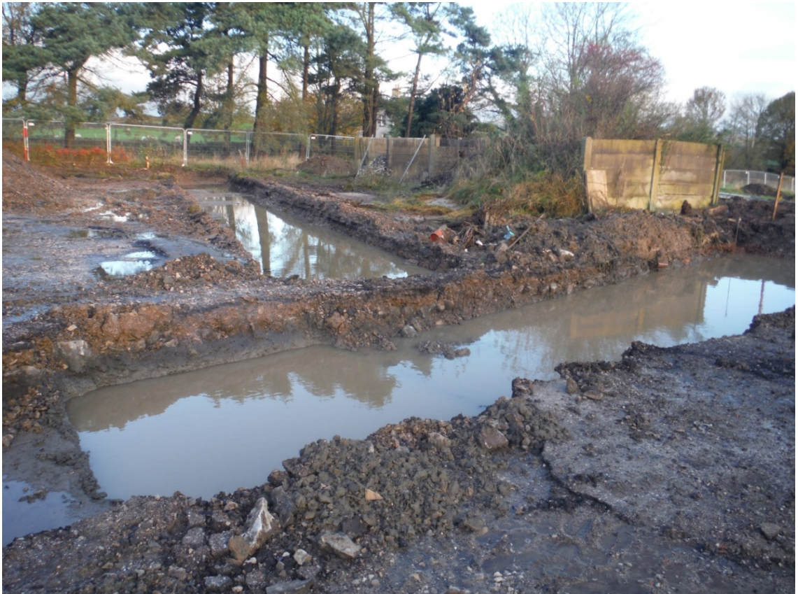
Figure 43. Working shot of flooded trenches.
