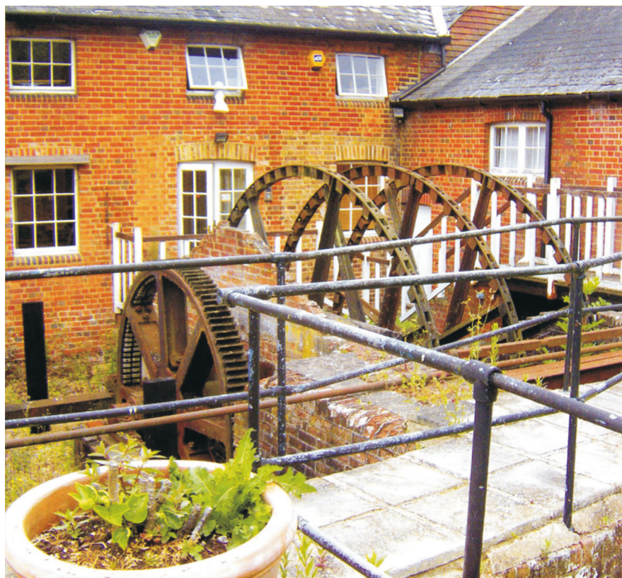
Fig 4 Downside Mill, Cobham. The obsolete water wheels on the south side of the later 18th century phase of Alexander Raby's iron mill at Downside. (Photograph by Andrew Norris, 2008)
