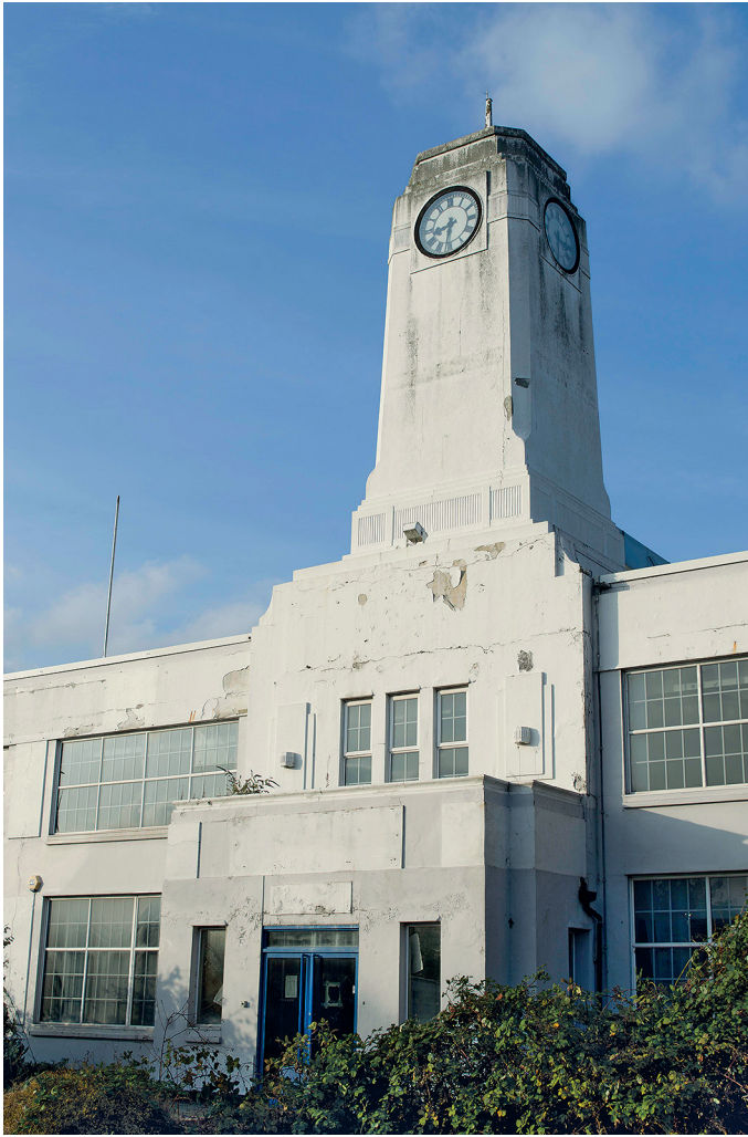
Fig 8 Former Thales Avionics Offices. The principal southern elevation, of two storeys and a central clock tower in the Art Deco style. (Photograph © ASE)
