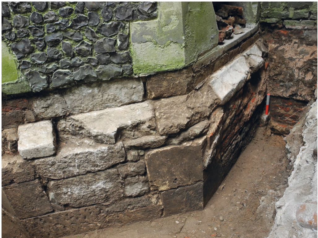
Fig 6 St Mary Magdalene Church, Paradise Road, Richmond upon Thames. Face of original Tudor tower exposed with later knapped flint face, facing east. (Photograph by MOLA)
