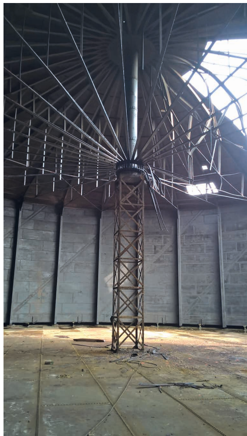
Fig 10 Land at Wrythe Lane (B278), Carshalton. View of the interior spiral-guided design of the 1930s gasholder. (Photograph by ASE)
