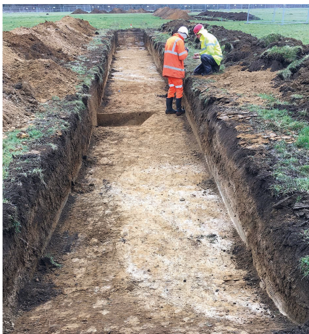
Fig 3 River Thames Flood Alleviation Scheme, Desborough Island, Walton Lane, Walton-on-Thames. N Randall (right), SCC Archaeological Officer, examines prehistoric pottery recovered from the fill of a ring ditch feature, possibly a Bronze Age barrow, visible in the foreground and under excavation during a trial trench evaluation (Photograph by C Charman, Environment Agency)
