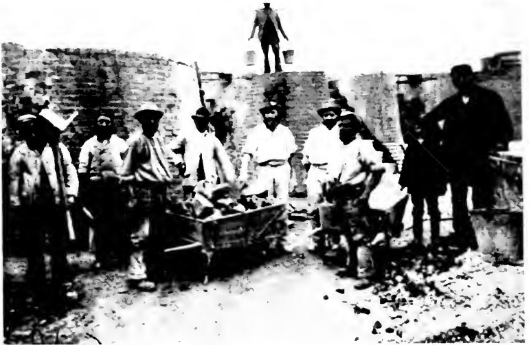
(a) CONSTRUCTION OF HOFFMAN KILN AT BETCHWORTH, c.1865.
