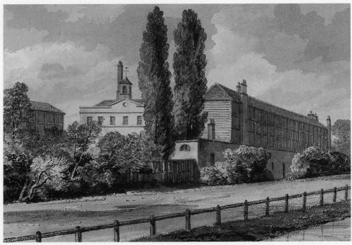
Fig 9 Pen and wash drawing, dated 1826, of Neckinger Mill by John Chessell Buckler. At that time Bevingtons used the mill as a leather works but the buildings illustrated appear to be those described in the 1805 sale particulars of the paper mill. Note in particular the drying lofts at the right and extreme left, and the steam engine house with the turret and chimney stack to the left of the tall trees. The view is from the north-east. Courtesy of Southwark Local Studies Library, P4288.
