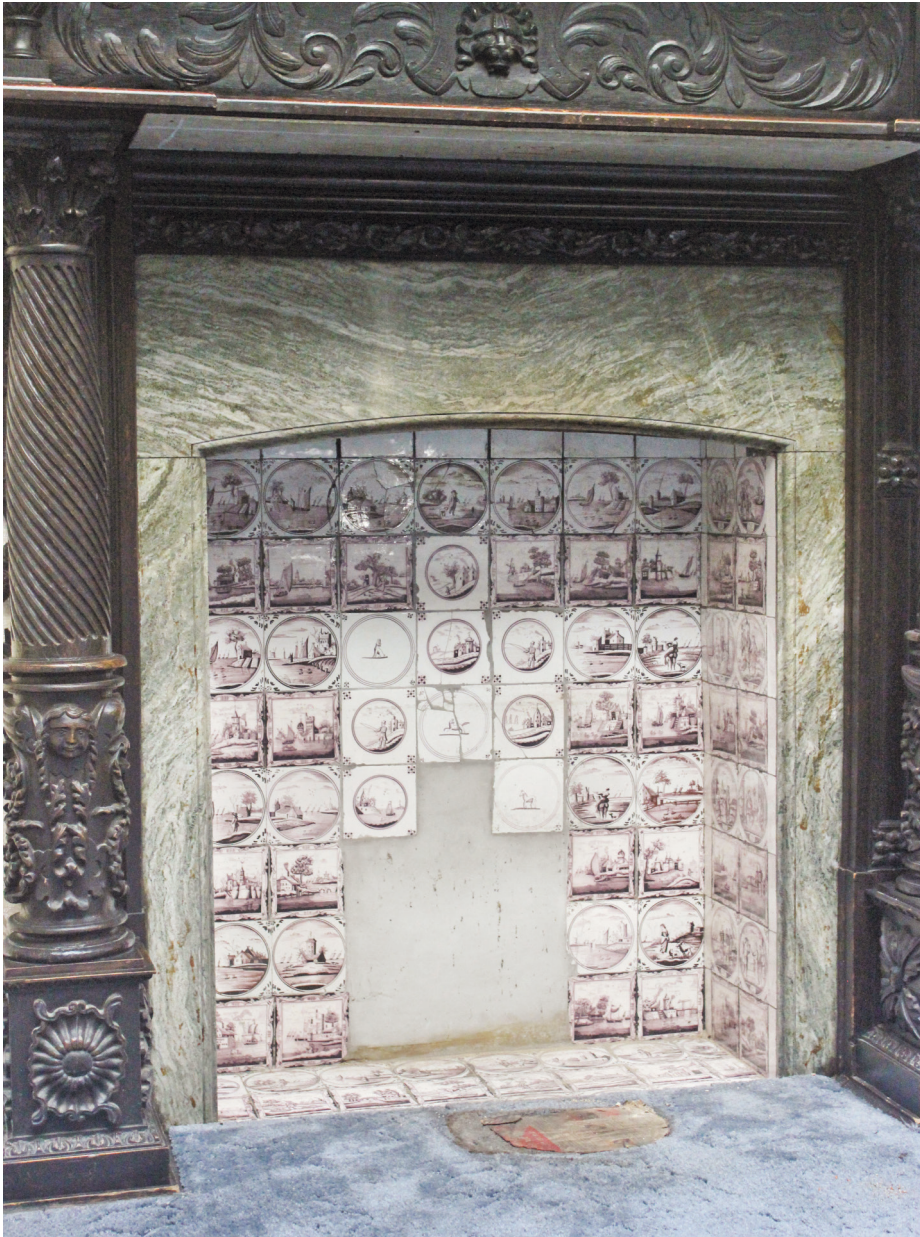
Fig 3 Surrey delftware tiles. Fireplace with late Victorian tiles, Shottermill Hall, Haslemere (I Betts).
