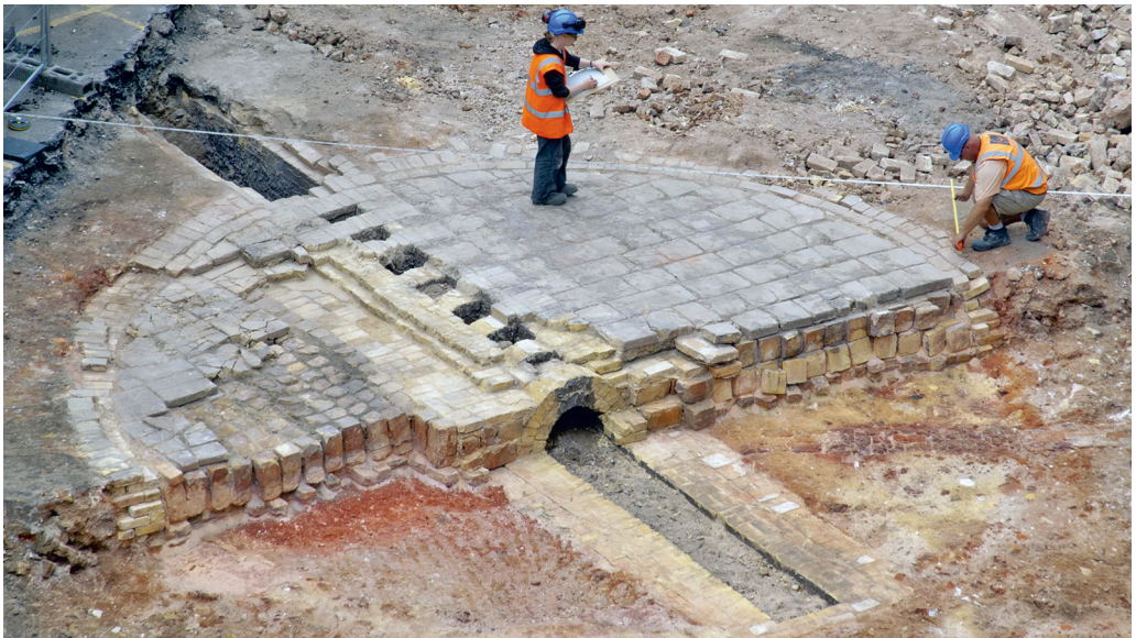
Fig 12 Doulton Terra Cotta Works. View of a section through the eastern kiln (S7), looking south-west.
