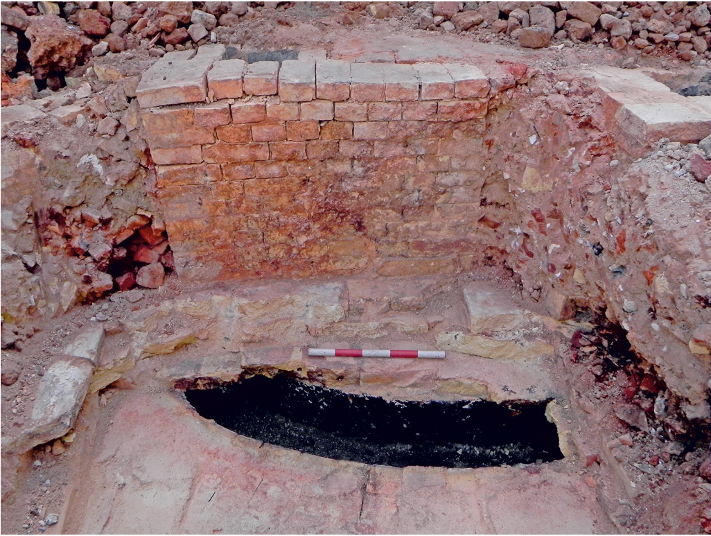
Fig 9 Doulton Terra Cotta Works. View of floor of Structure 5 with one of three flues found below it and one of the three brick structures built on it, looking south (0.5m scale).
