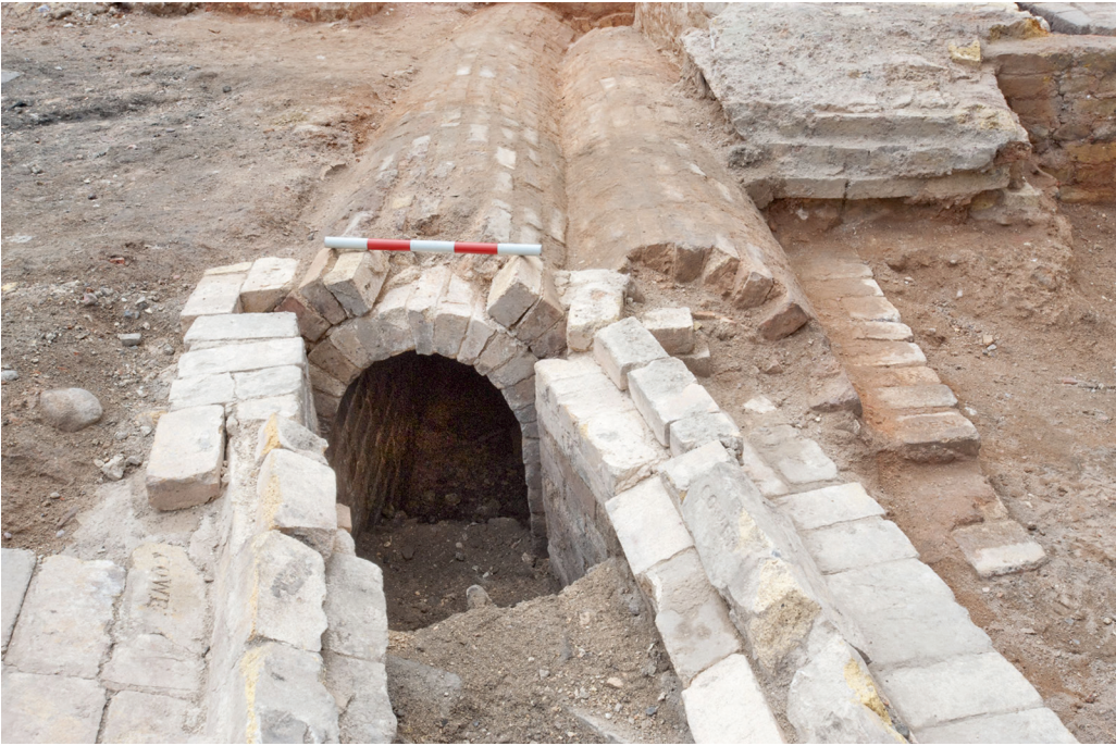
Fig 7 Doulton Terra Cotta Works. View of the double flues (Structure 3) looking south (0.5m scale).
