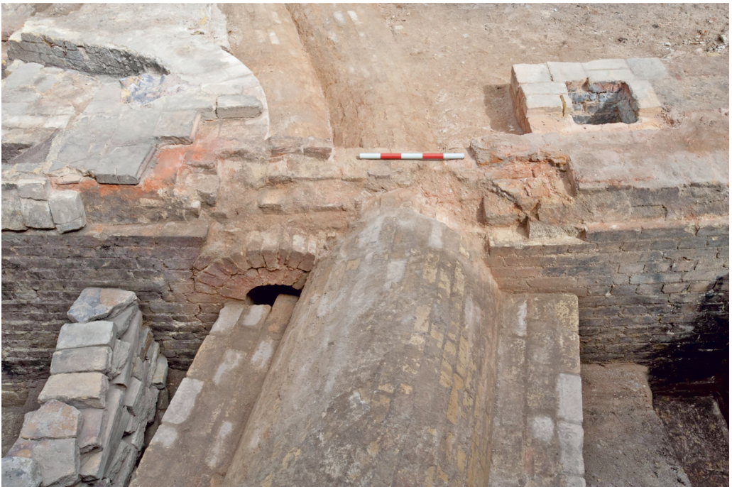
Fig 15 Doulton Terra Cotta Works. View of flue Structure 11 inserted into disused Structure 2 to join a re-used Structure 3 flue to the chimney, looking north (0.5m scale).
