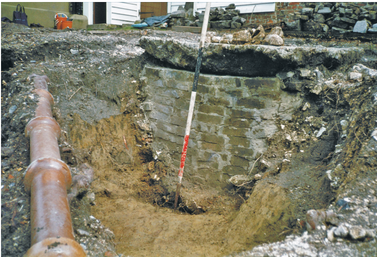
Fig 5 Cheam pottery. Repair to well, looking north (photograph: LBS archives).
