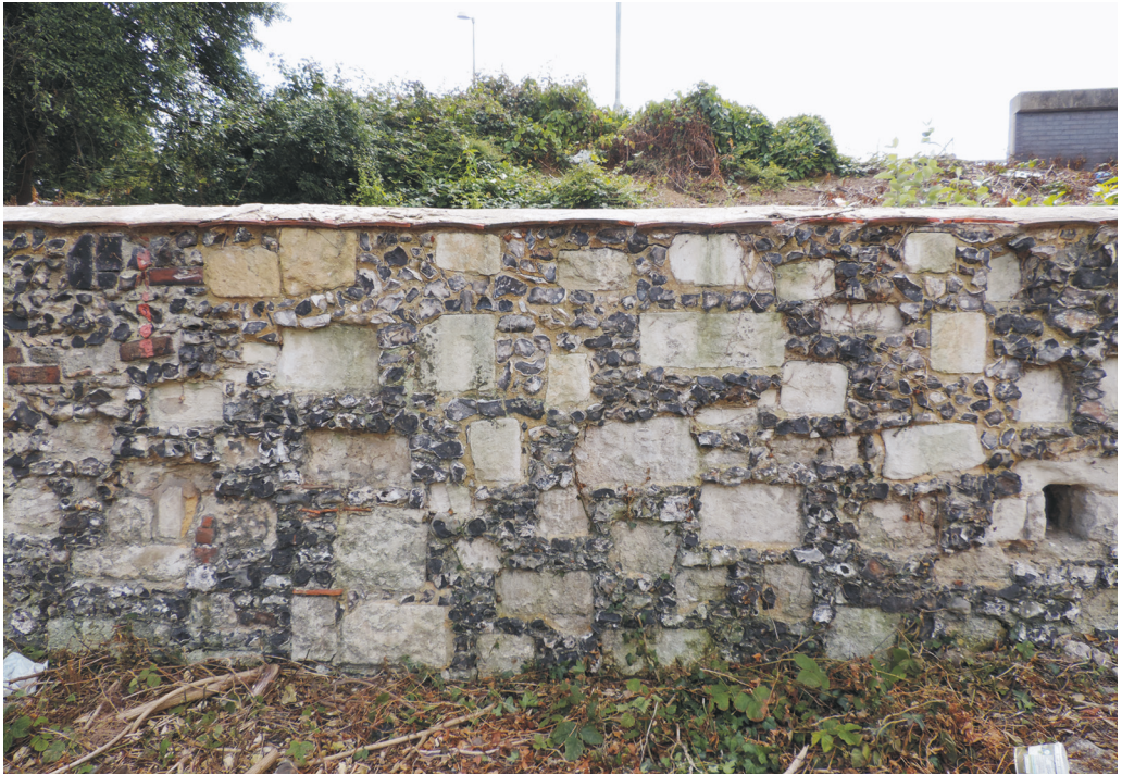
Fig 14 Merton Priory. North-eastern boundary wall composed principally of ashlar blocks and flint, with some brick and tile. (Photograph by MOLA)
