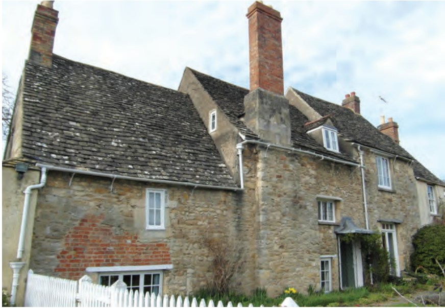
Fig. 4.2. Bartlemas Farmhouse, east-facing frontage.
