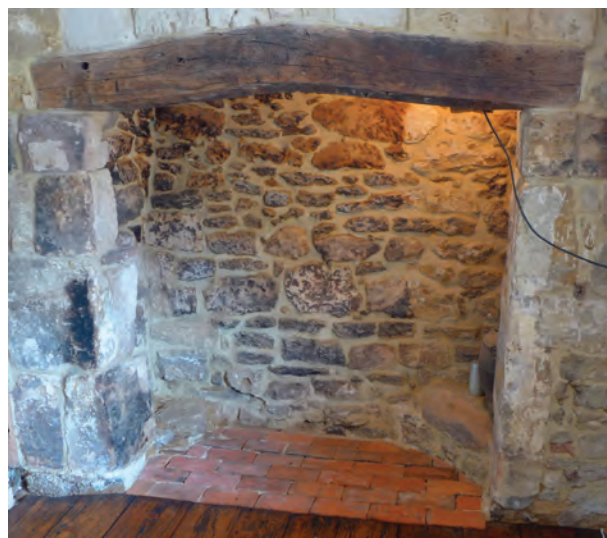
3. The rear wall of this inglenook contains fragments of a chamfered lintel and socketed stones.
