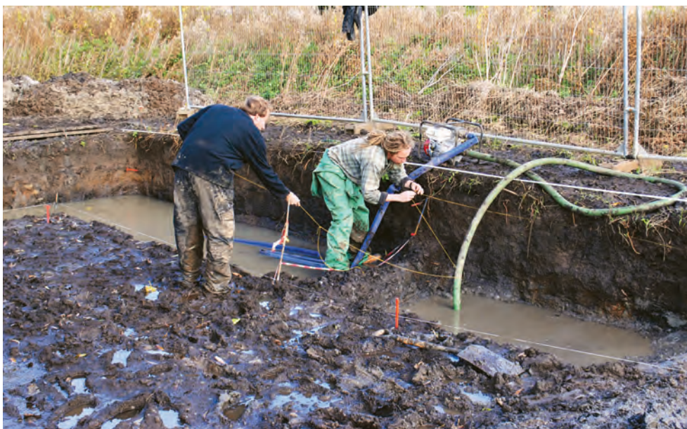
Fig. 5.8. Excavation conditions in Trench 1.
