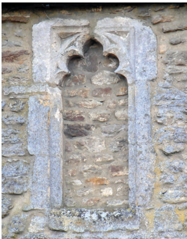
Fig. 5.31. Blocked-up dormitory cinquefoil window, priory building, eastern façade.
