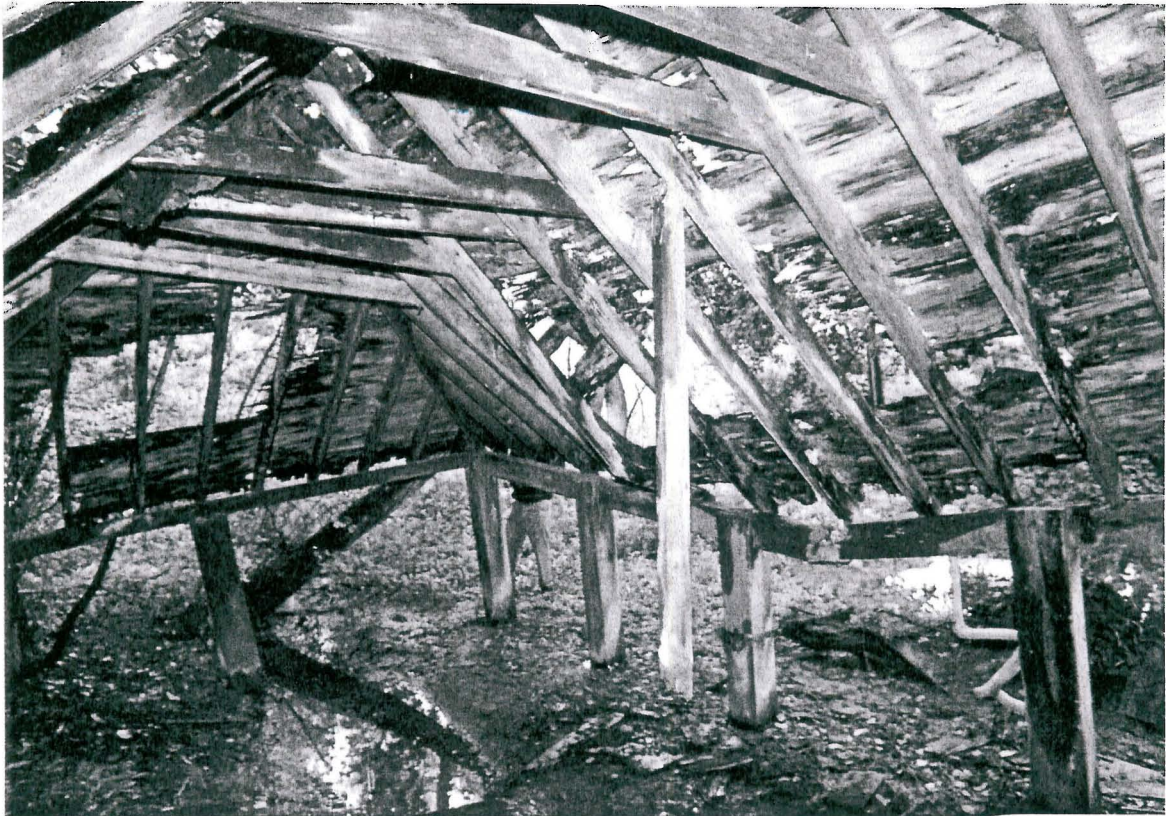
The interior of the boathouse from the south-east
