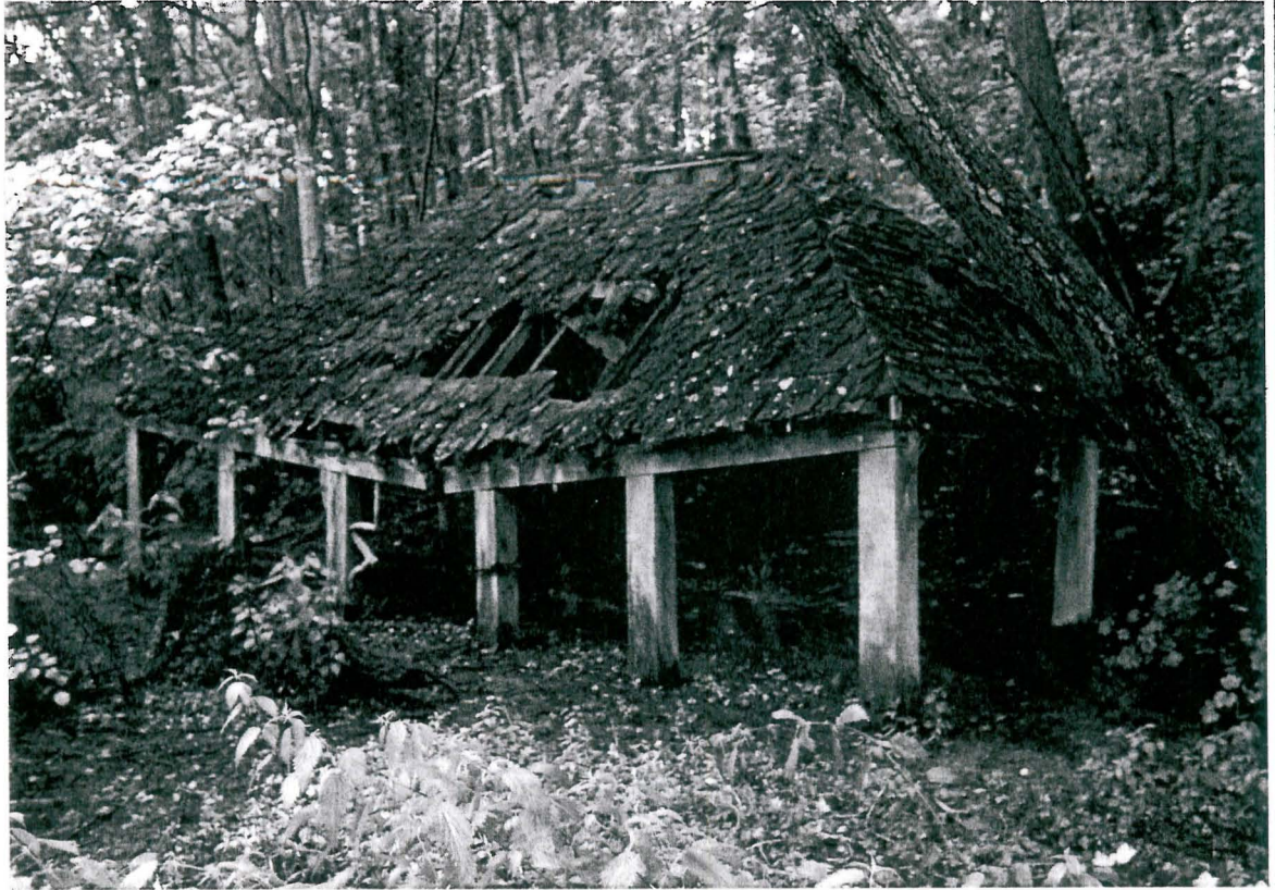
The boathouse from the north-west
