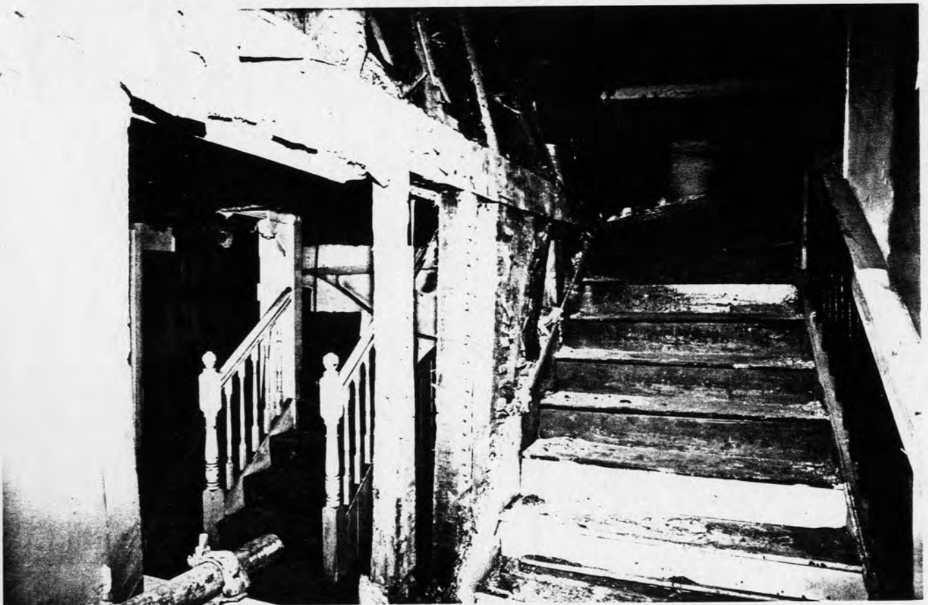
Buildings A & C: The party wall from the south-east, showing the wall plate of A and the raised wall of C
