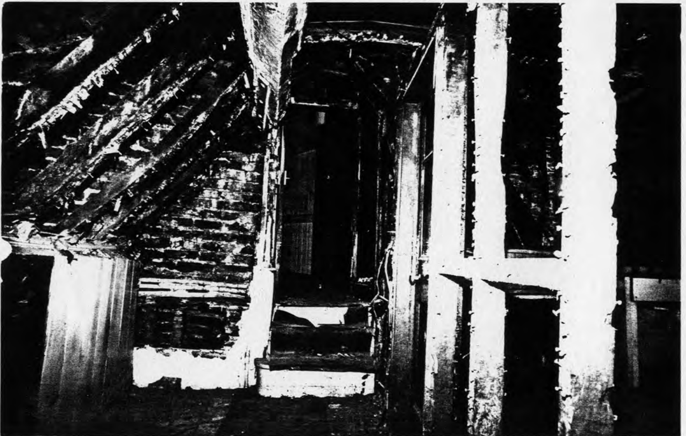
Building A: South frame, attic floor, north face, showing the inserted doorway and part of the original roof
