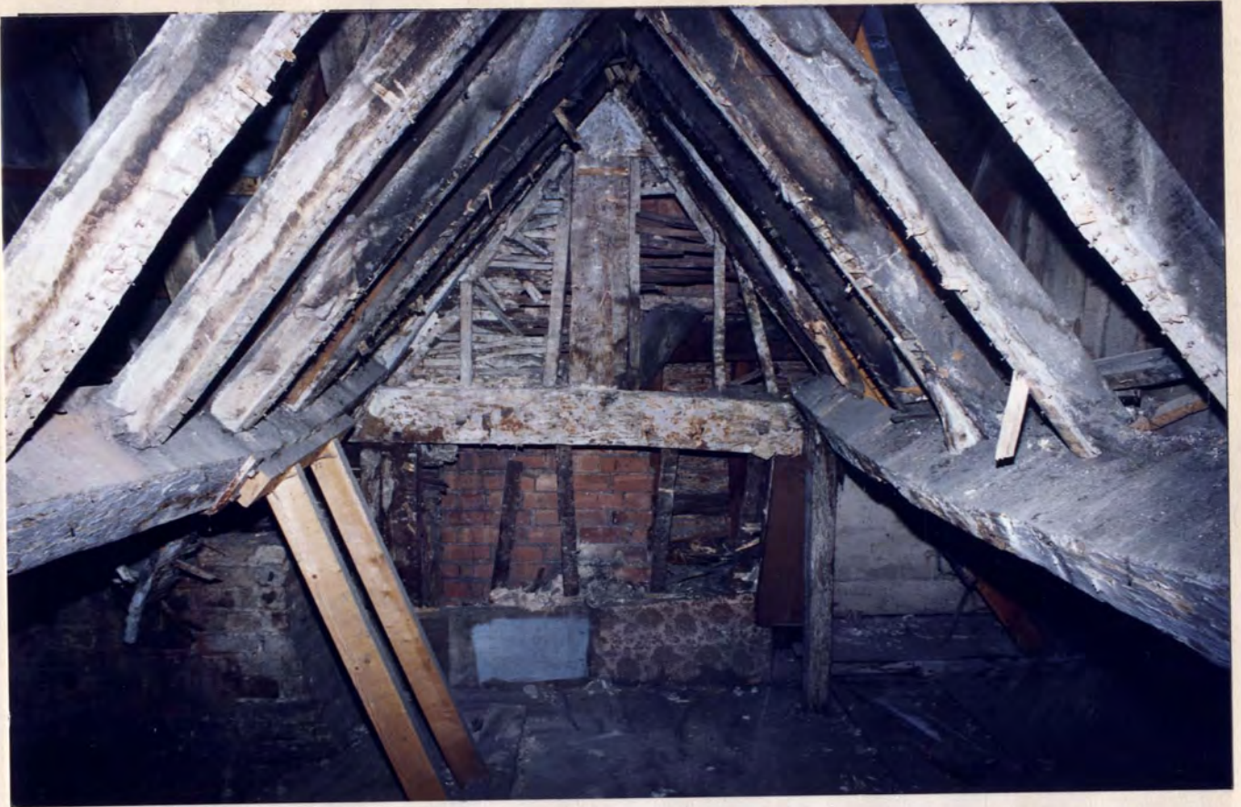
Building A: North frame, attic, south face, showing the upper part of the truss and original purlins and rafters
