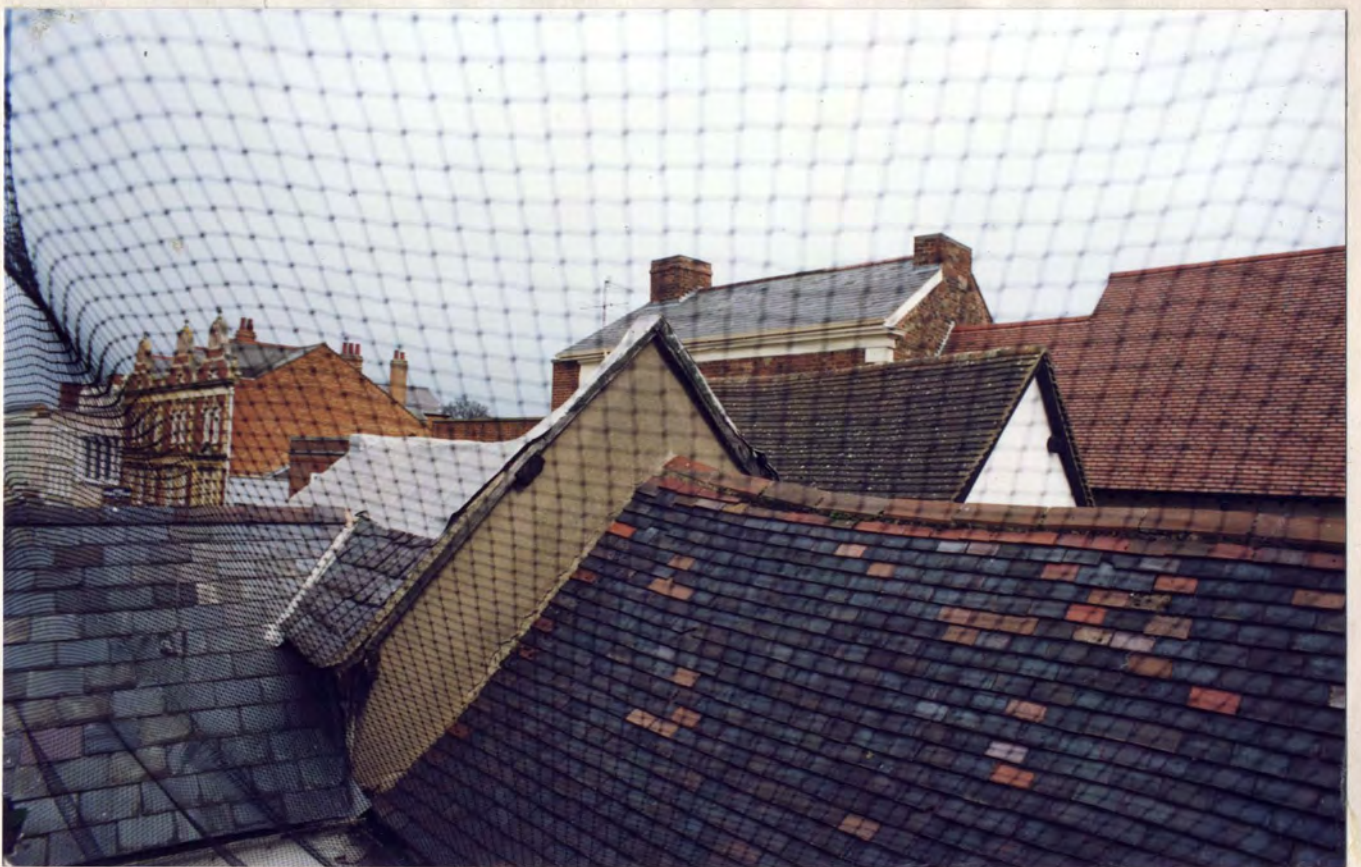
The roof of 12 High Street from the south-west
