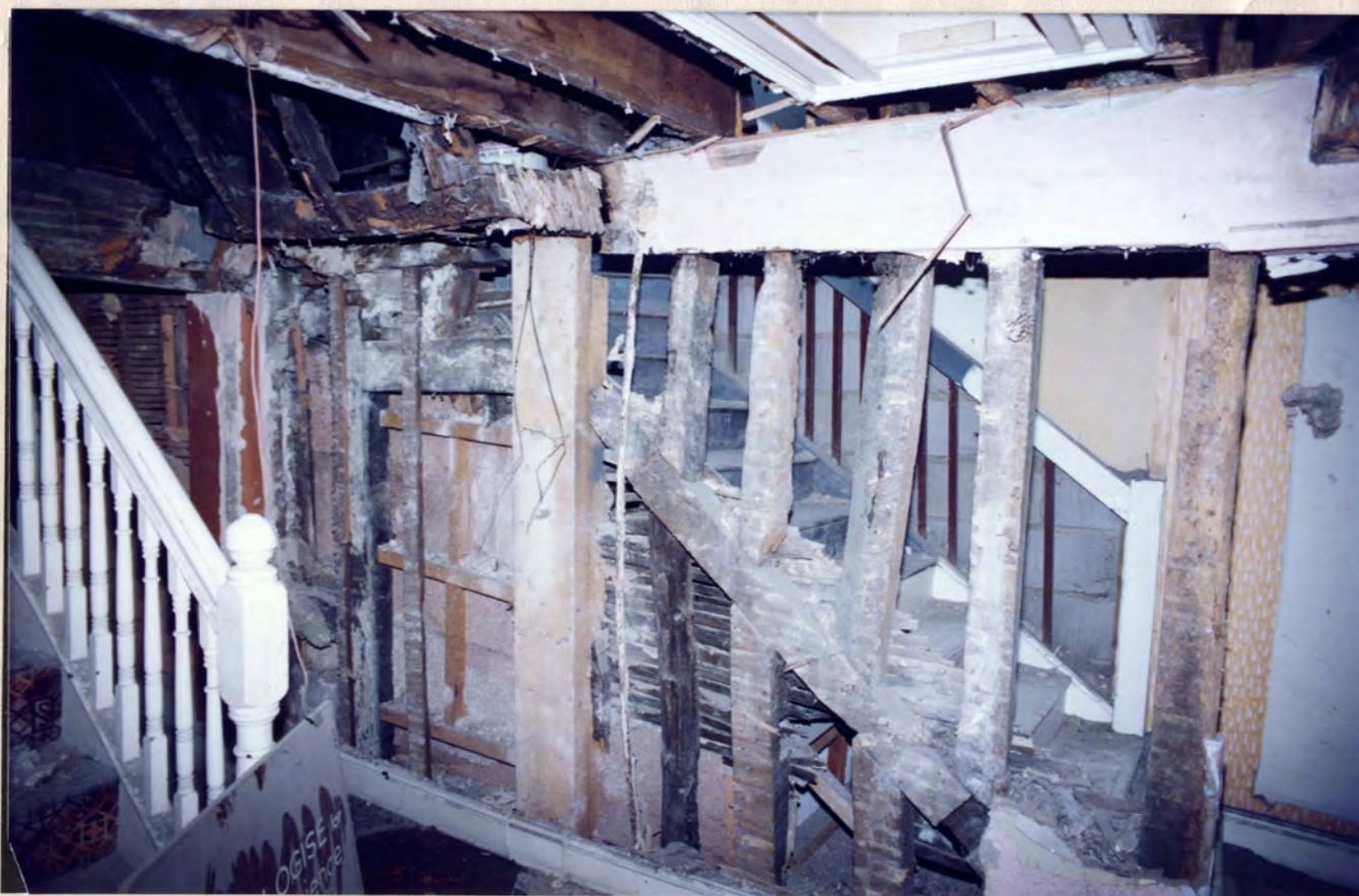
Building A: East frame, 1st floor, west face, showing the north-eastern corner post and the wall plate
