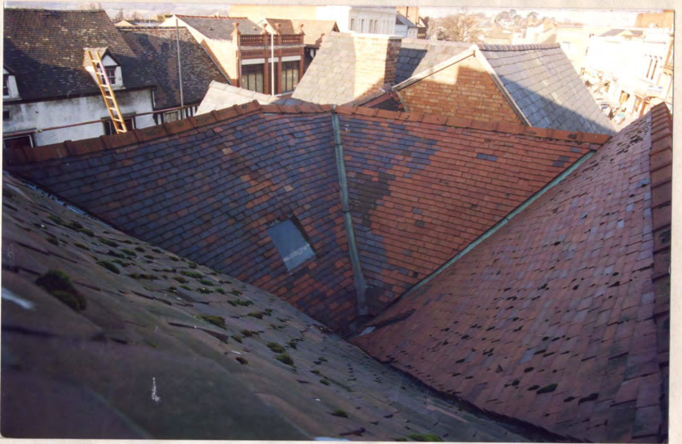
The roof of building A from the south
