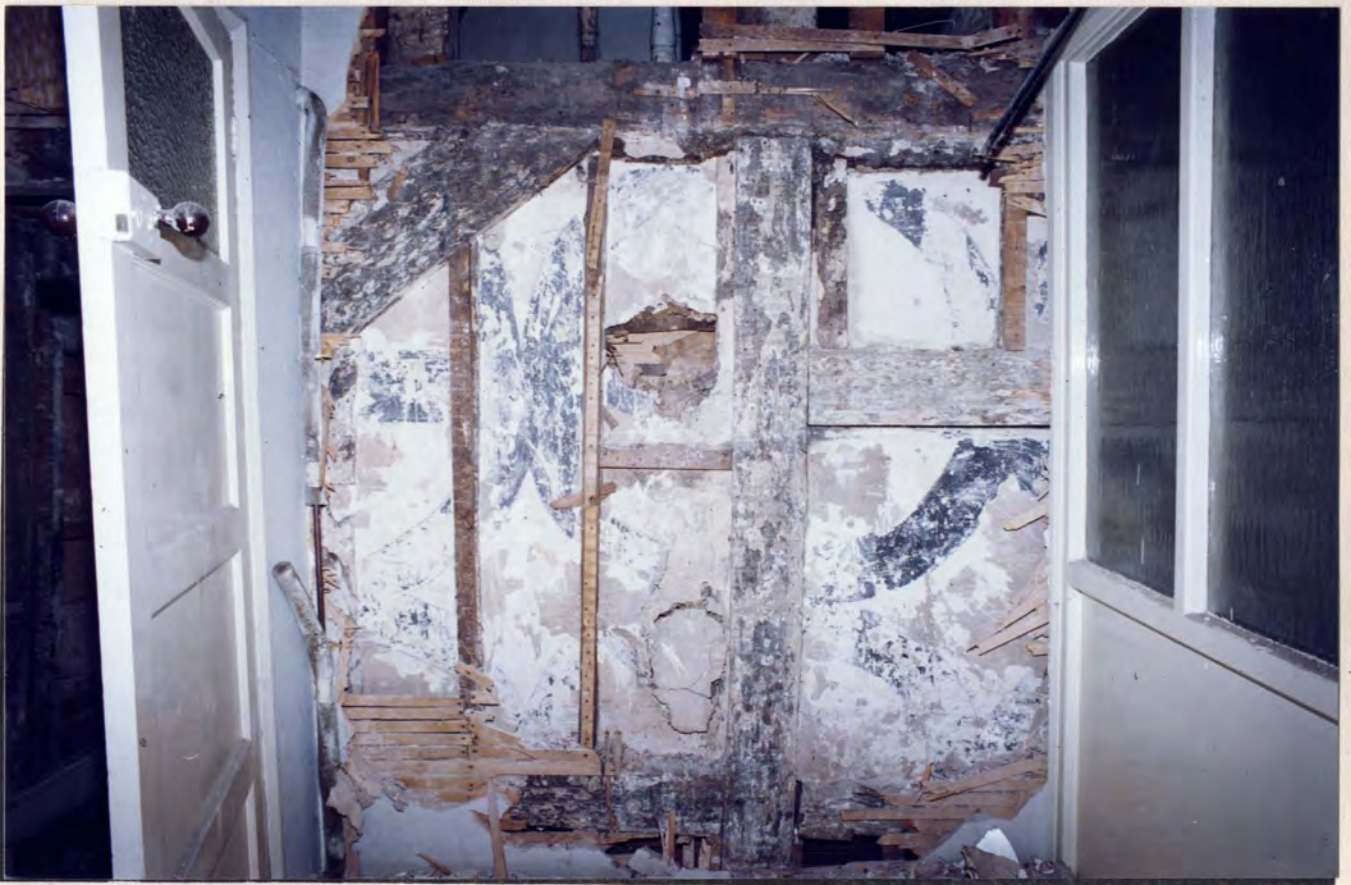
Building A: Intermediate frame, attic floor, south face, showing original purlins and rafters
