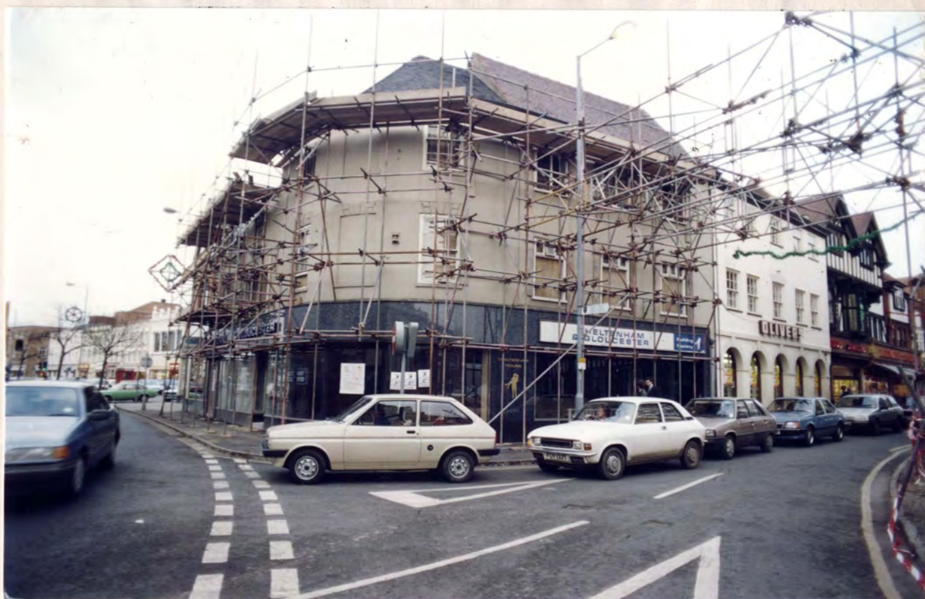
1 Bridge Street from the south-west
