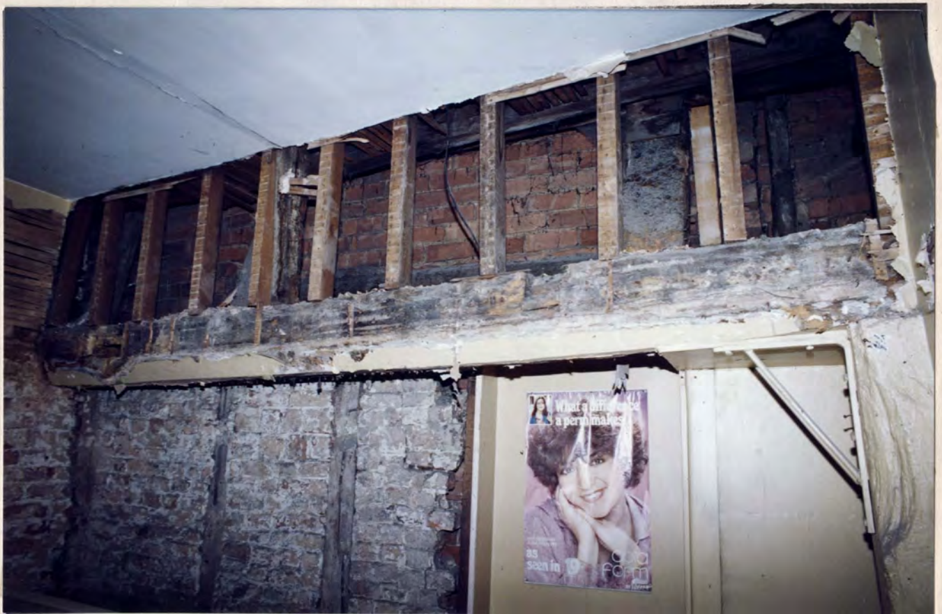
Building A: North frame, attic, south face, showing the upper part of the truss and original purlins and rafters
