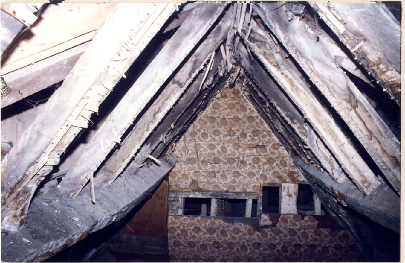
Building A: Intermediate frame, attic floor, south face, showing original purlins and rafters
