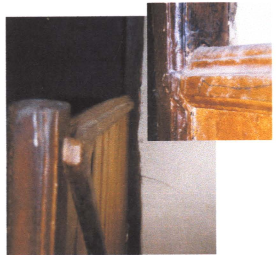
Plate 4 Balustrade and moulded Handrail.
