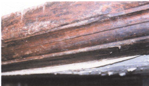
Plate 5 Detail of moulding from window frame in dormer window
