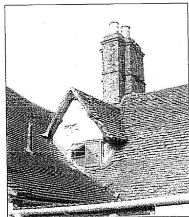
View illustrating Roof Line intersections and modified dormer window
