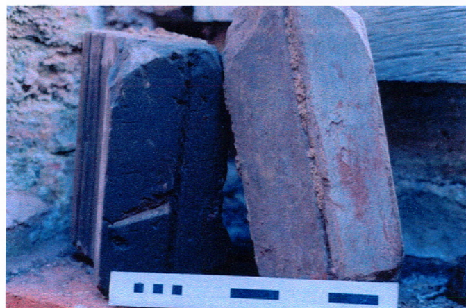
Plate 9, 17th c. Transom/mullion pieces from Room 4, Small Finds 3 and 4, showing glazing slots and paint.
