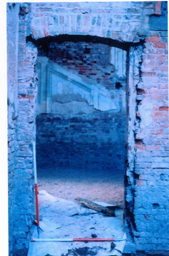
Plate 15, Doorway between Room 1 and the stair tower, unblocked.
