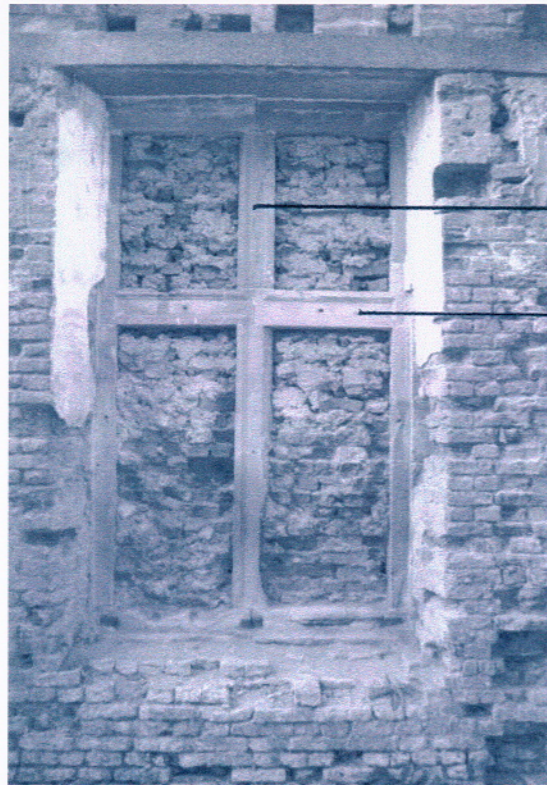
Plate 5, Blocked 17th century window in the main entrance hall.
