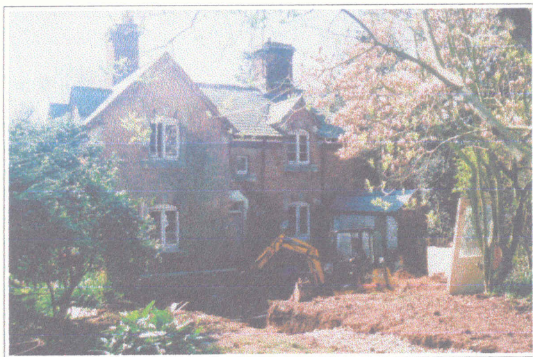
Plate 4 Showing area of excavation for foundations
