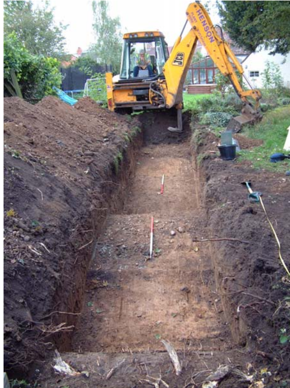
Plate 1: The trench during excavation
