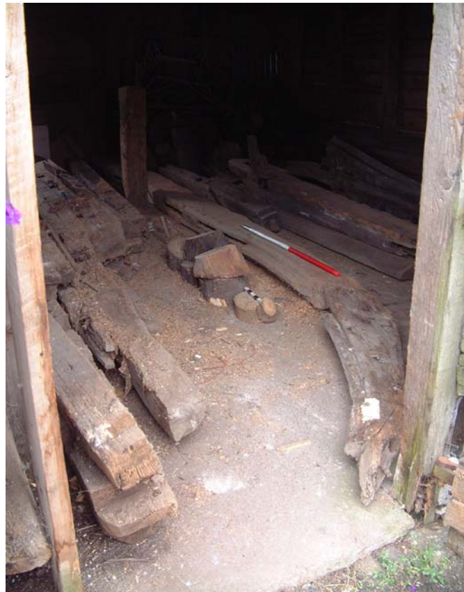
Plate 2: The remaining cruck blade is unfortunately fractured (Scale 1 metre)
