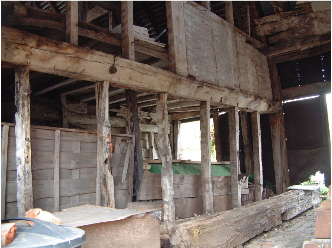
Plate 15: The inserted 'passage frame' in Bay 1, looking north-west
