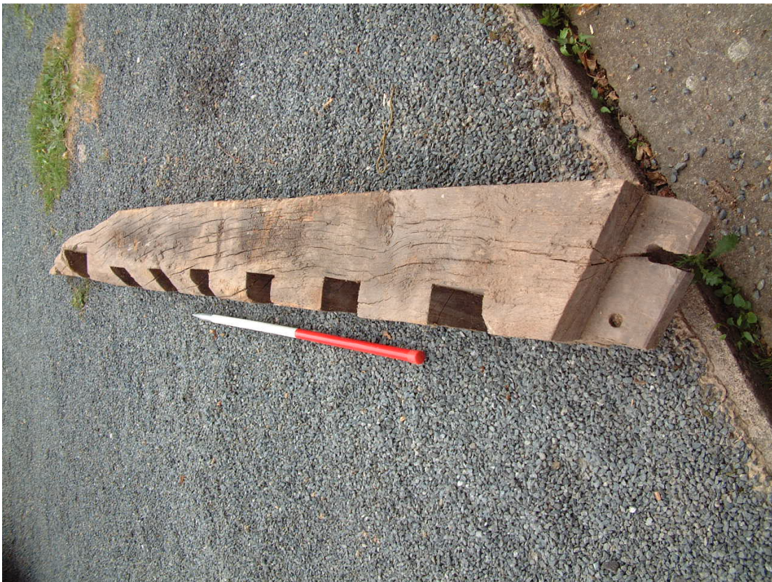
Plate 8: Upper floor beam. Angle of tenon suggests it was an integral cruck tiebeam (Scale 1 metre)
