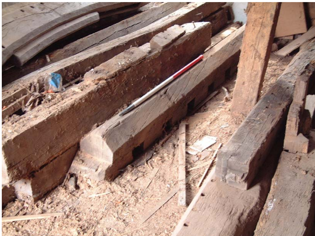
Plate 10: Steep chamfered bridging beam (Scale 1 metre)
