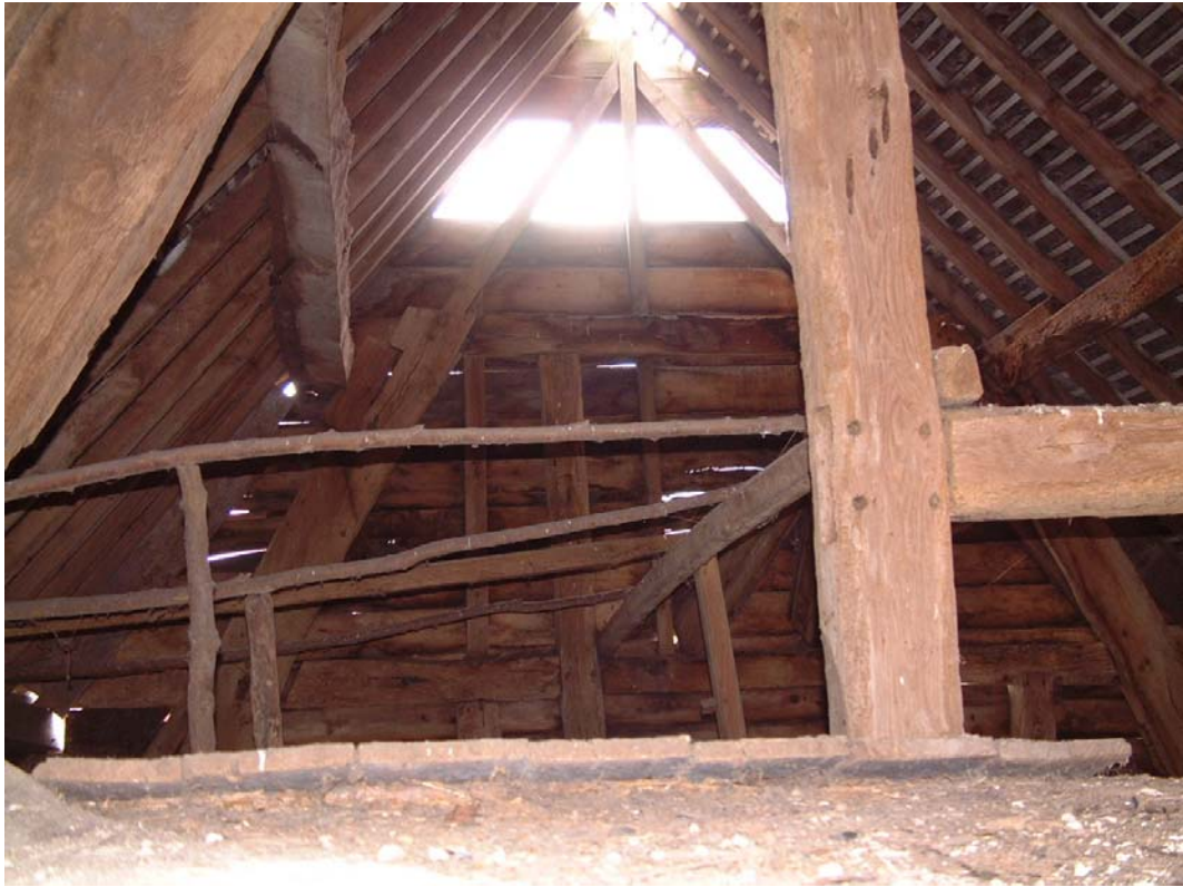
Plate 19: Base cruck C4, looking west
