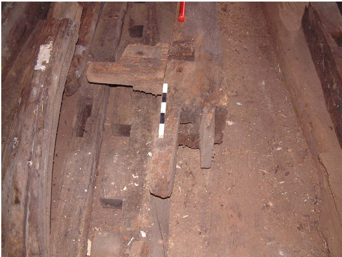
Plate 6: Cruck stud with attached crook spur, the opposite one was not found (Scale 25 centimetres)
