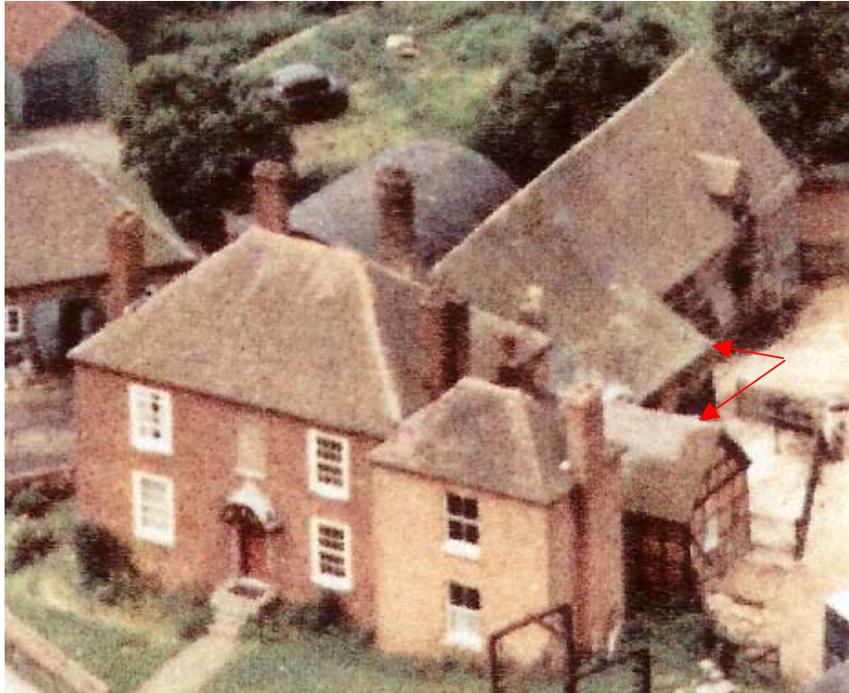
Plate 11: Aerial photograph of Butts Bank Farm showing the northern timber frame projection (arrowed), probably of 17 th century date (Photograph courtesy of Mr and Mrs Barnes)
