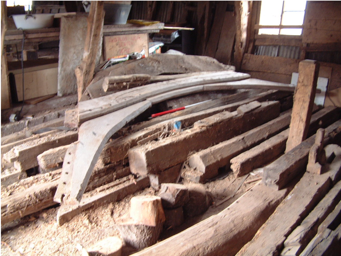
Plate 3: Cruck collar re-united with its arch-braces (Scale 1 metre)
