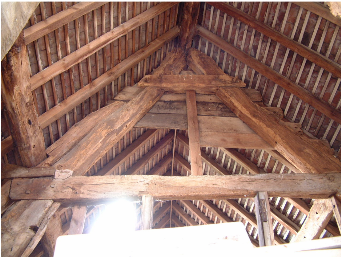
Plate 16: Detail of the true cruck apex style
