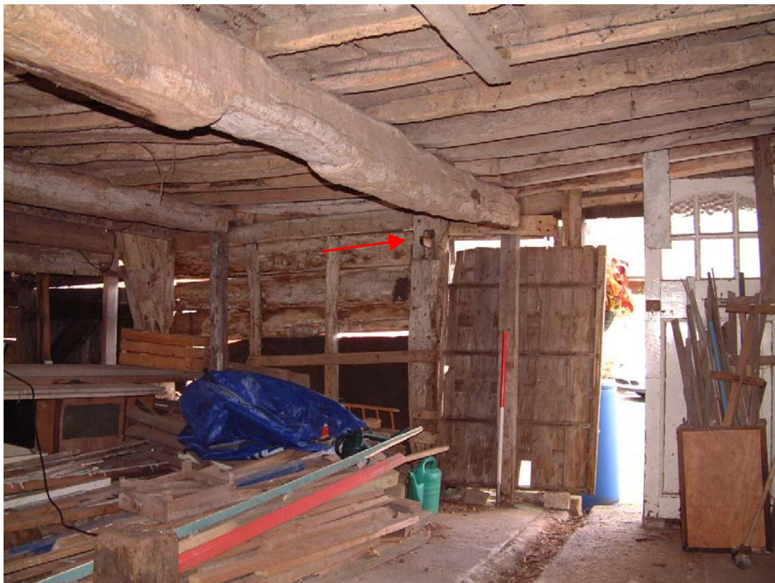
Plate 18: The opposite northern framing of Bay 2, with the original location of the opposite end of the bridging beam arrowed
