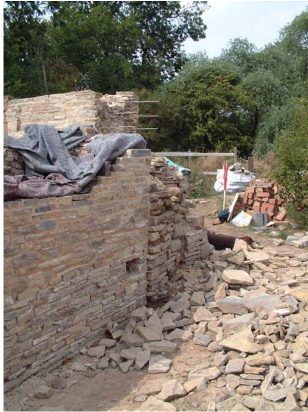
North-east corner of kitchen looking north-west
