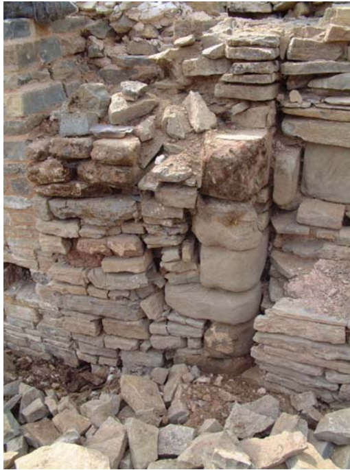
Plate 6: Western reveal of doorway in east-west wall, exposed during renovation work
