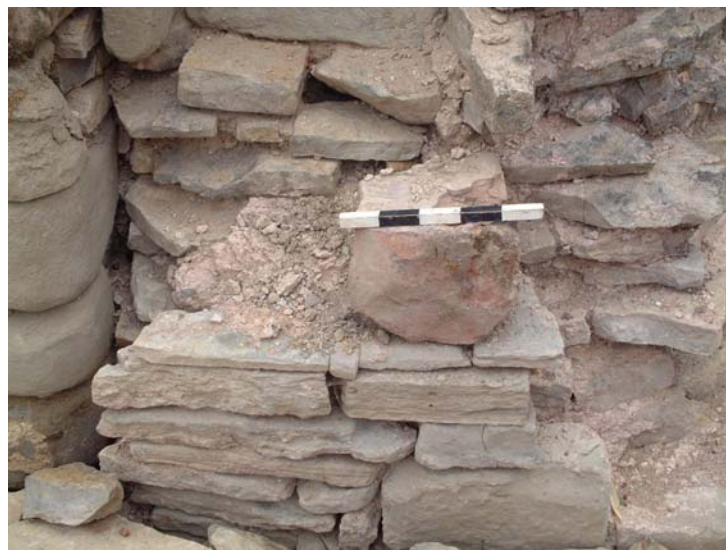
Plate 7: Burnt stone re-used in repair to north-eastern corner. The stonework below is the face of the Phase 4 repair to the wall
