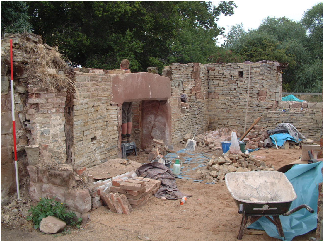
Internal western elevation looking north-west (scale 2 metres)
