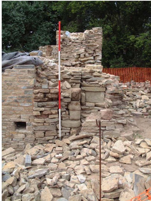
North-east corner looking west (scale 2 metres)
