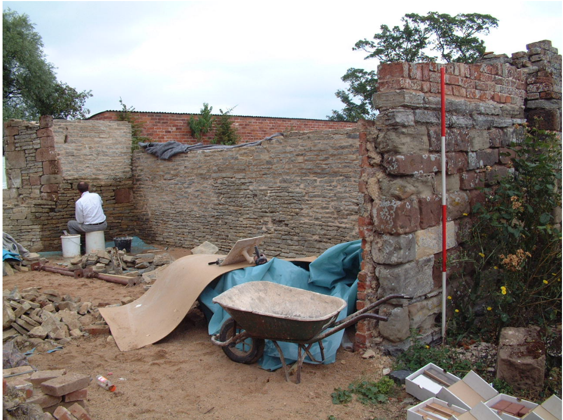
Internal north-east corner (left of centre) looking north-east
