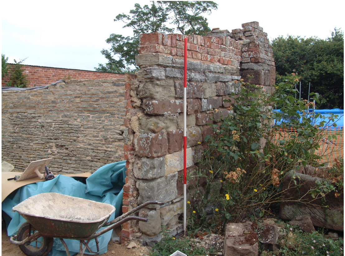
Ashlar blockwork of the southern elevation, looking north-east (scale 2 metres)
