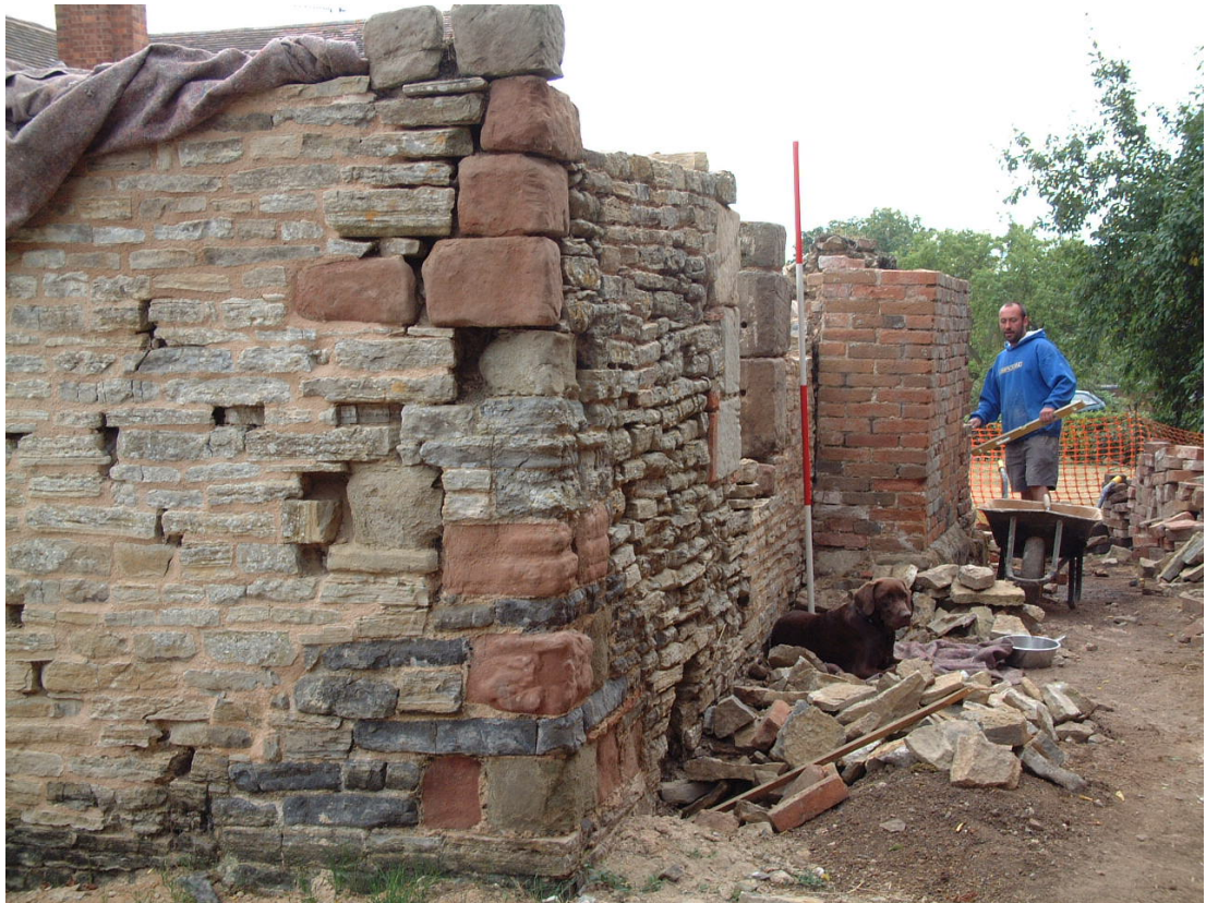
North-western corner looking south (scale 2 metres)
