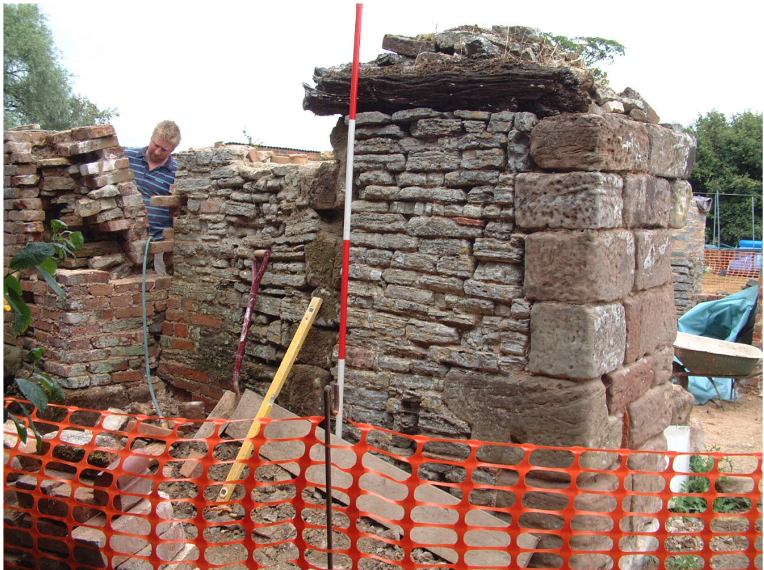
The south-west corner looking north-east (scale 2 metres)
