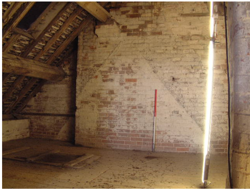
Roofline of the earlier phase of the mill on the gable end of the farmhouse (scale 1 metre)
