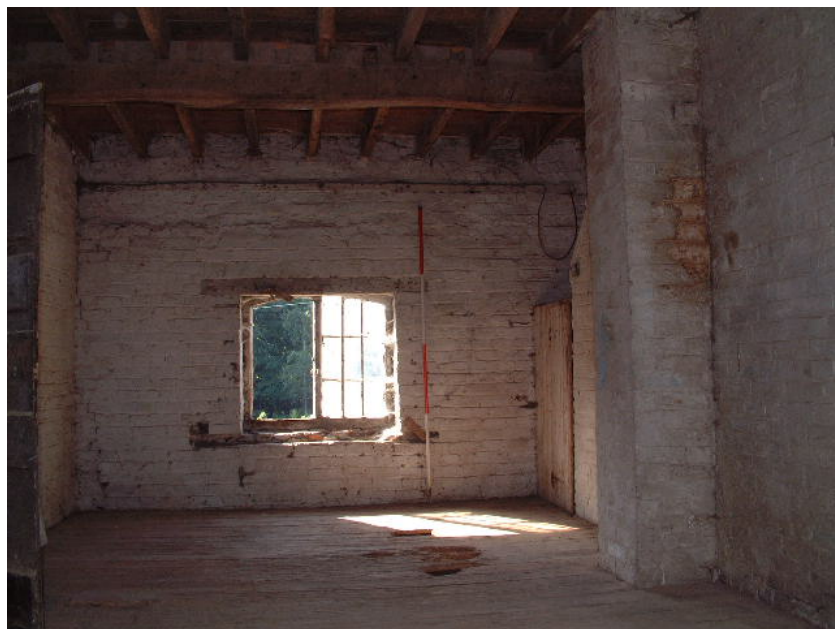
Western end bay of floor 1 (scale 2 metres)
