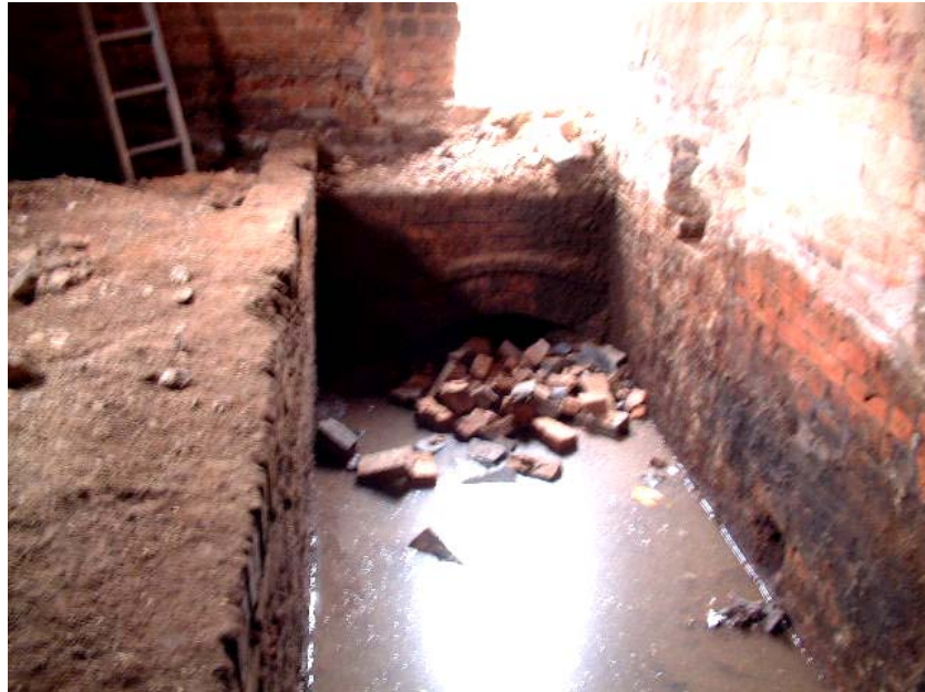
The partially excavated wheel chamber looking south towards the drain
