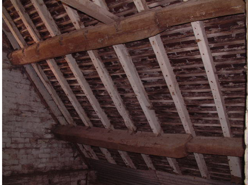
Re-used purlins, note the reduced timber at the ends
