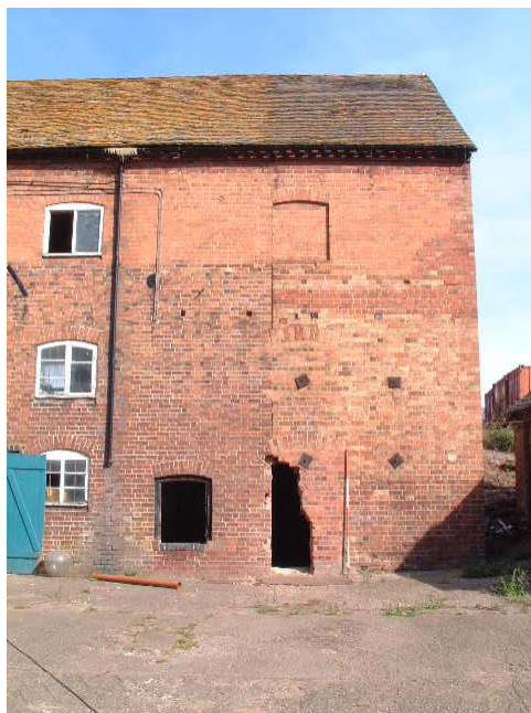
The low aperture marking the position of the pit-wheel, the waterwheel sat in the end bay behind the 2-metre scale
