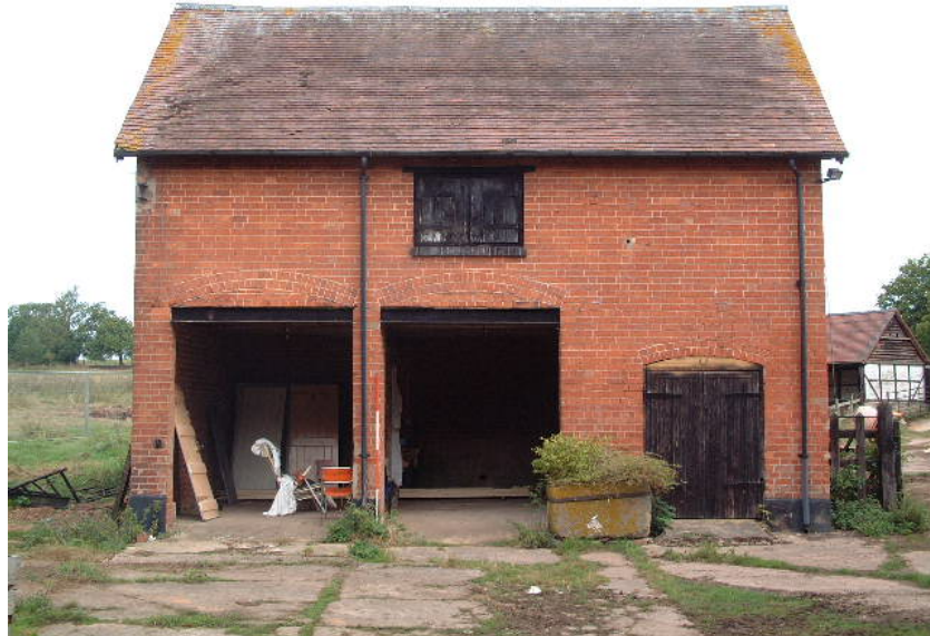
Building 4B looking north-east (scale 2 metres)
