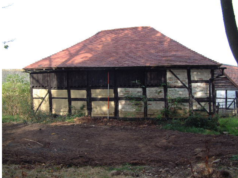
Building 2 looking north-west (scale 2 metres)
