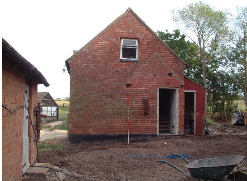
Building 3 looking north-east (scale 2 metres)
