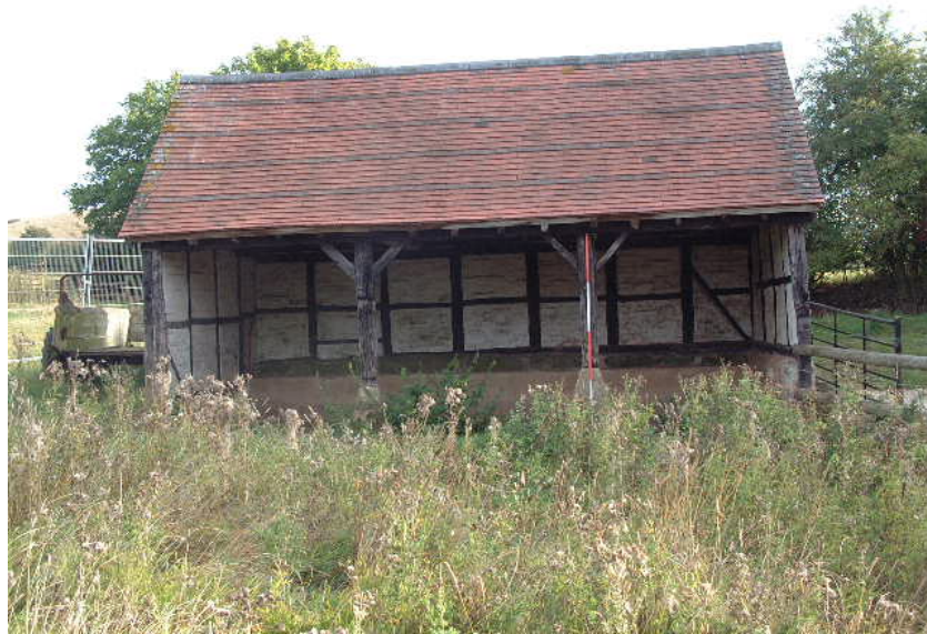
The shelter shed (Building 1) looking east (scale 2 metres)
