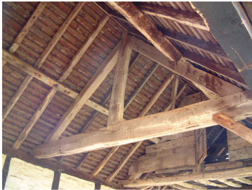
Re-used timber as tiebeam in kingpost truss (Building 1)
