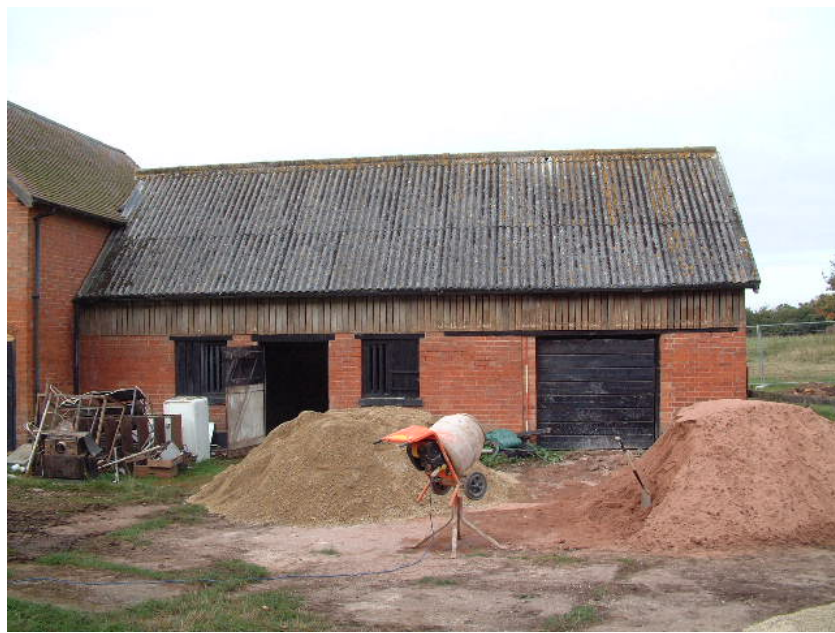
Building 4A looking north-west (scale 2 metres). Space 4B is at right angles to it on the left of the picture
