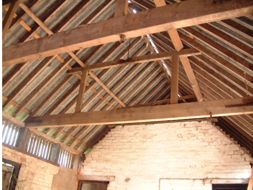
20 th century roof trusses in Building 4A
