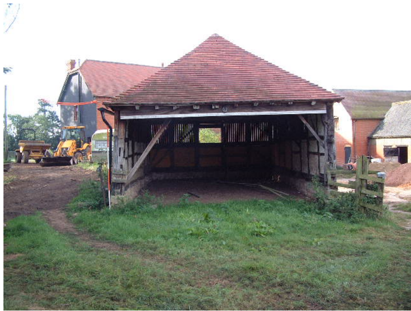
Building 2 looking south-west (scale 2 metres)
