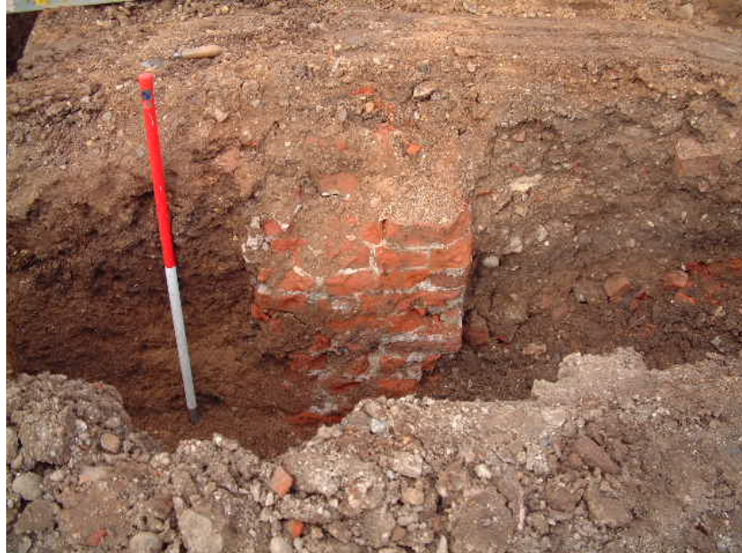
Wall foundations [105] looking west (scale 1 metre). Note the cellar backfill to the right and none to the left
