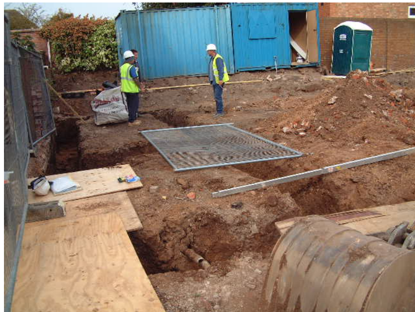
Work in progress at Head Street
