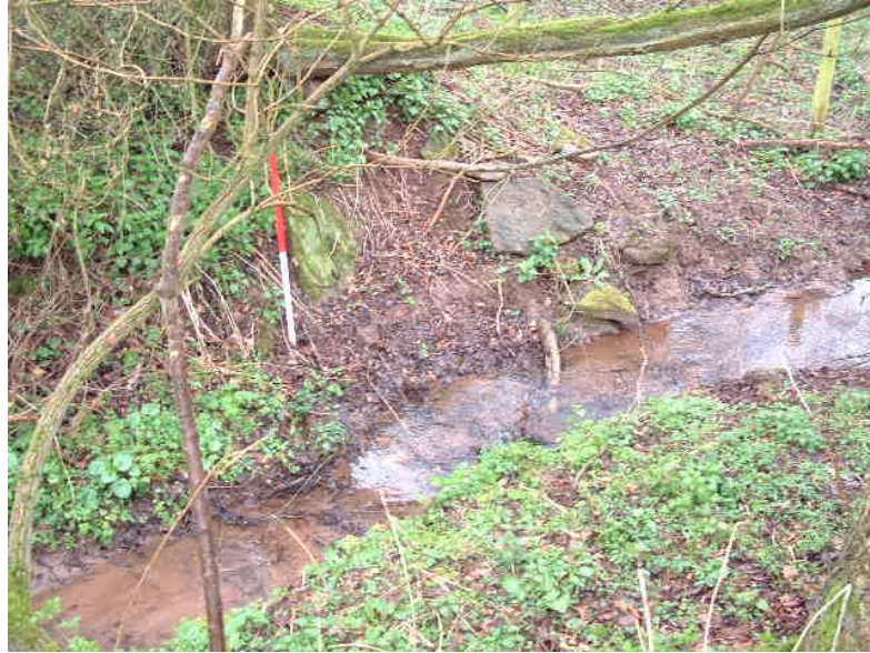
Stone slabs scattered along the stream and in the bank may be from the former footbridge or possibly artificial rapids at the head of the waterfall below the present footbridge (Looking west; Scale 1 metre)
