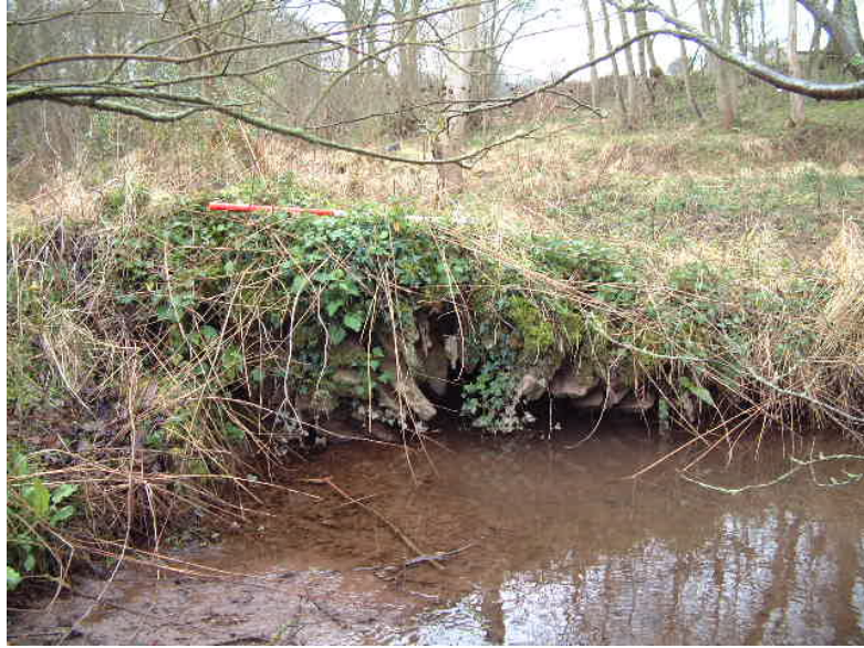
The flat arch of the dry-stone bridge (Looking south; Scale 1 metre)
