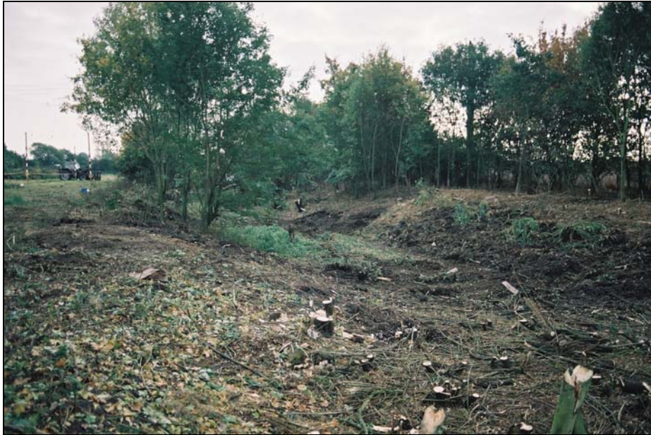
The western end of the site prior to the commencement of excavation work
