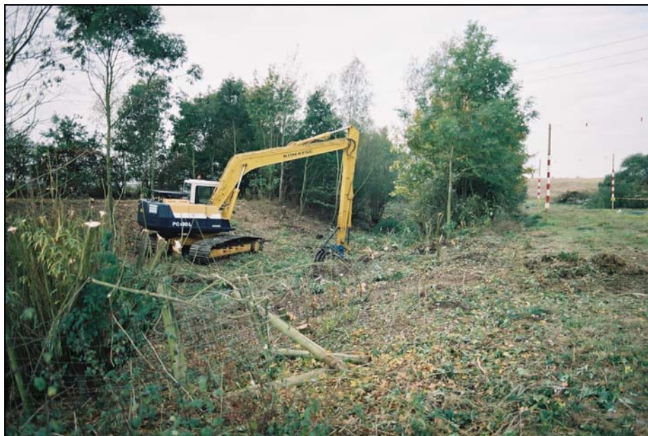
Work in progress, view to the west
