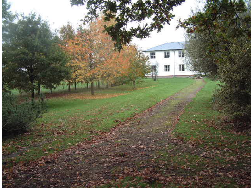
View of the site looking east towards the new extension
