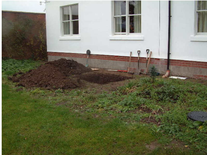
Test Pits 1-4 on the west side of the new build
