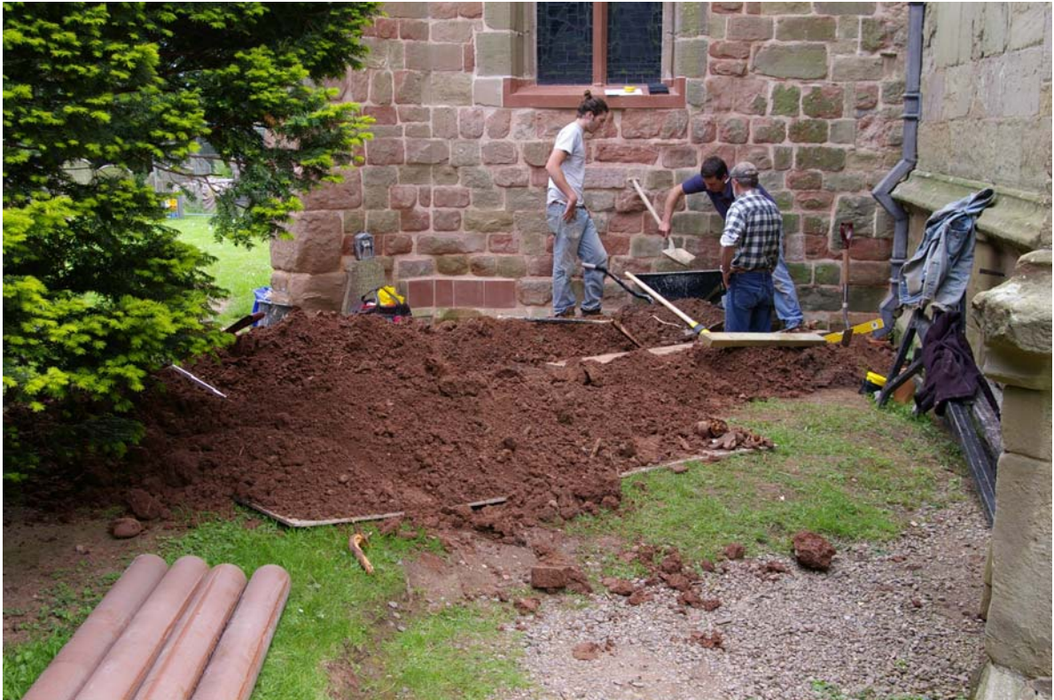
Plate 1: The connecting trench under excavation, looking east.
