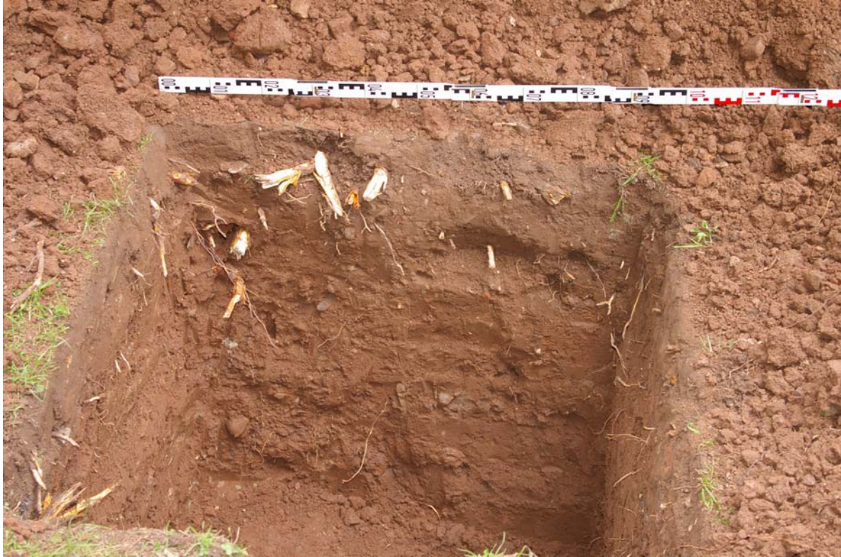
Plate 2: The excavated soakaway pit
