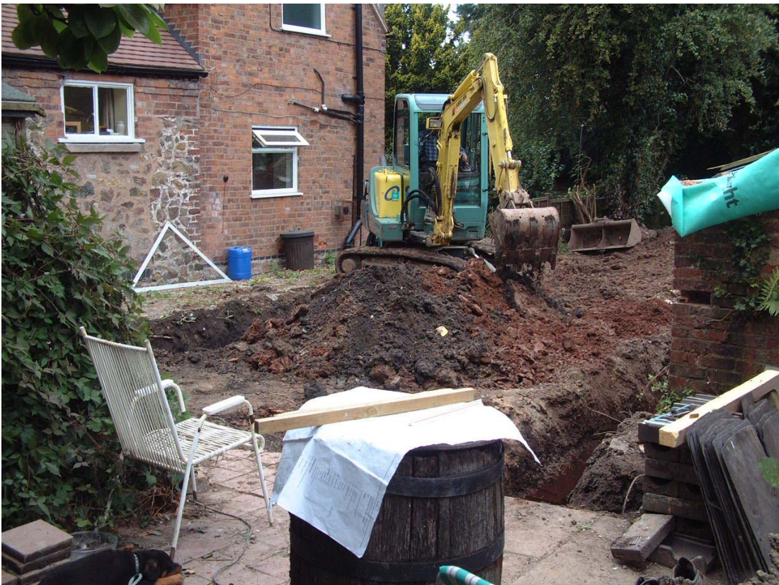
Plate 2: Work in progress at the site
