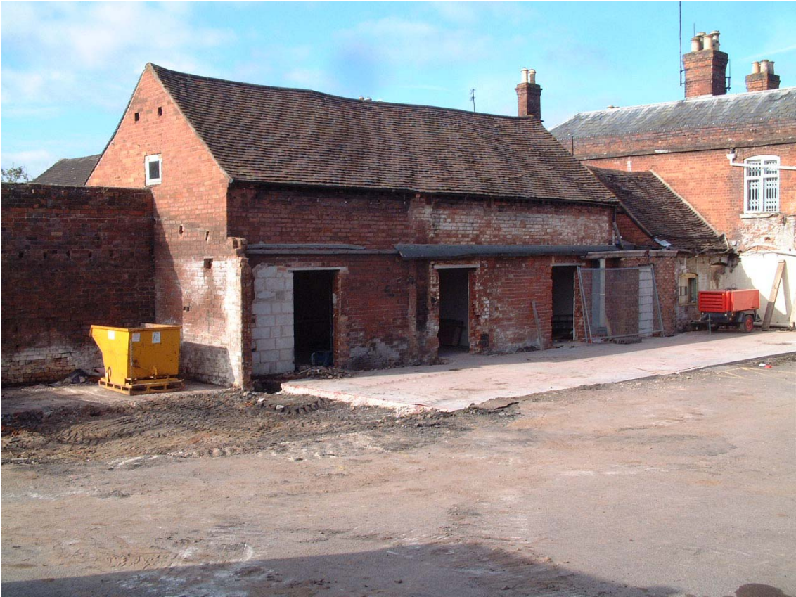
PLATE 4: The site after demolition of the 1960's buildings
