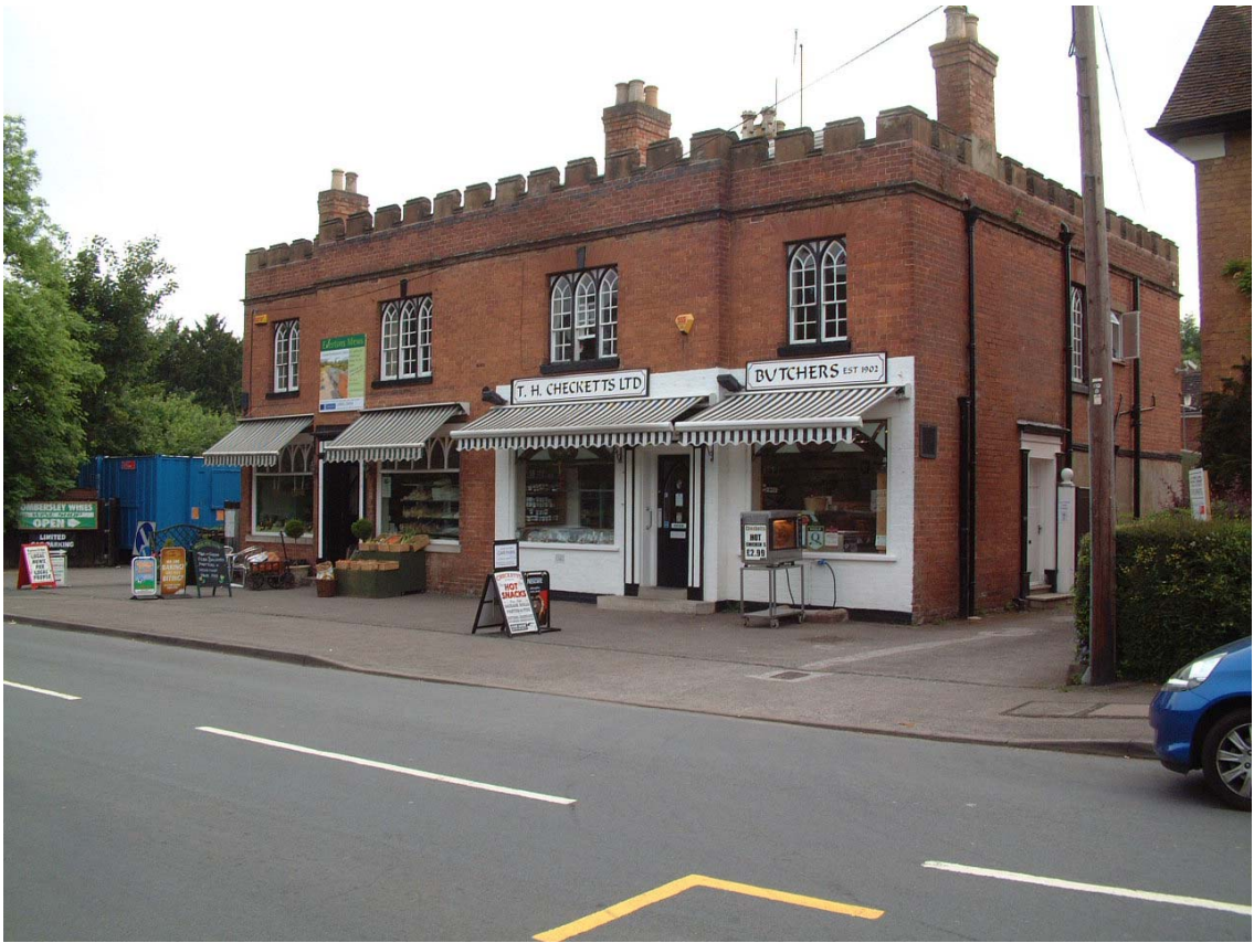
Plate 1: Everton's Store looking north-east from Main Street
