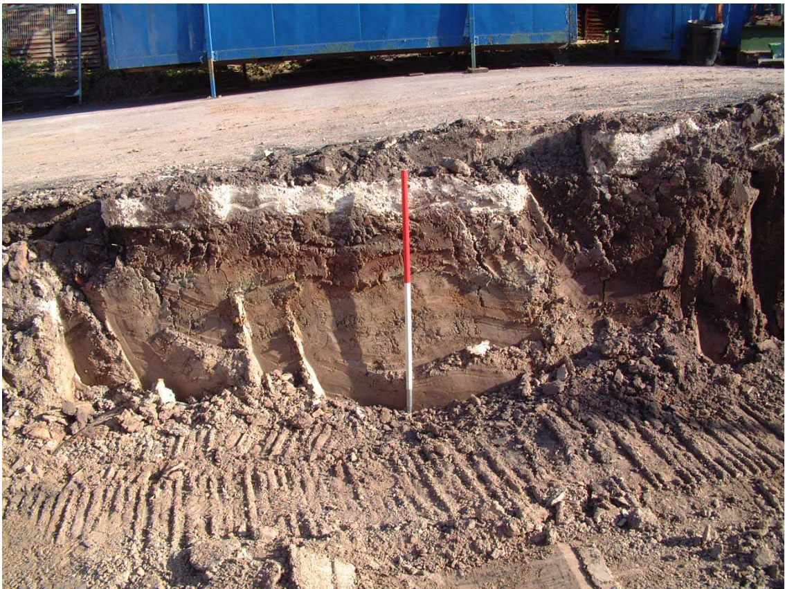
PLATE 6: The general soil / deposit profile on the eastern side of the site (scale 1-metre)
