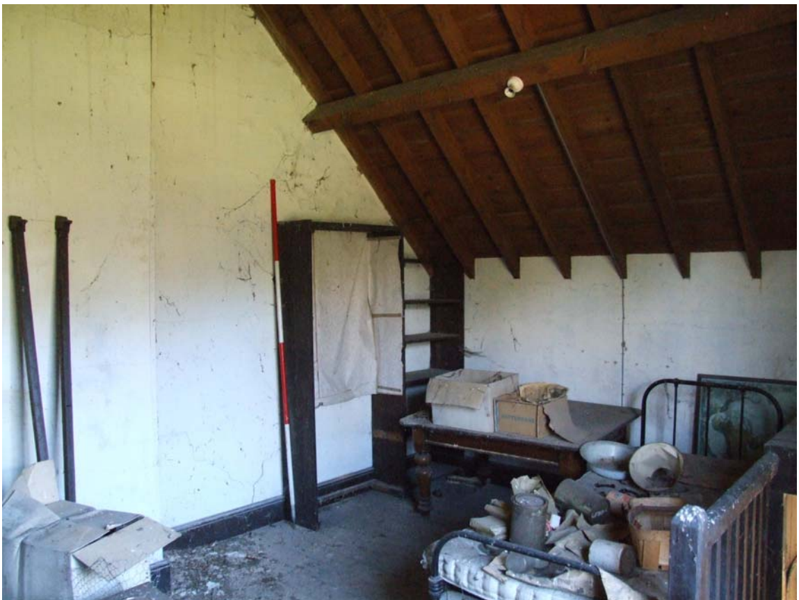
Plate 28: Bedroom above the kitchen in the Jubilee Rooms
