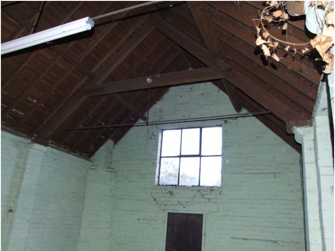
Plate 27: Roof truss in the assembly room
