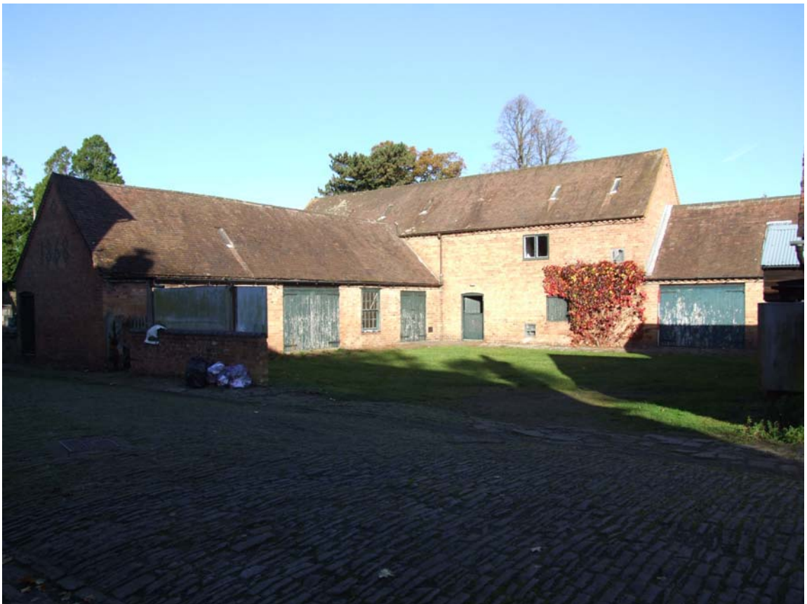
Plate 2: The northern range (right of picture) looking north-west
