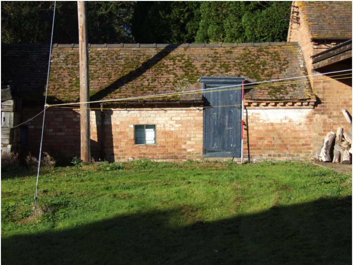
Plate 19: Former piggy in the western range
