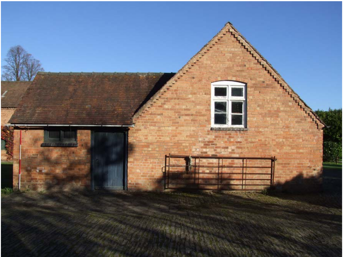
Plate 14: Extension to the eastern range (left of gable)
