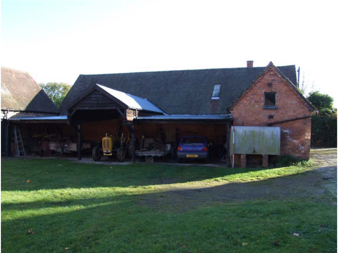
Plate 13: Lean-to on the western side of the eastern range
