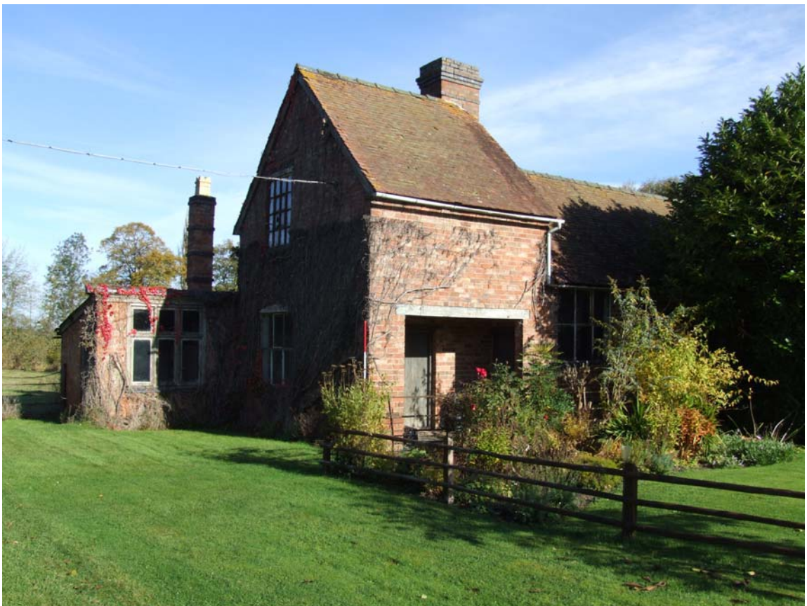
Plate 24: The kitchen and bedroom block of the Jubilee Rooms, looking north-east
