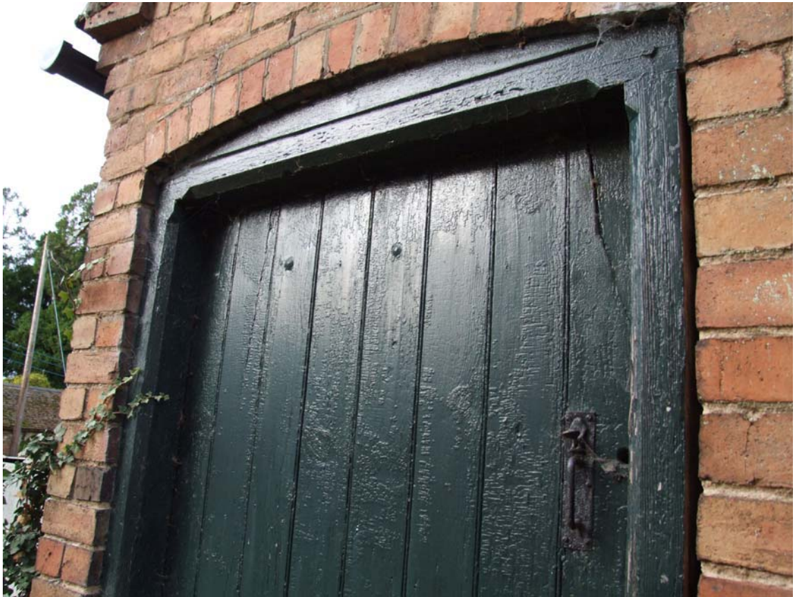
Plate 3: Original door with chamfered and stopped frame
