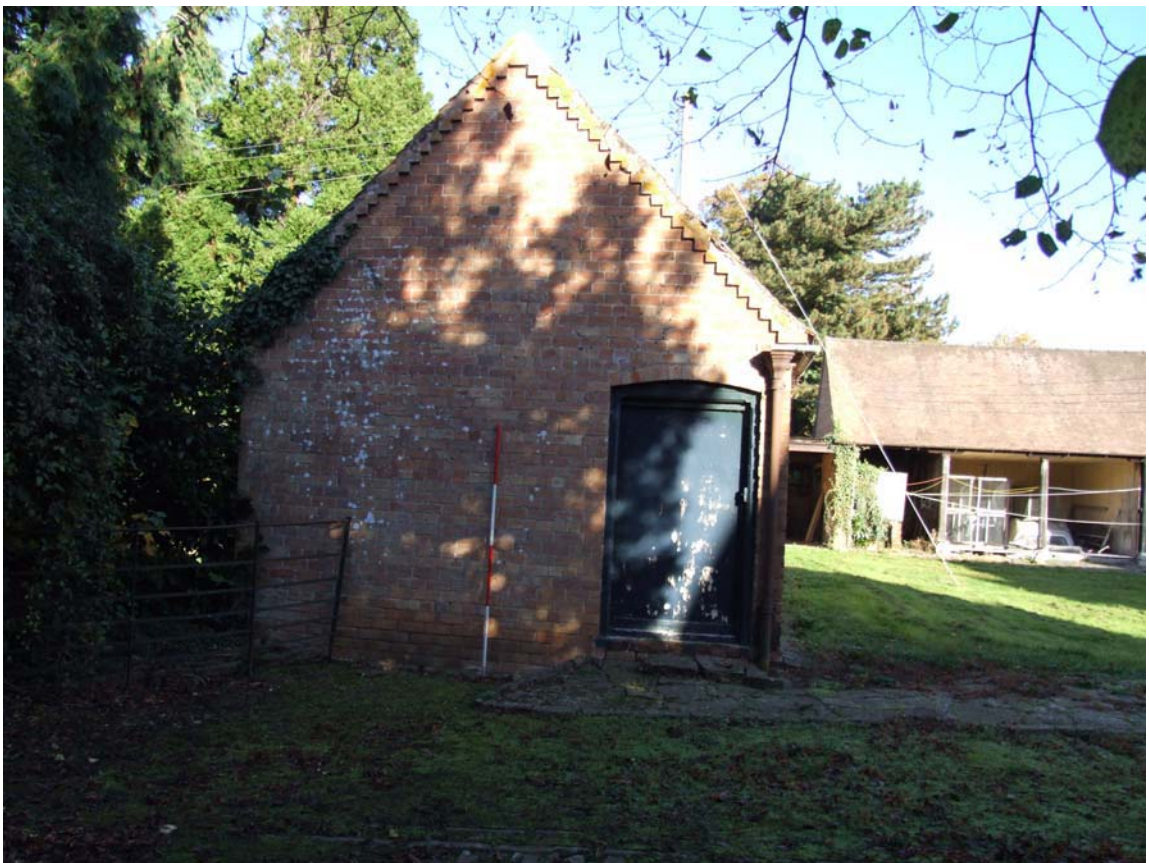
Plate 22: Feed processing block at the southern end of the western range
