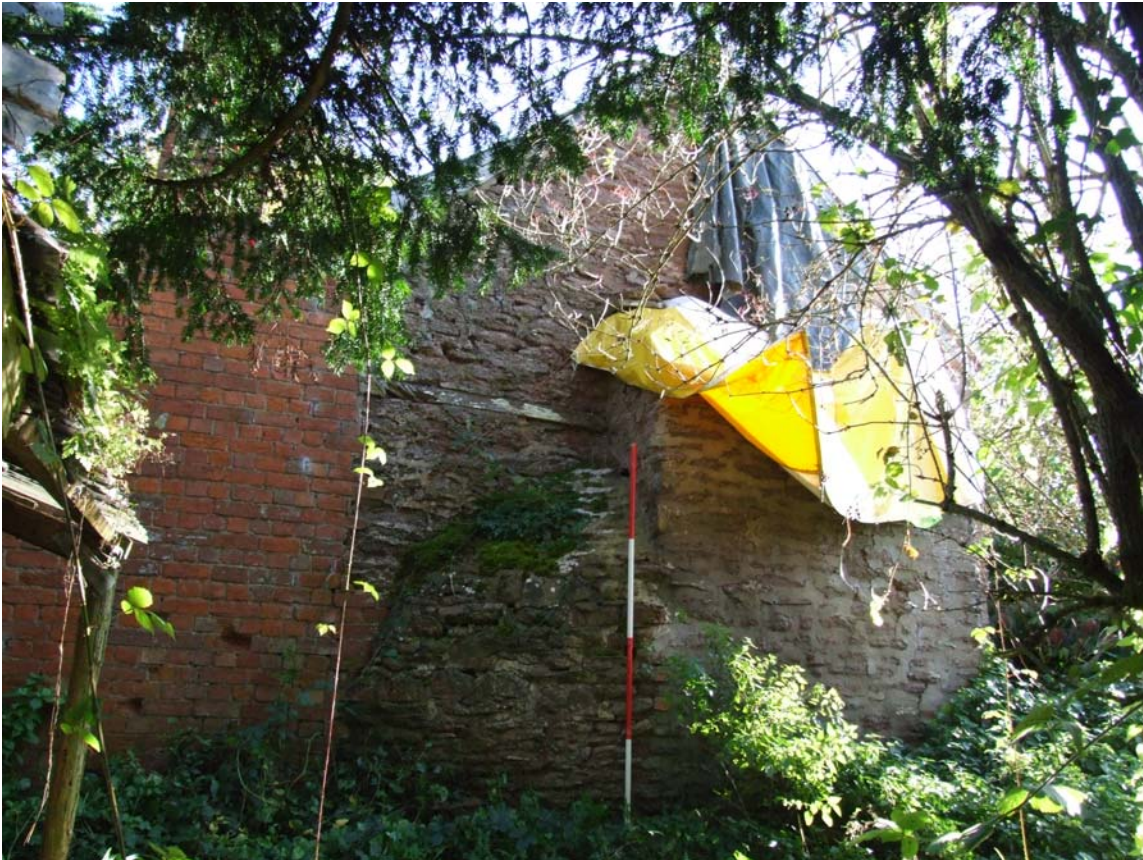
Plate 5: Western gable end (scale 2-metres)
