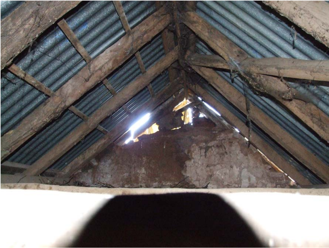
Plate 11: The roof space looking west
