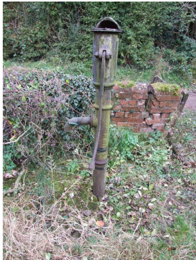
Plate 22: The water pump
