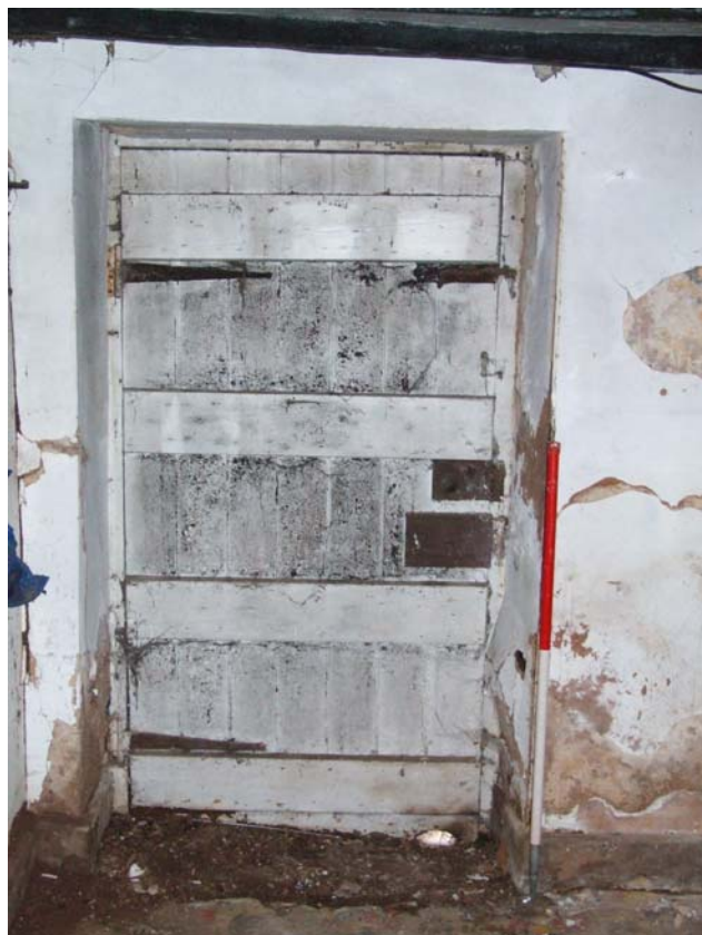
Plate 8: Door in the southern elevation (scale 1-metre)
