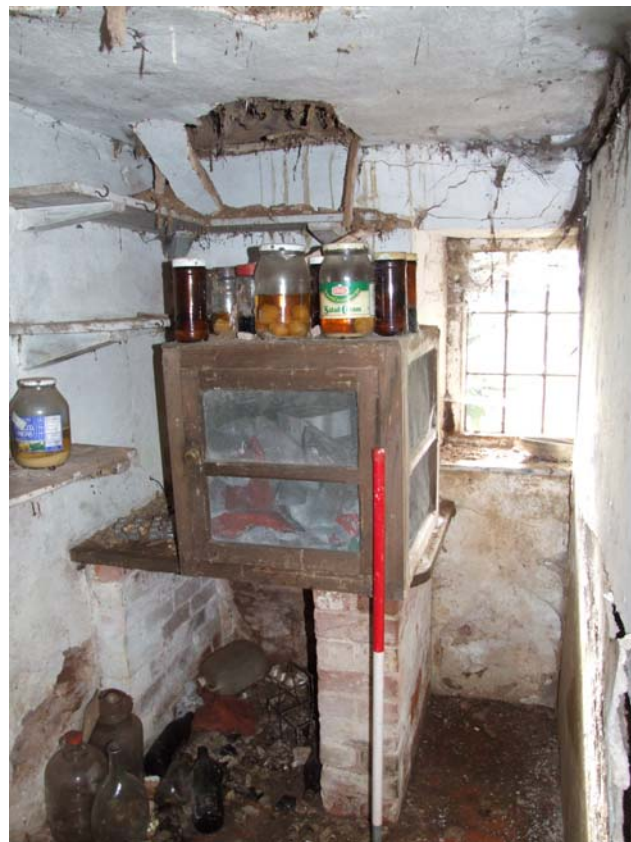
Plate 14: The pantry looking south (scale 1-metre)
