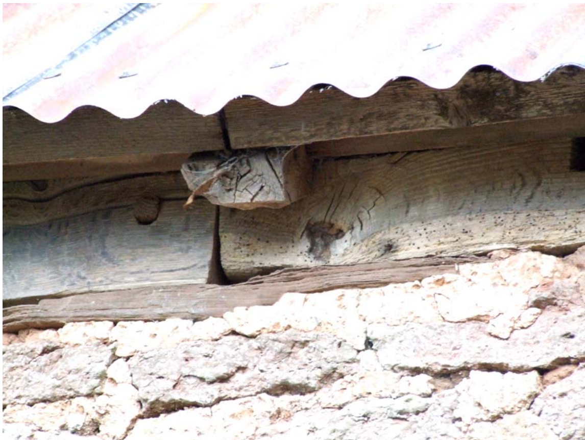
Plate 10: The southern wall plate
