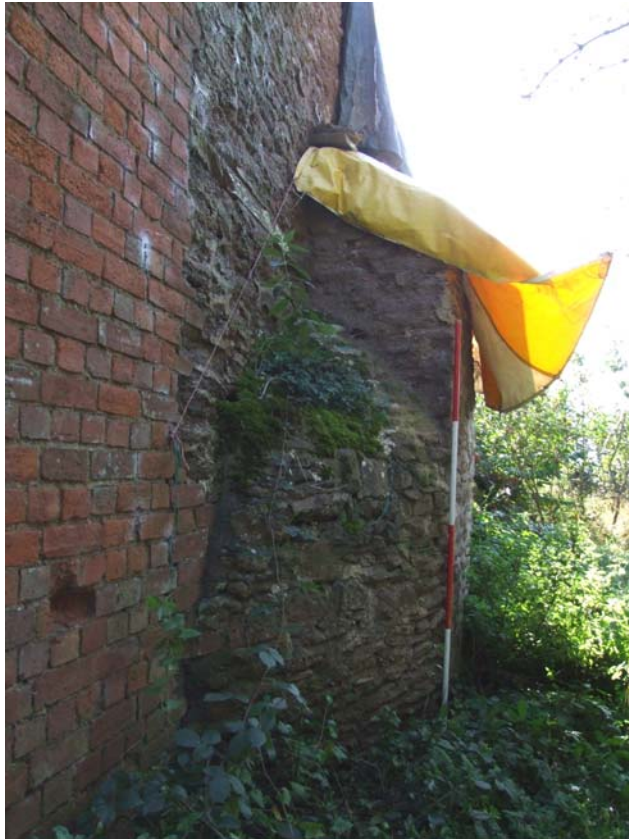
Plate 9: The bread oven wall against the chimneystack (scale 2 metres)
