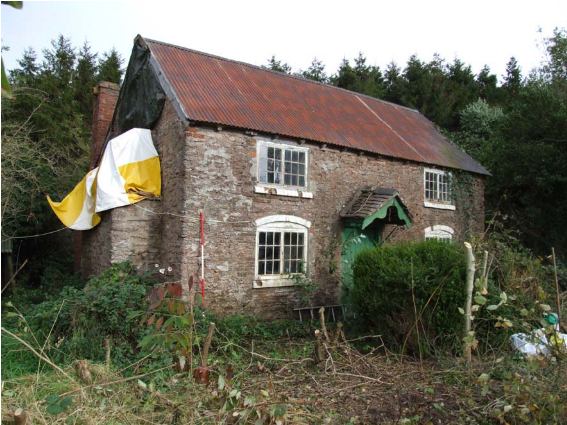
Plate 2: View to the north-east (scale 2-metres)
