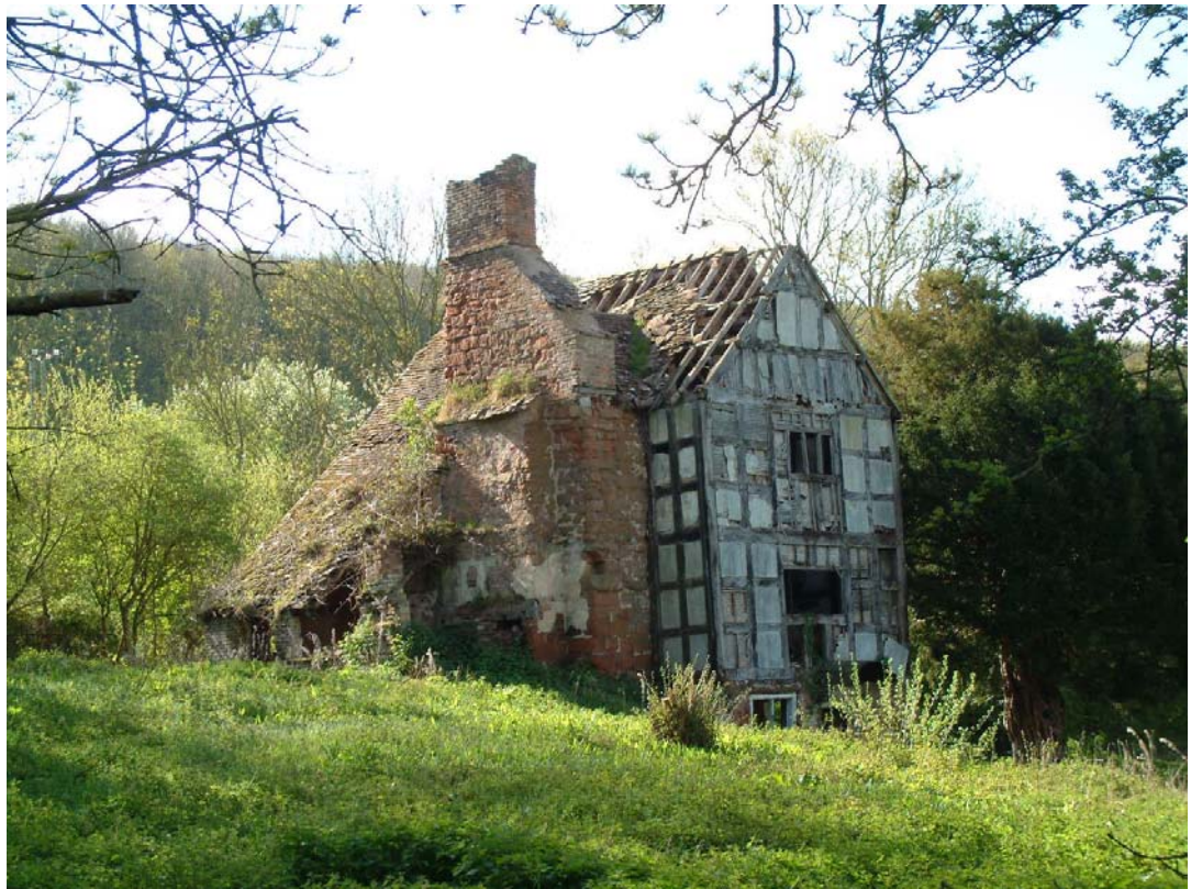
The Old Court looking south-east.
