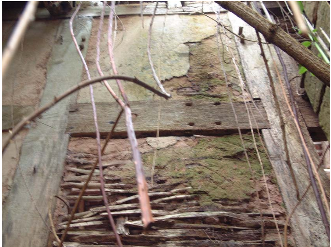
Replacement timber framing at The Old Court (see Plate 16)
