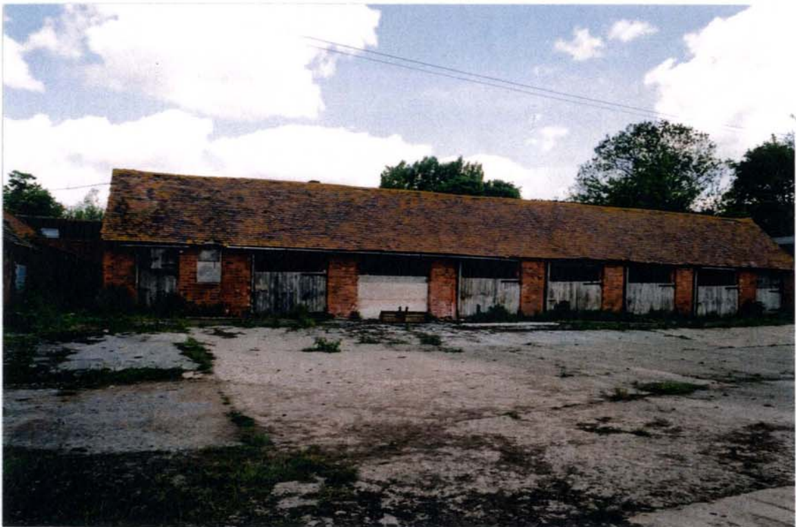
Fig 17: South elevation; north range
