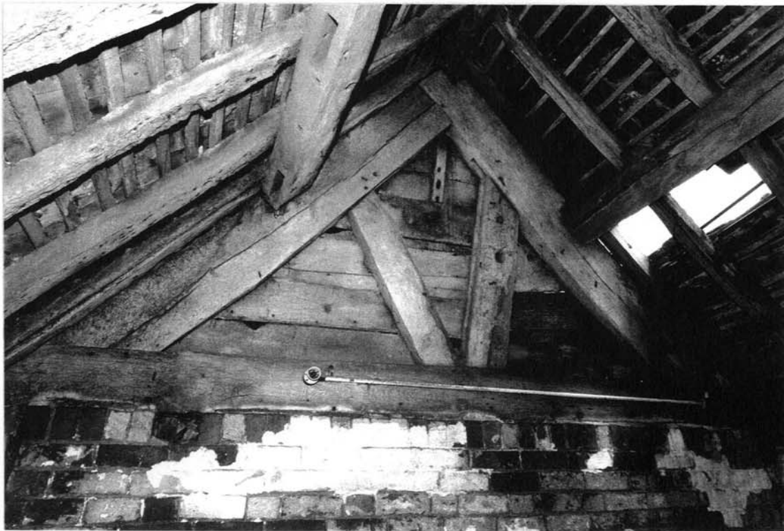
Fig 21: Roof truss; west range
