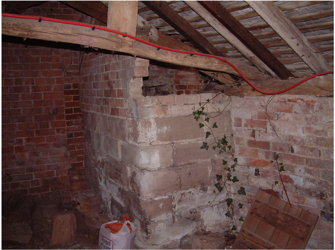
Plate 4: Southern post of central truss of the former detached building, showing 40 cm gap to the hall (Scale 2 metres)
