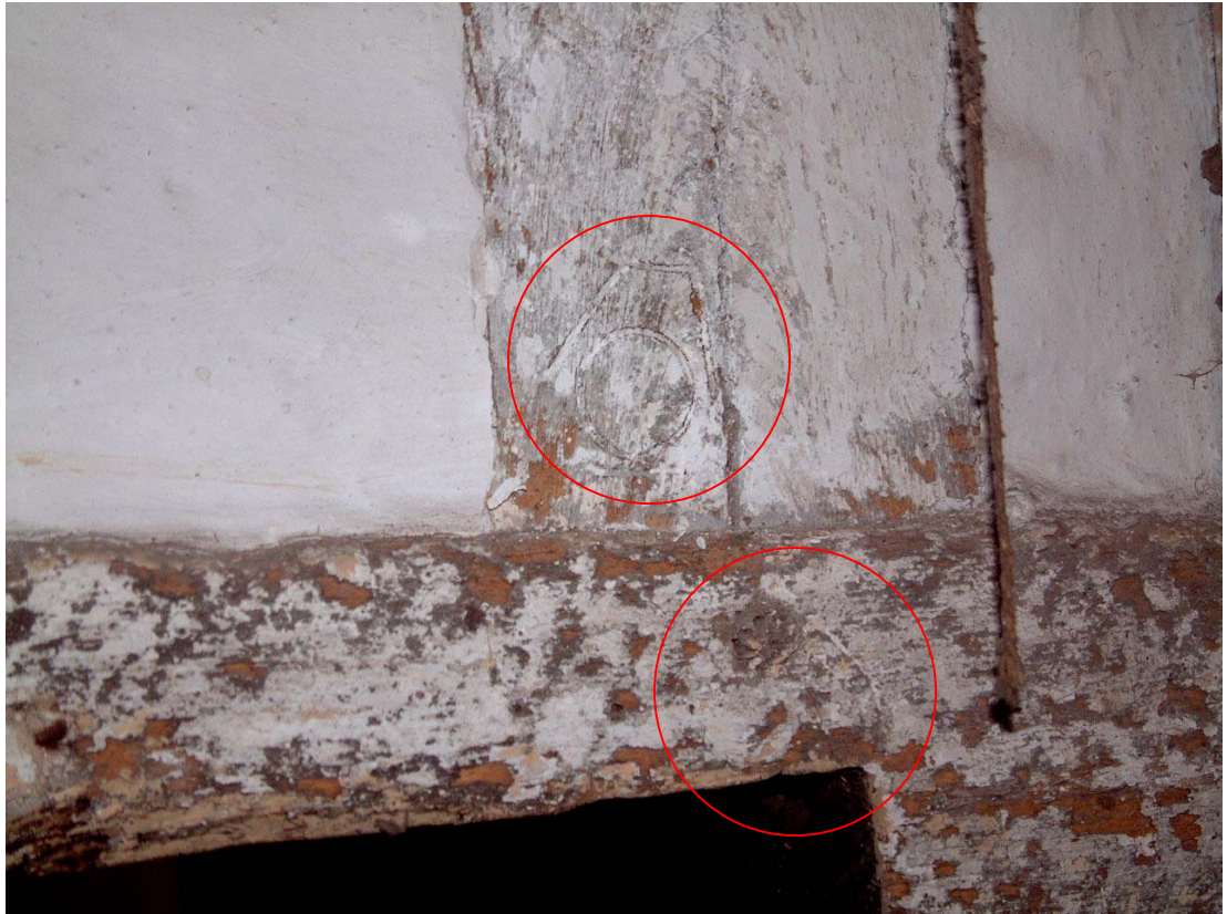
Plate 9: Carpenters assembly marks on the studding and tiebeam of the northern hall frame (northern face)
