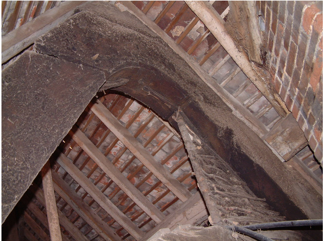
Cruck-saddle and remaining wattles above the collar
