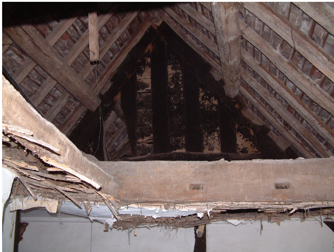
Northern frame of the hall viewed to the south
