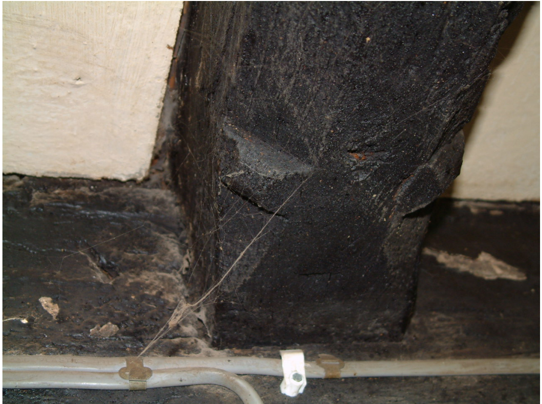
Chamfer and stops on bridging beam within the hall
