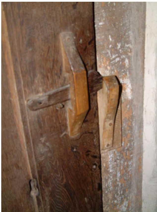
17 th century door catch (service chamber at northern cross-wing)
