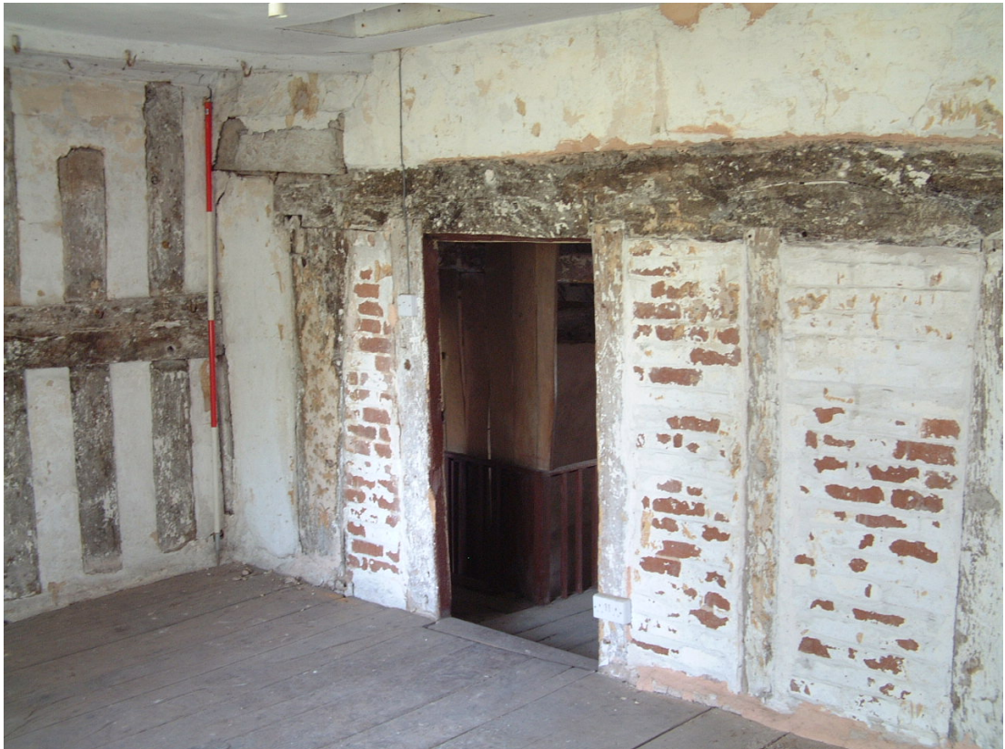
Plate 4: Southern post of central truss of the former detached building, showing 40 cm gap to the hall (Scale 2 metres)
