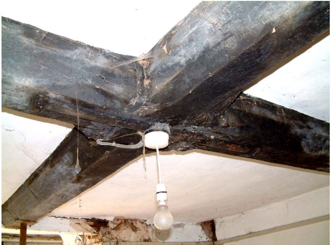
Pyramid stops on bridging beams in the southern cross-wing
