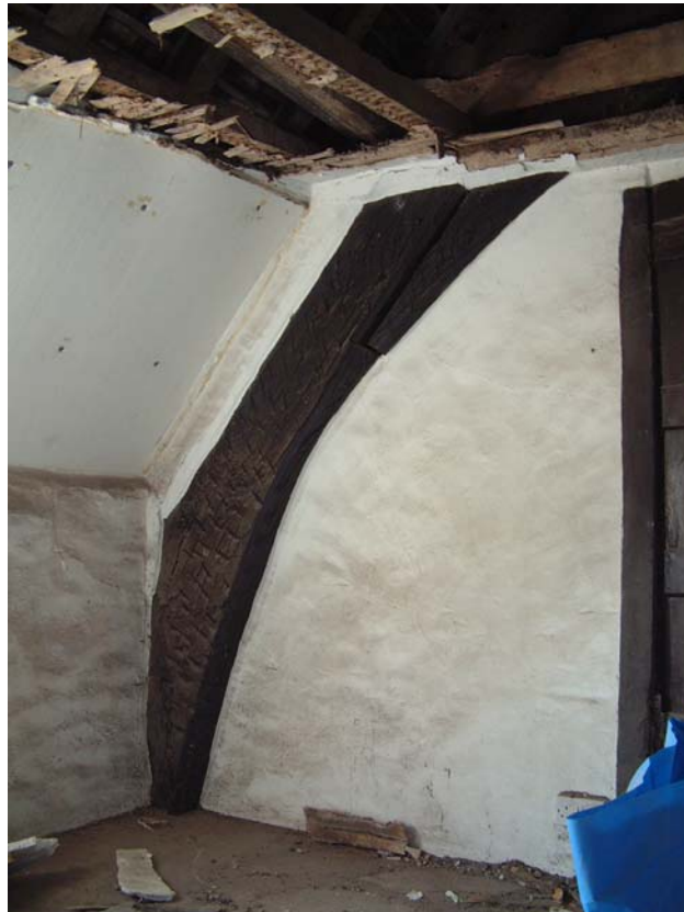
Cruck-frame at first floor level
