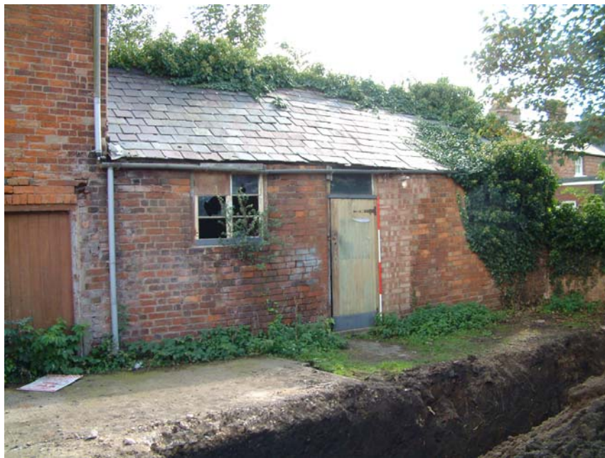
Plate 4: The single storey structure adjoining the tower, looking south-east (scale 2 metres)
