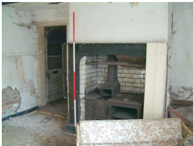
Plate 7: Cast-iron range inside the street frontage building (scale 2 metres)
