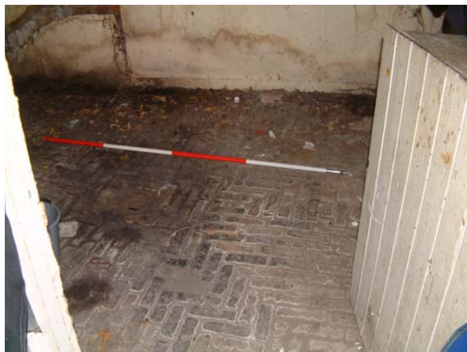
Plate 8: Brick floor and central drain (scale 2 metres)
