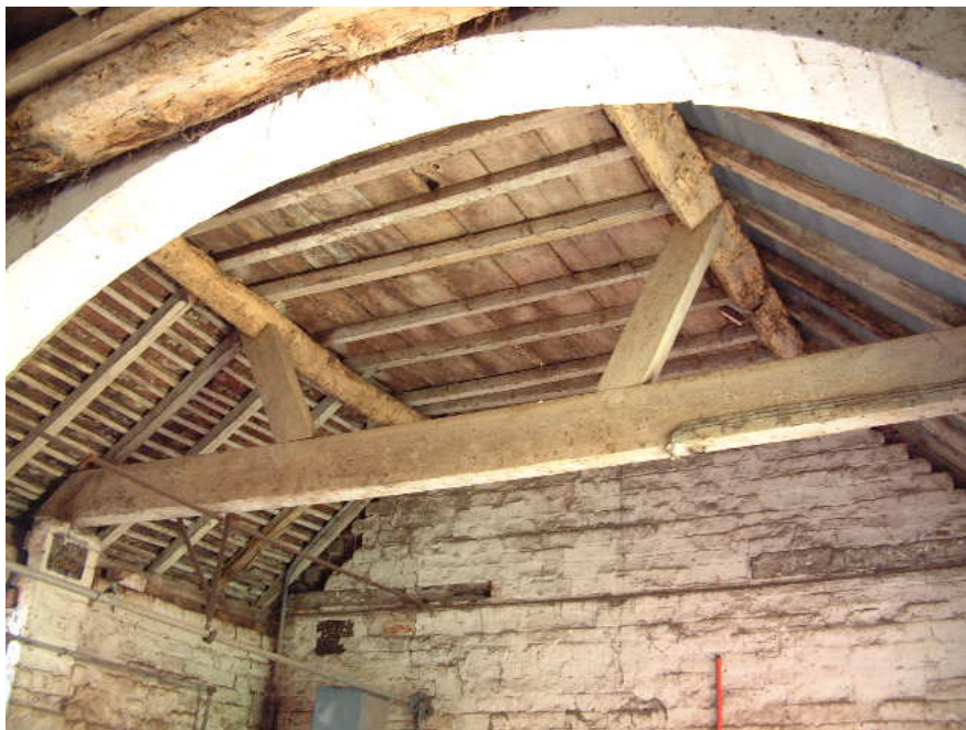
Queen-post half truss in projection at northern end of Building 2
