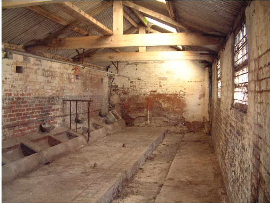
Interior of cowhouse, Building 4 (scale 1 metre)
