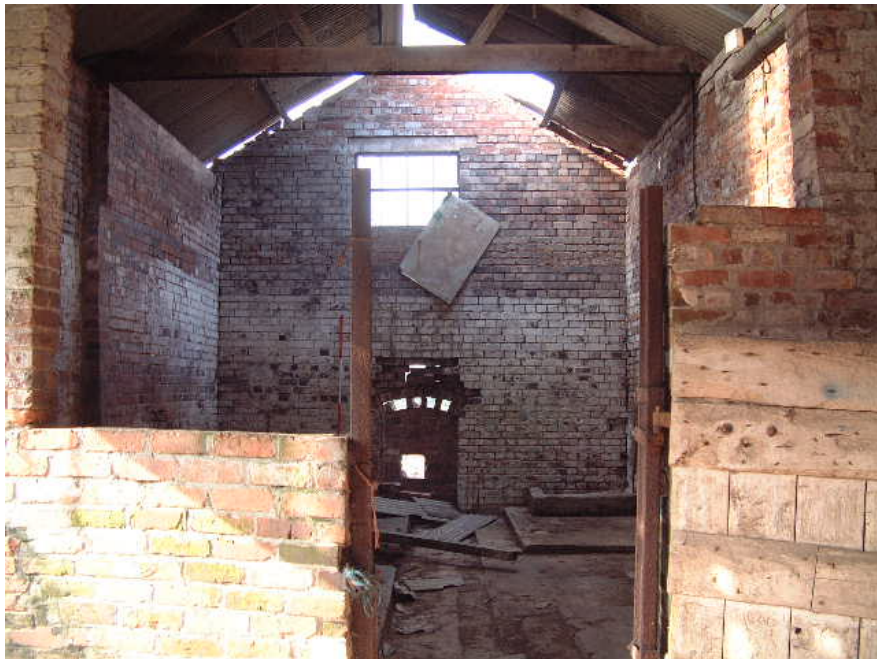
Extension to the southern end of Building 3 (scale 2 metres)
