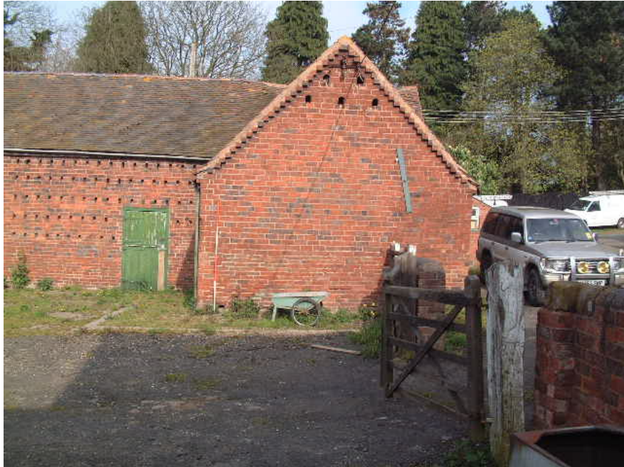
Pigeon loft in the gable of the northern projection of Building 2 (scale 2 metres)
