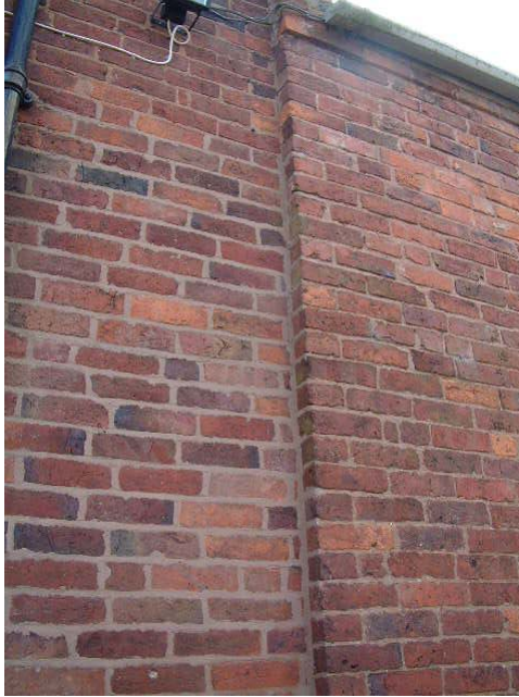
Joint between Building 3 and the farmhouse
