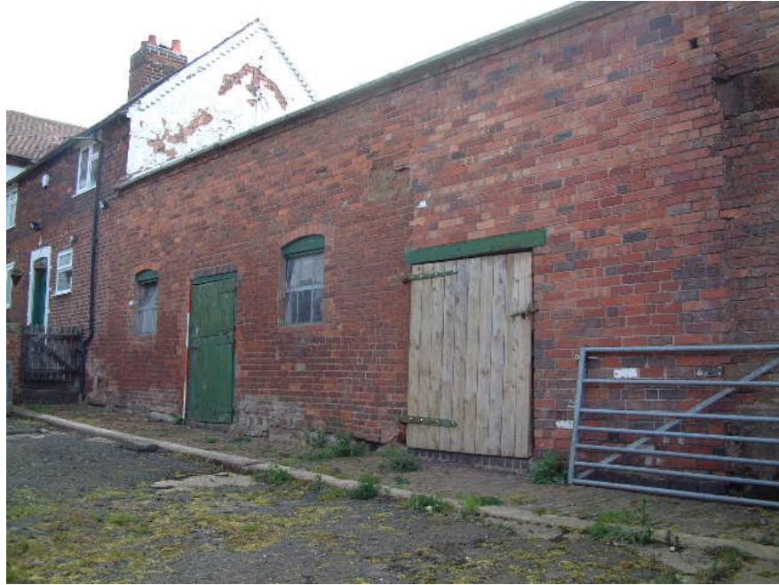
Building 3 looking north-east. Note the bricked up cartway (scale 2 metres)
