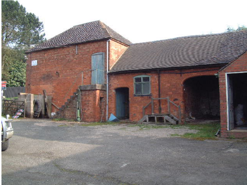
Building 1 viewed to the north
