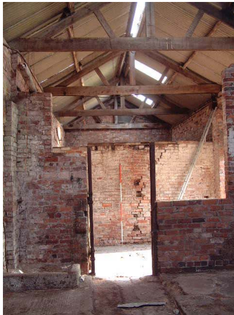
King-post trusses in Building 3, looking north (scale 2 metres)
