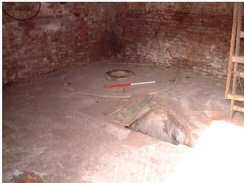
Modern grain processing infrastructure in Building 2 (scale 1 metre)
