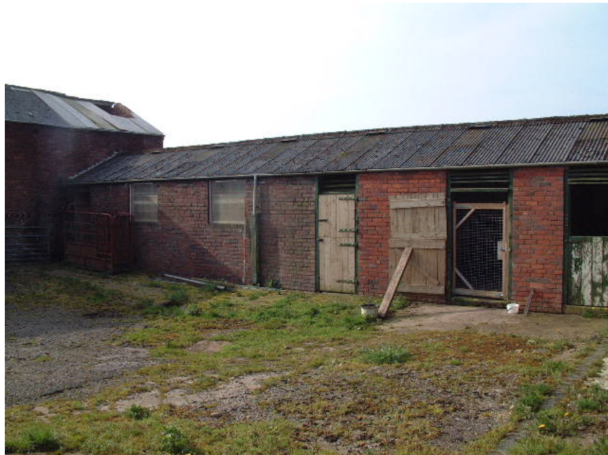
Building 4 looking south (scale 2 metres)
