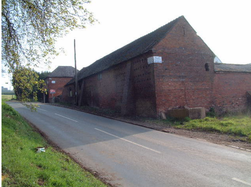
Building 2 viewed to the north-east
