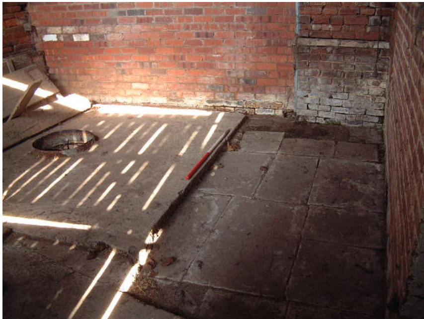
Threshing floor in Building 2 (scale 2 metres)
