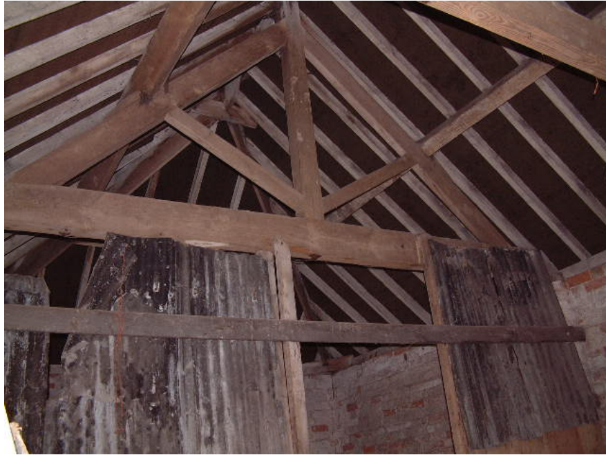
King post truss in Building 1
