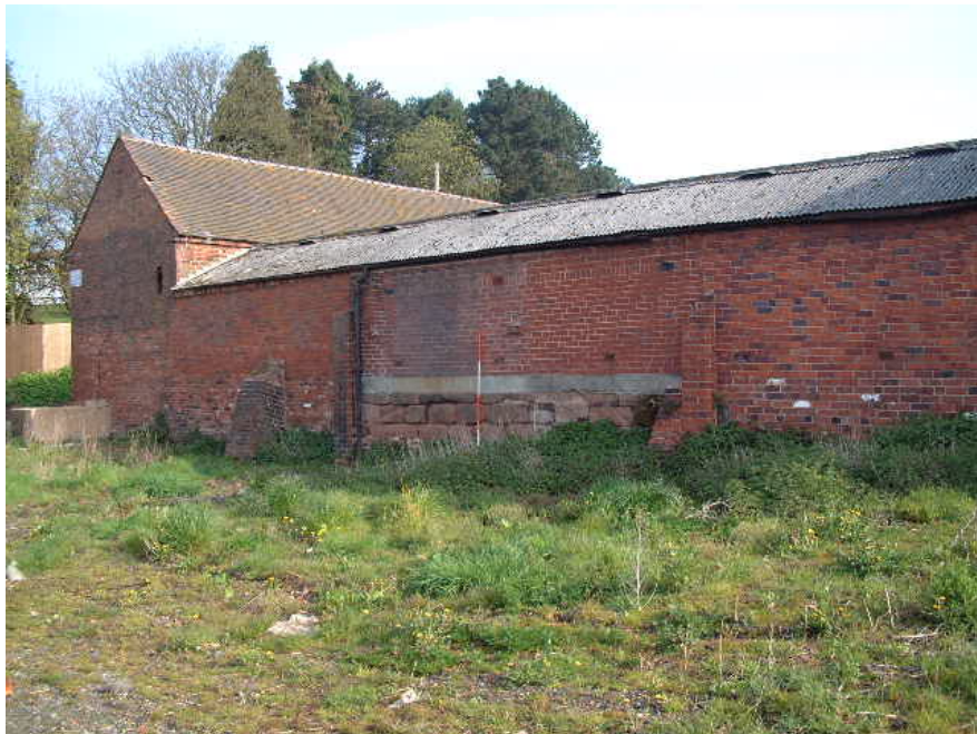
Sandstone wall within the fabric of Building 4, looking north (scale 2 metres)
