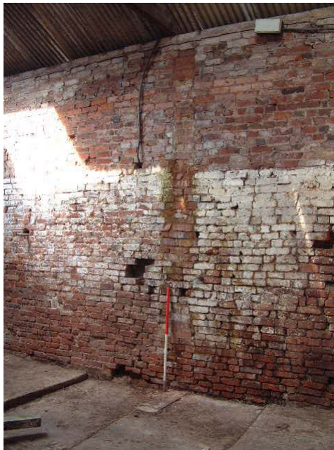
Rough construction of the extension at the northern end of Building 3
