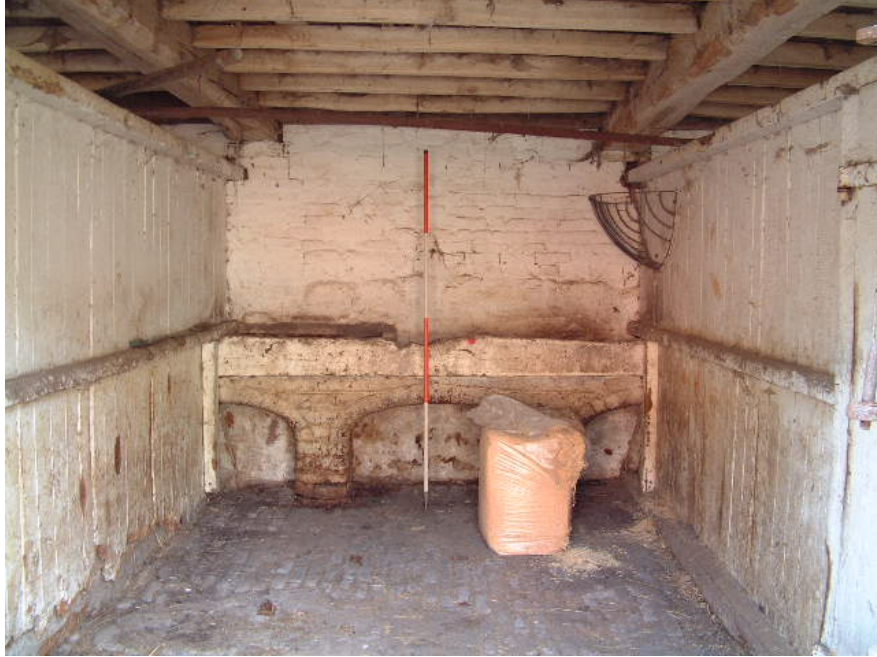
Inside stable within Building 3 (scale 2 metres)
