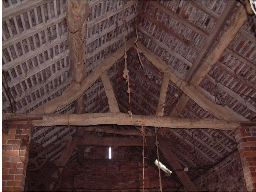
Queen strut trusses in Building 2
