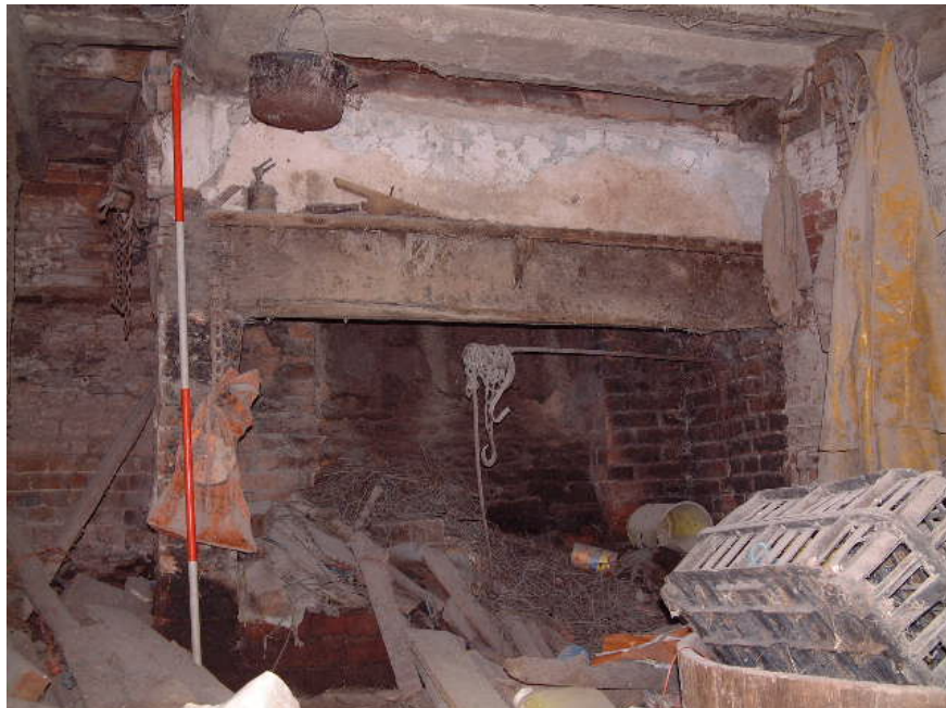
Hearth with iron spit below mantel beam, probably 19 th century (scale 2 metres)
