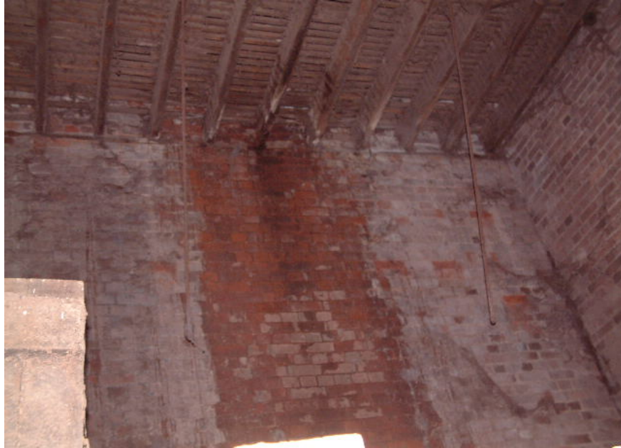
The laths of the drying floor in one of the hop kilns
