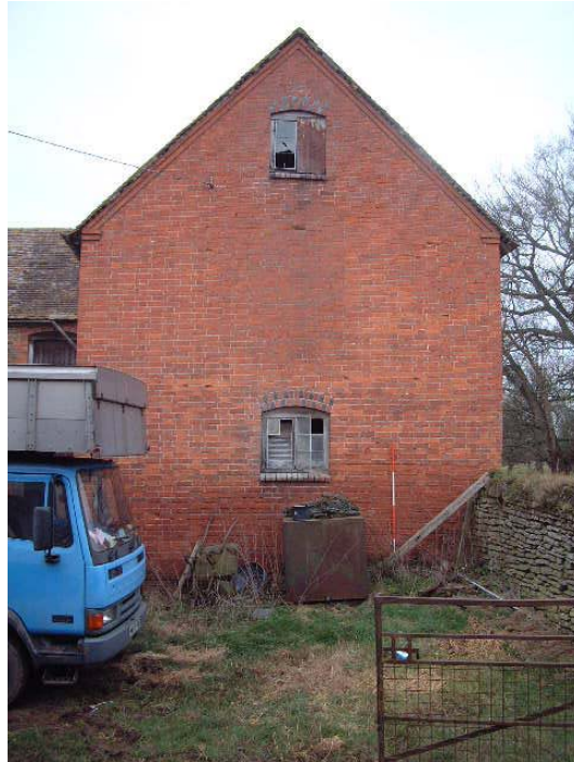
Gable end at south of farmhouse (scale 2 metres)
