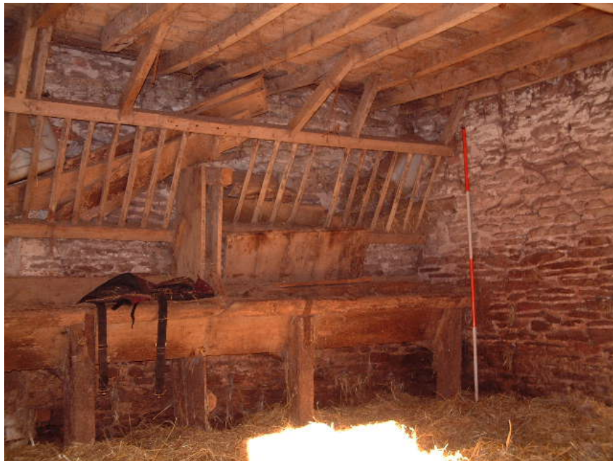
Space C (stables) looking north-east (scale 2 metres)
