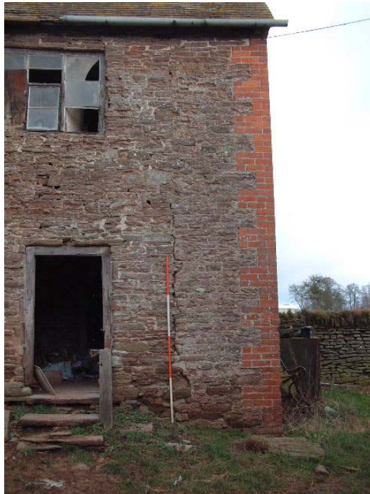
Rebuilt stonework tied into the newer brick southern elevation
