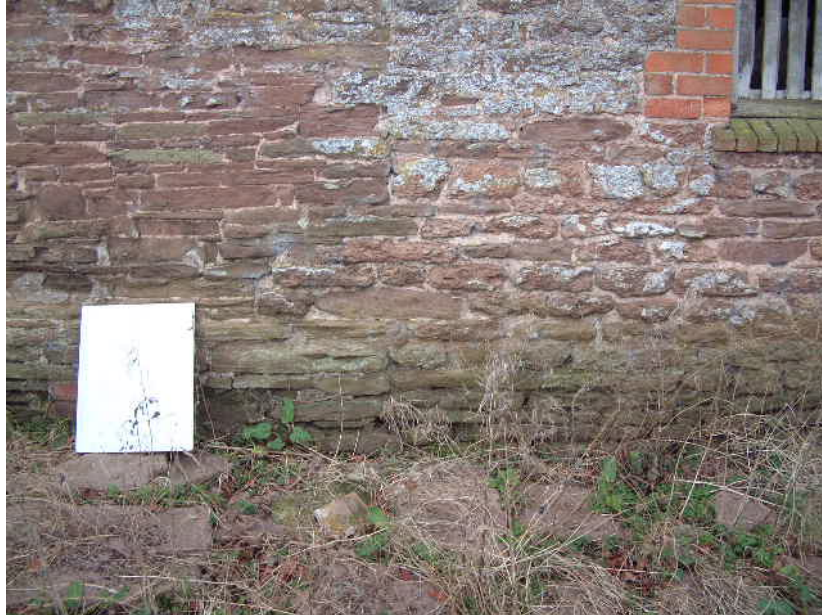
The stonework at the base of the build continues past the north eastern corner of the gable of the farmhouse, the extension (right) is built onto it (see text)
