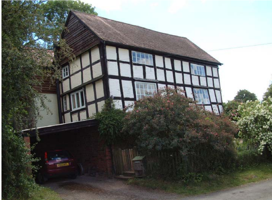
The Boathouse looking east
