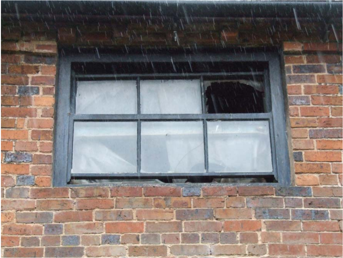
Plate 21: 6-light sash window
