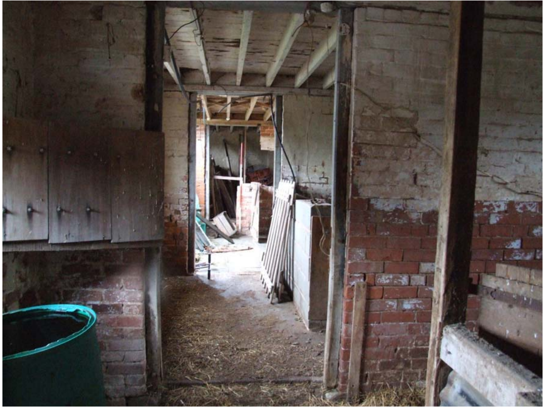
Plate 7: View to the west from cross passage (B), showing bay division for loose boxes
