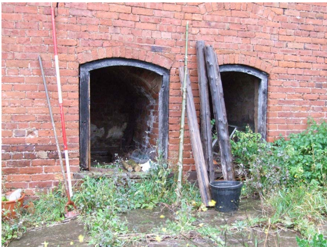
Plate 18: Dog kennels at west end of south elevation
