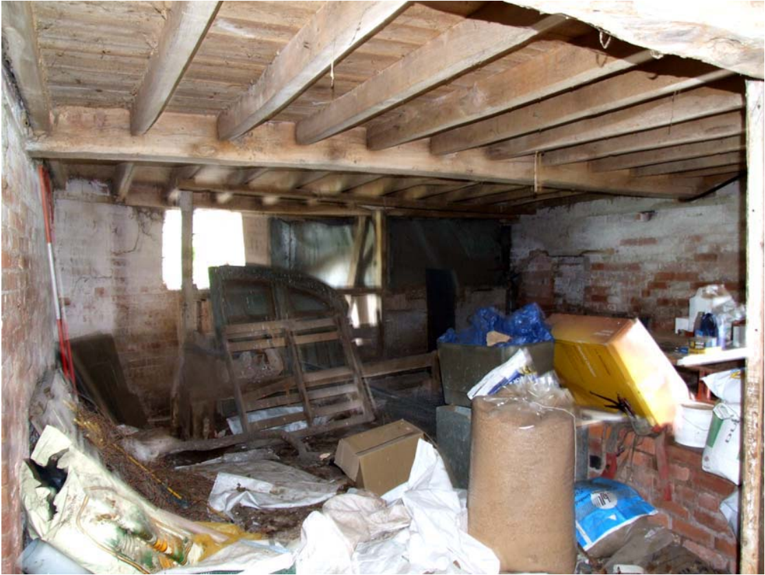
Plate 13: Space C looking north-east
