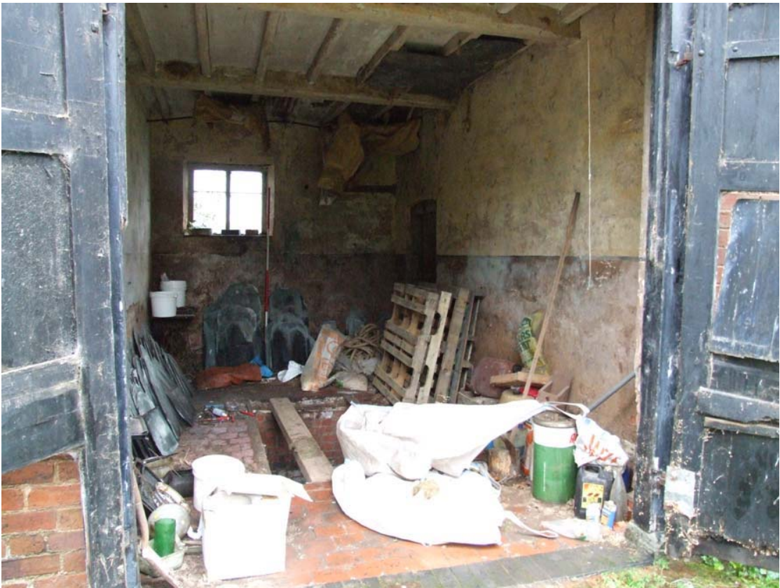
Plate 14: Garage pit in space D2
