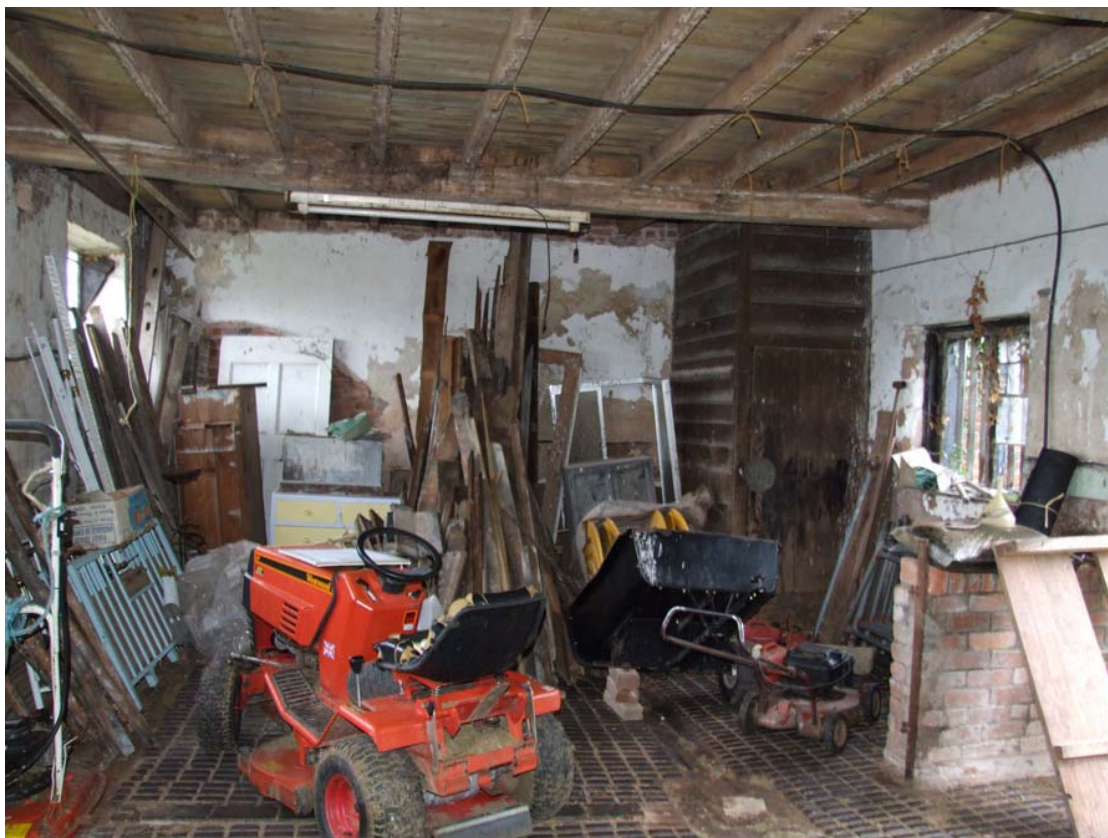
Plate 15: Space E looking west
