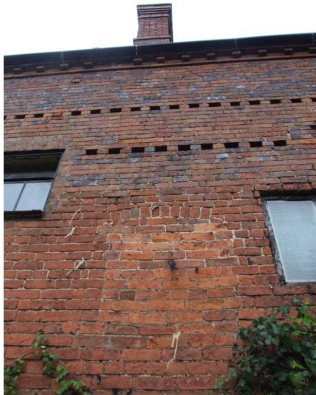
Plate 11: Blocked window with inserted chimney behind, northern side of D3
