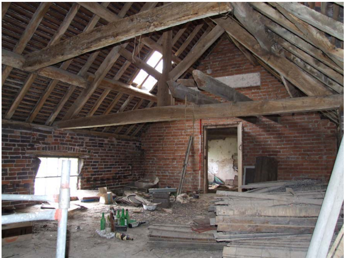
Plate 25: Timbers above space E
