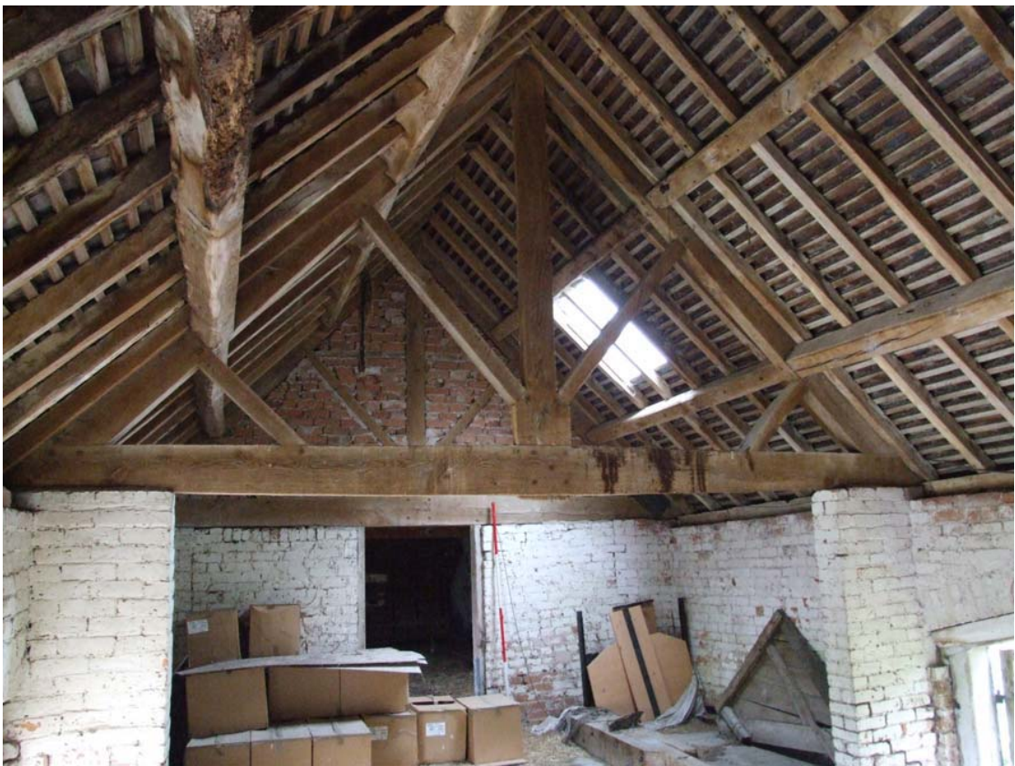
Plate 23: Typical truss
