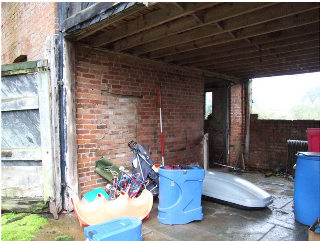
Plate 12: Blocked doorway in inserted bay partition (A3)
