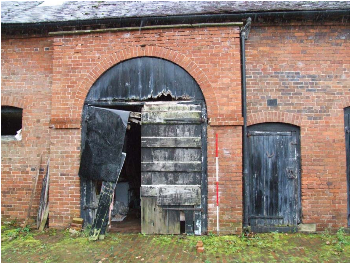
Plate 10: Added embellished doorway to the southern elevation of A5
