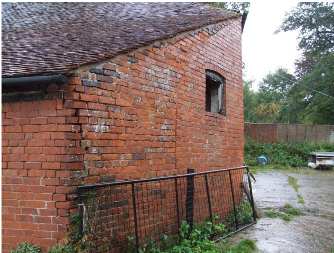
Plate 17: Scar of former roofline and front wall of second phase piggery
