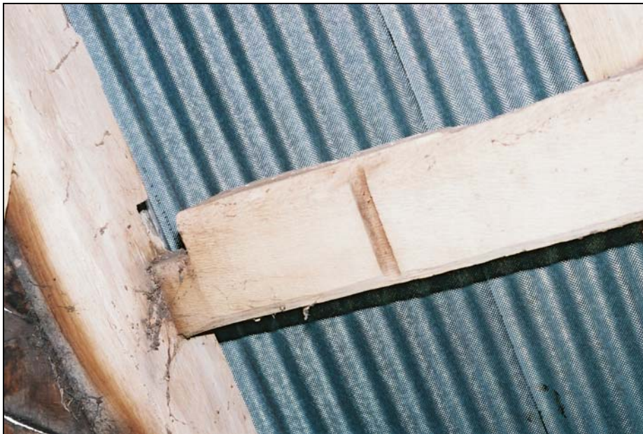
This purlin has been made from a re-used timber. Note the remains of the peg hole; showing the timber has been cut along its length
