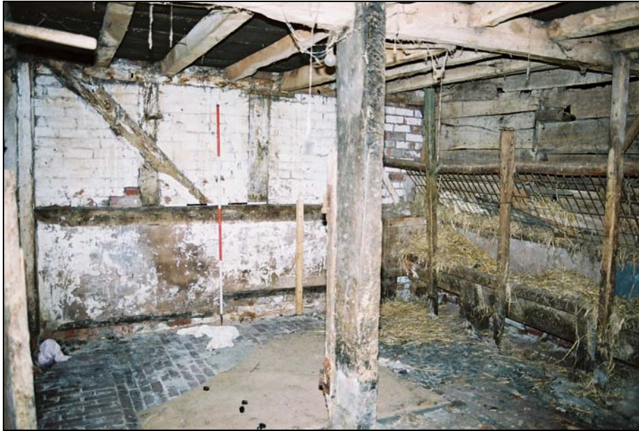
Bay 1 (lower) showing the inserted hayloft above and the part cobbled floor
