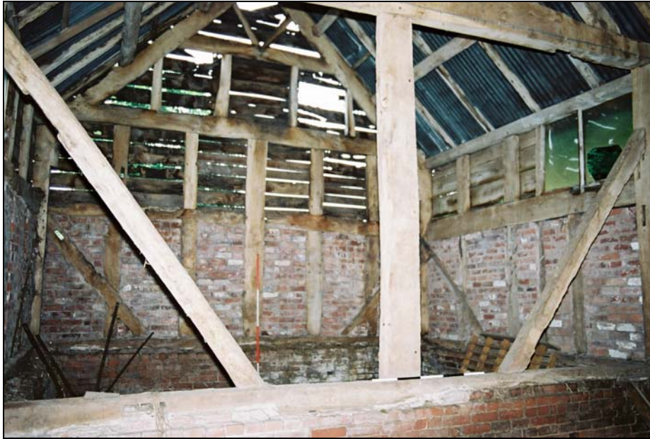
Truss T6 and Bay 5 from Bay 4
