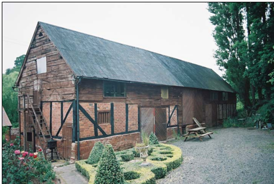
South elevation of the barn
