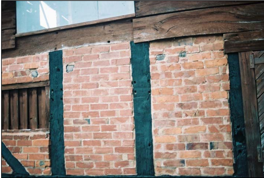
Unused peg holes on studs in Bay 2, indicating the position of a former rail forming square panelling
