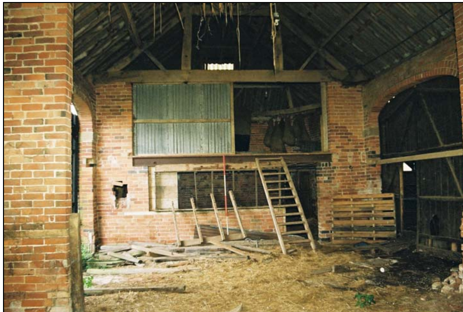
Building 8; truss above the hayloft
