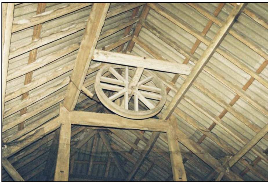
The sack hoist in Building 8
