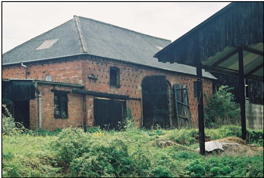
Building 8; the 3 bay threshing viewed to the southwest
