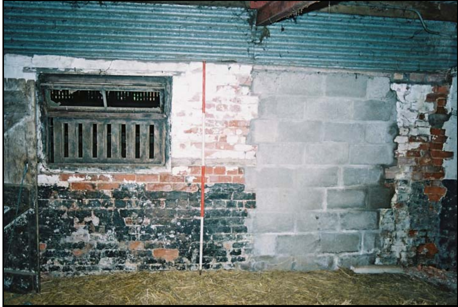
Building 6 showing the blocked up door and slatted vent
