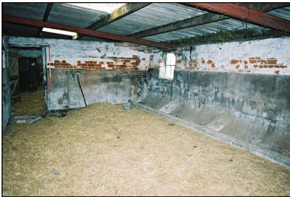
View from building 4, through Building's 5 and 6 towards the barn (scale 2 metres)
