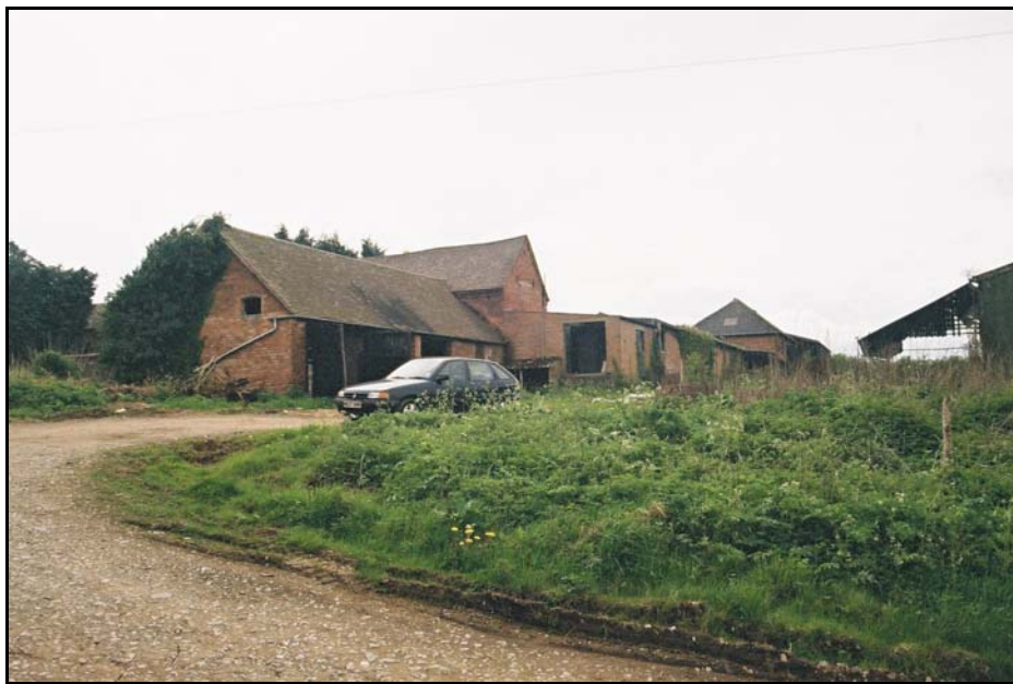
Building 1 viewed to the southwest
