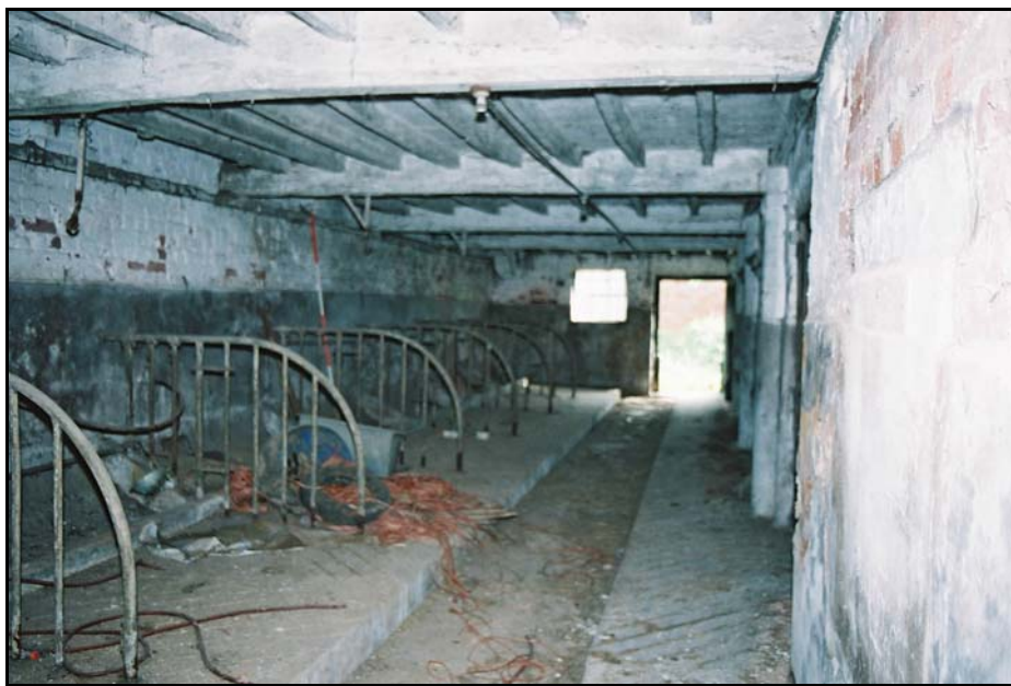
Building 2 showing animal feeding partitions (scale 2 metres)
