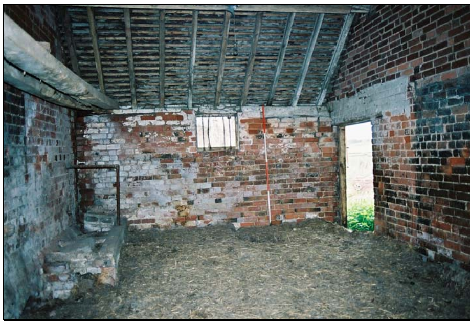
Building 1 showing arched drain in bottom left corner (scale 2 metres)
