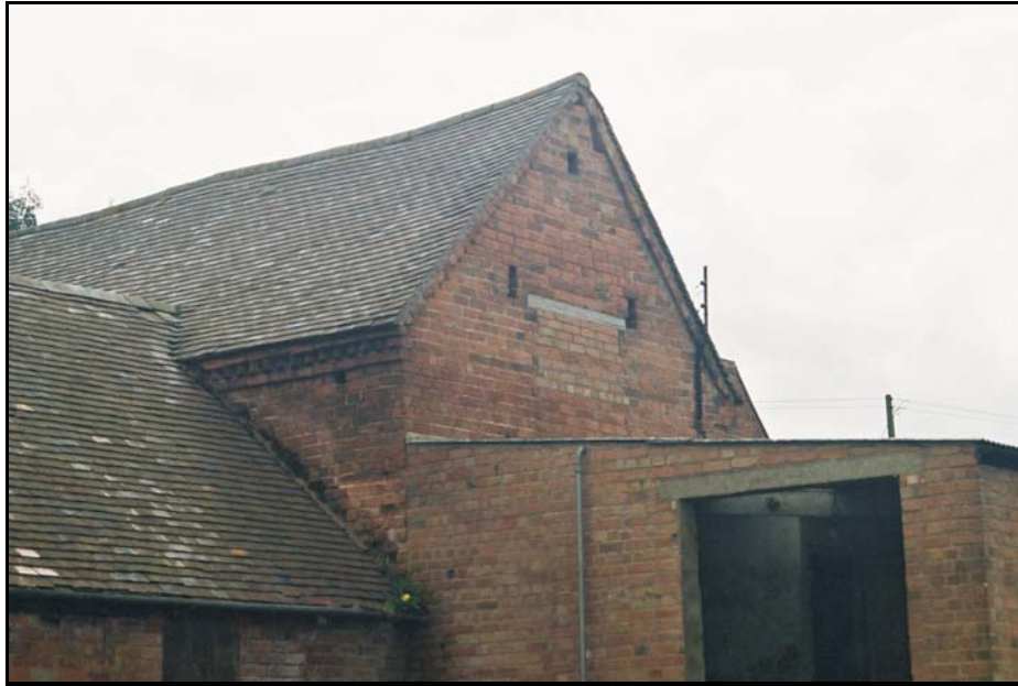
Building 2 showing bricked up pitching eye in former hayloft
