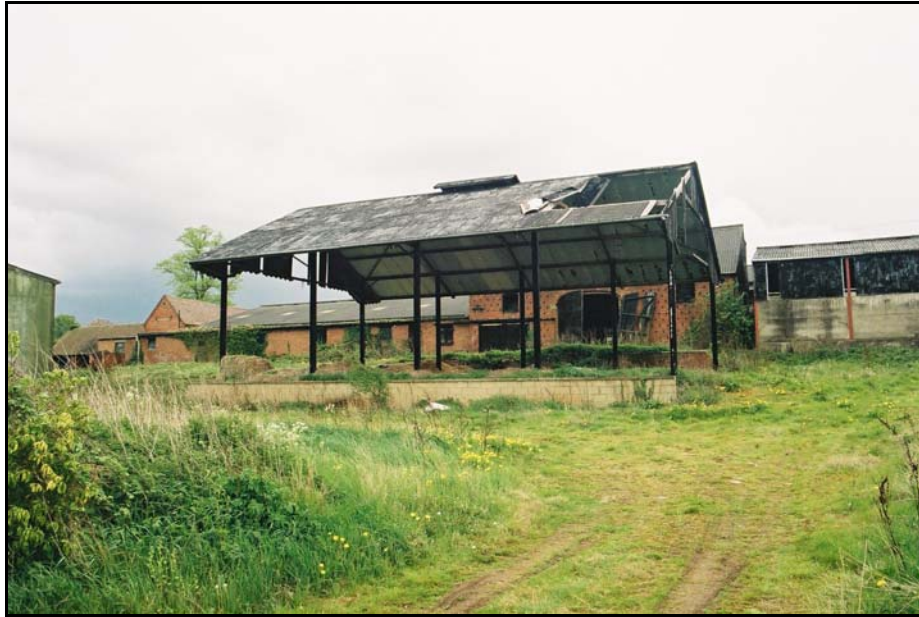
View of the farm complex looking south
