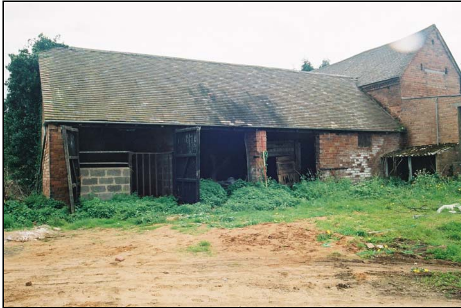
Building 1 looking south and showing detail (scale 2 metres)
