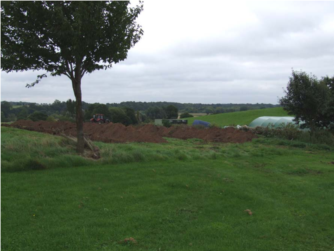
Plate 1: The site looking south-east
