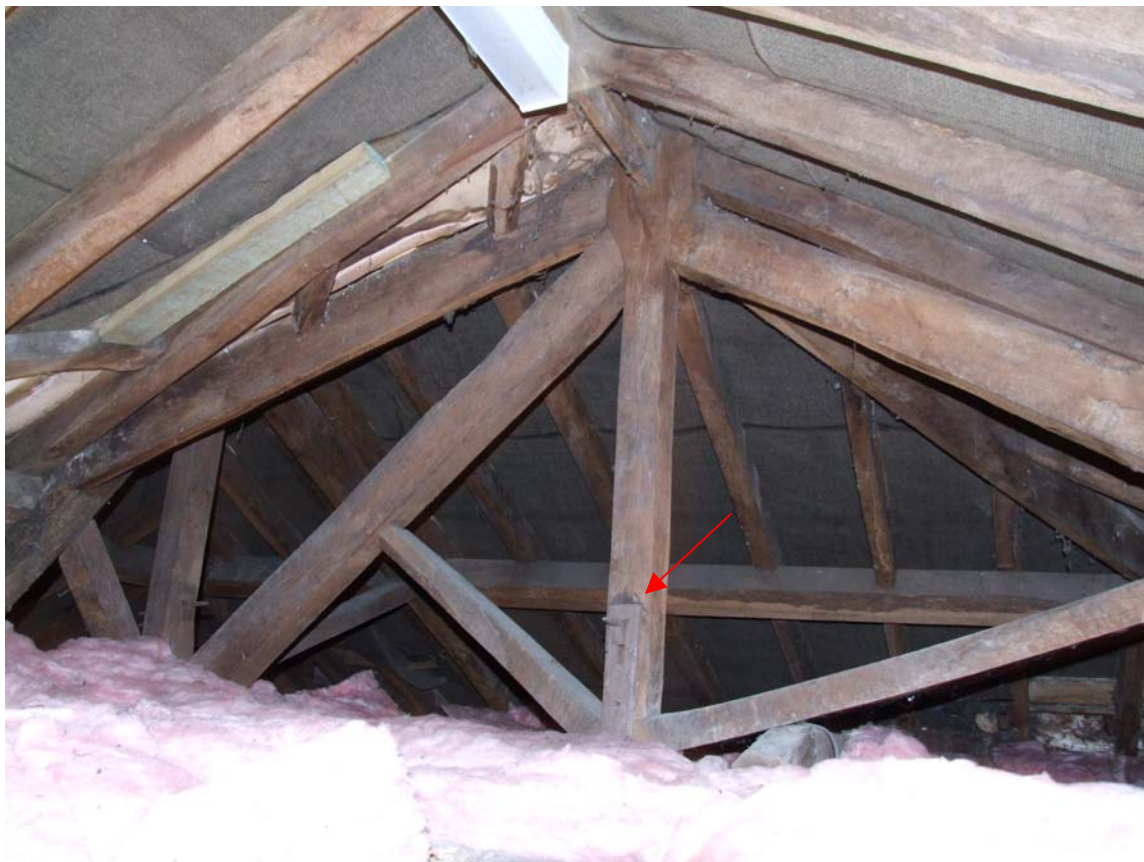
Plate 4: King-post roof truss with iron stirrup and cleat (arrowed)
