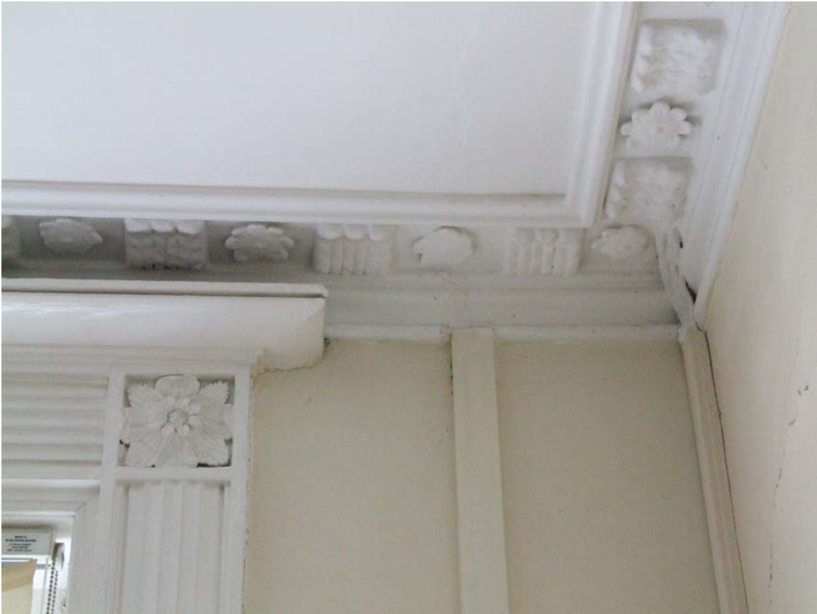
Plate 7: 1st floor cornice mouldings
