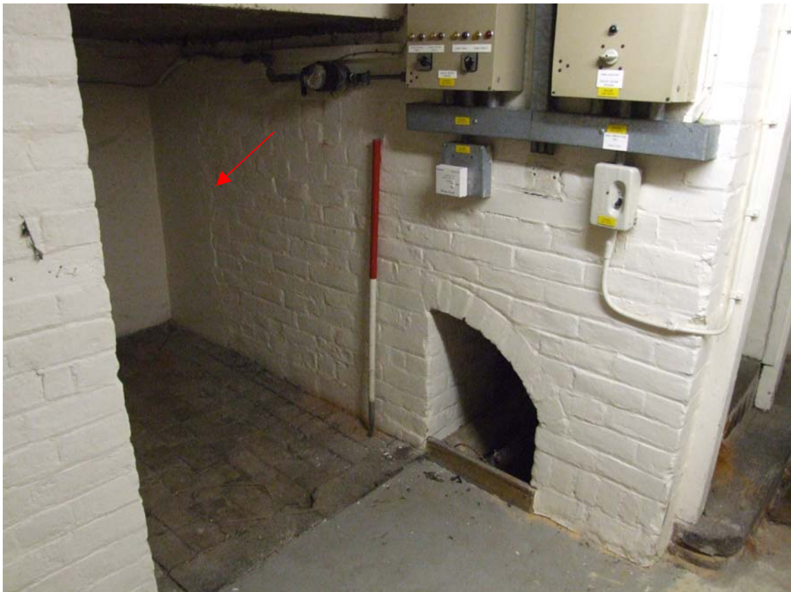
Plate 14: Cellar (below steps) showing possible alteration suggestive of blocking (Scale 2-metres)
