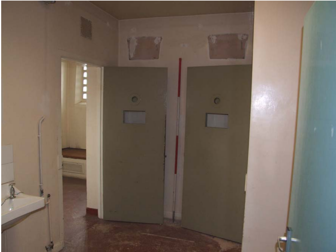
Plate 17: Entrance to the two cells (Scale 2-metres)
