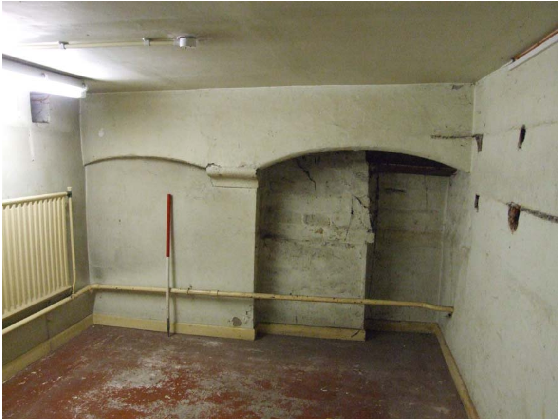
Plate 13: The former kitchen (Scale 1-metre)
