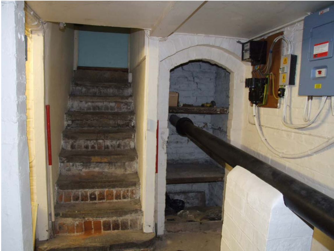
Plate 15: The cellar steps (Scale 1-metre)
