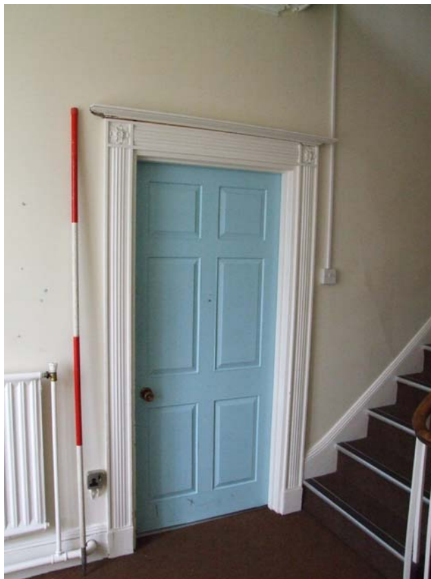
Plate 6: Original 1 st floor door and surround (Scale 2-metres)
