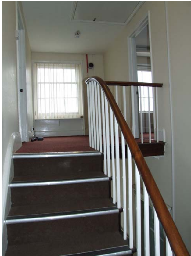
Plate 5: Staircase up to the 2 nd floor, taken from the half-landing
