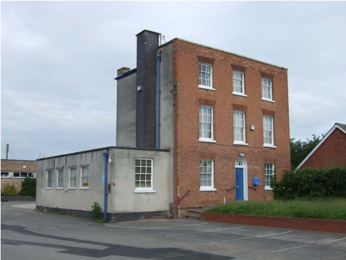
Plate 1: Front eastern elevation (scale 2-metres)
