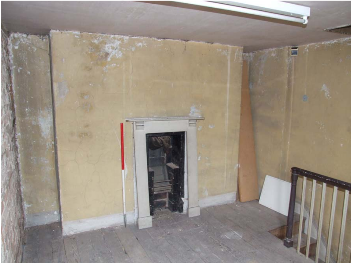
Plate 9: Rear servants bedroom (scale 1-metre)
