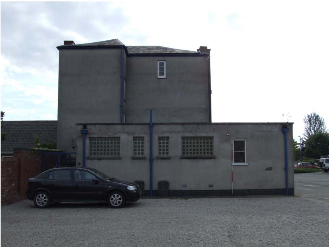
Plate 2: Rear western elevation (scale 2-metres)
