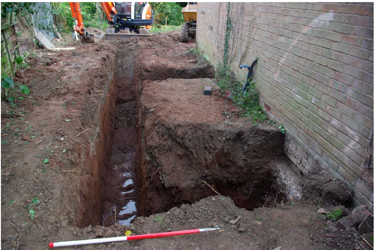
Plate 2: Work in progress at the site
