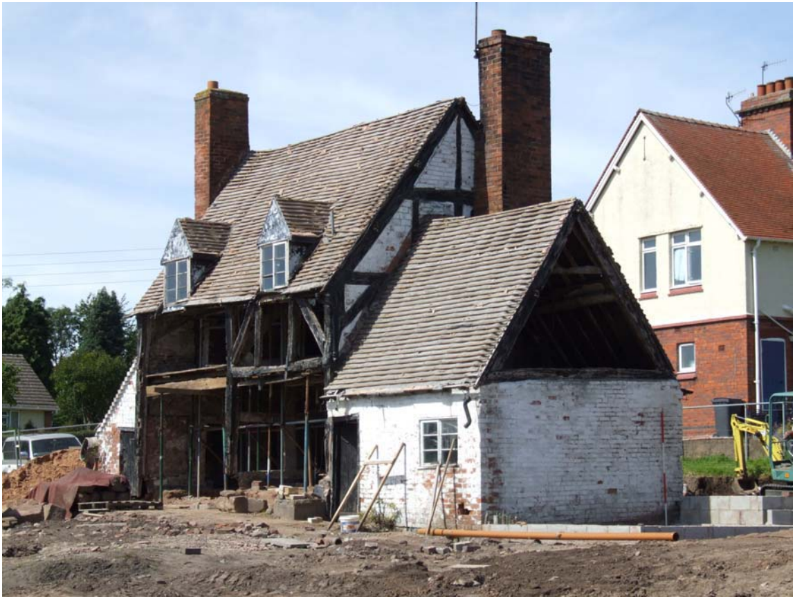
Plate 1: Cottage looking north-west (scale 2-metres)
