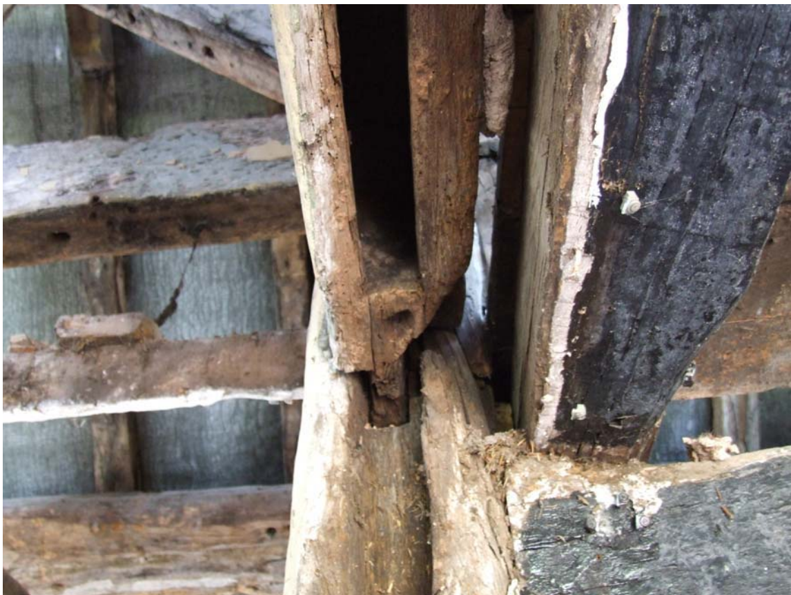
Plate 10: Slip tenon in T2, looking north
