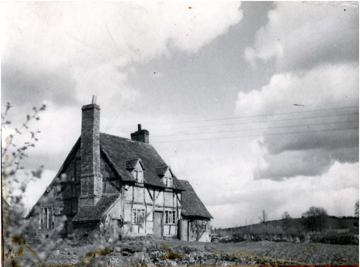
Plate 5: Steward's Cottage around 1950. Photograph kindly supplied by Rob Blakeway
