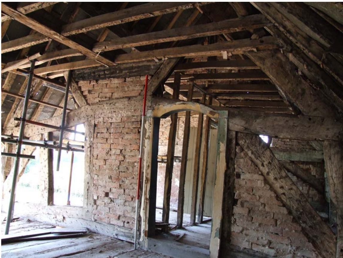
Plate 8: Truss T2 upper, view from Bay 2 (scale 2-metres)
