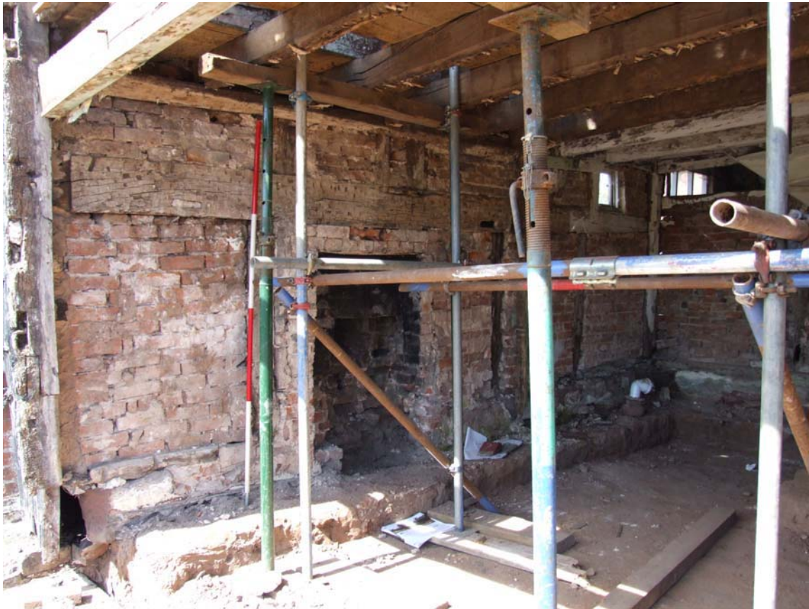
Plate 7: Frame T1 lower (scale 2-metres)
