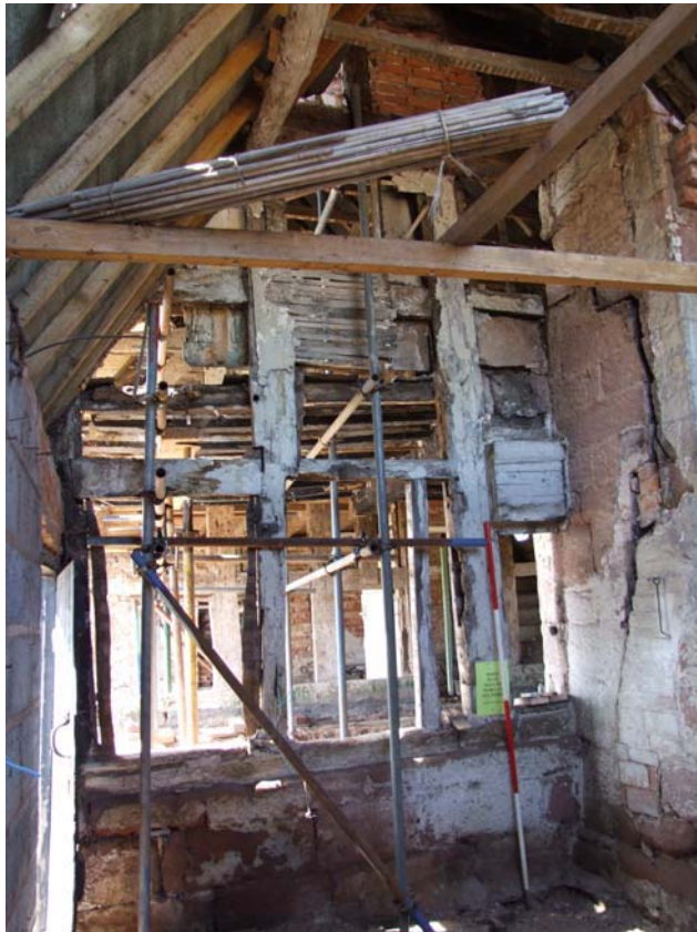
Plate 15: View of T3 from inside eastern extension (scale 2-metres)
