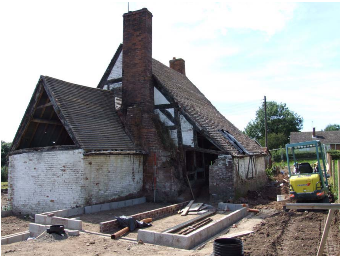
Plate 2: Cottage looking west (scale 2-metres)
