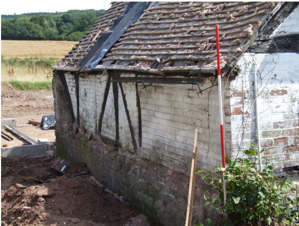
Plate 18: North frame of outshut looking south-east (scale 2-metres)
