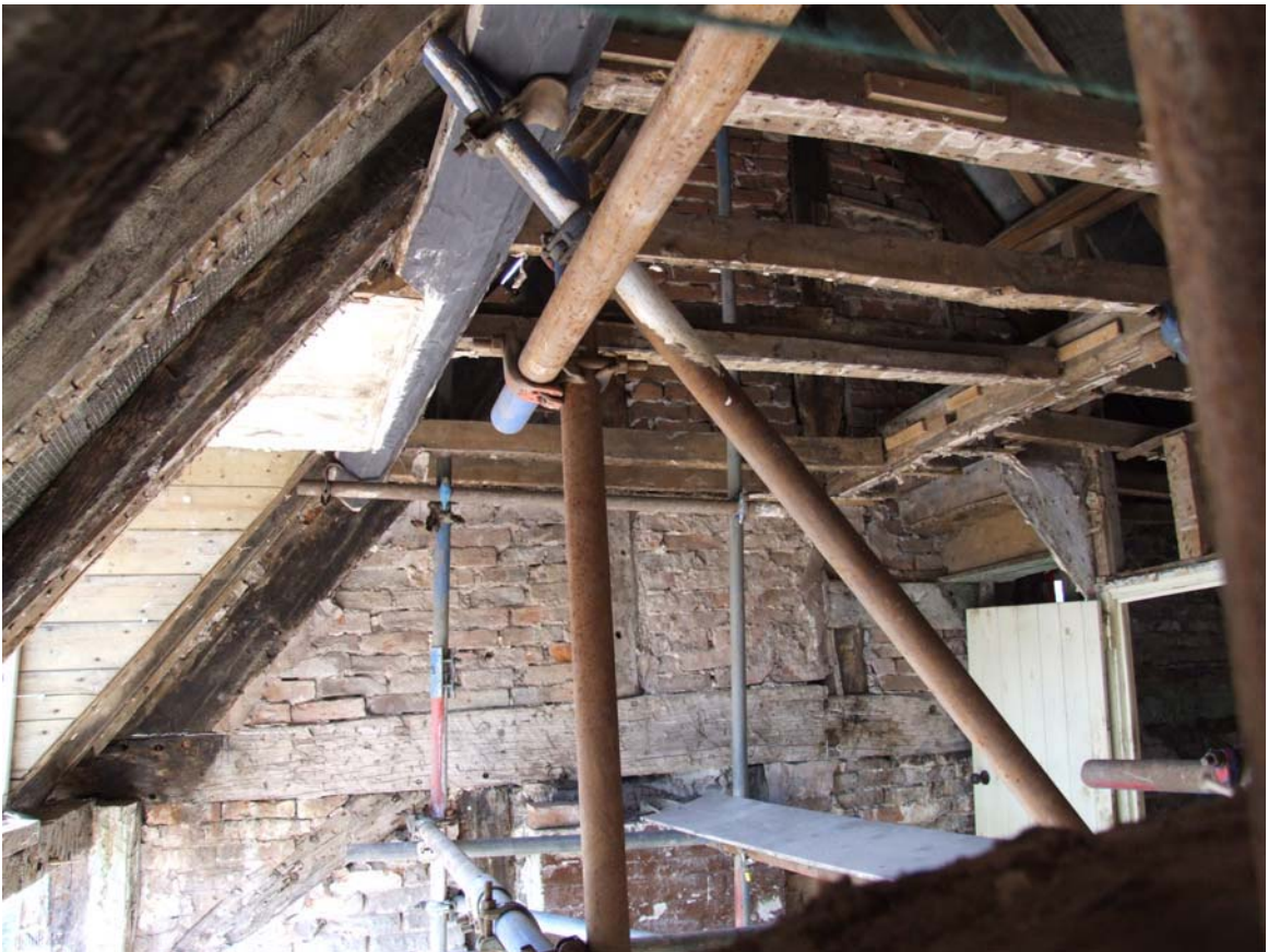
Plate 6: Truss T1 upper
