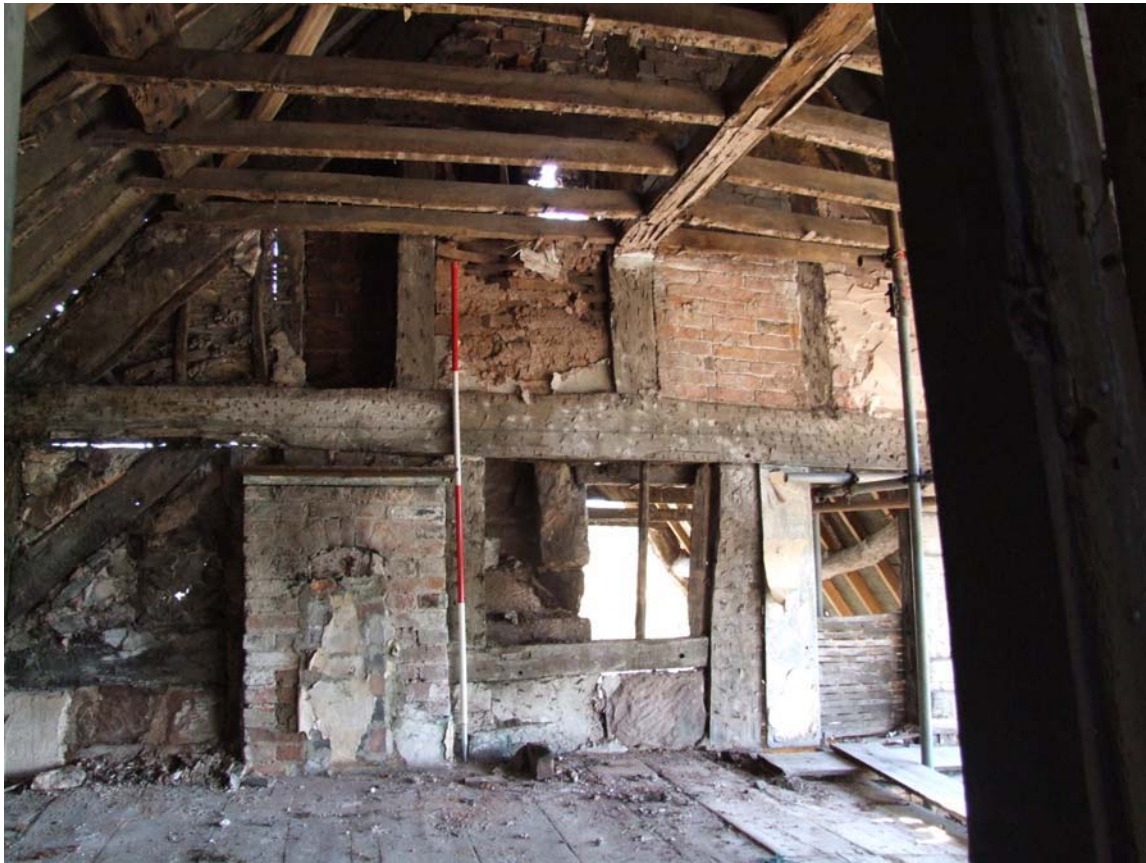
Plate 11: Truss T3 upper (scale 2-metres)
