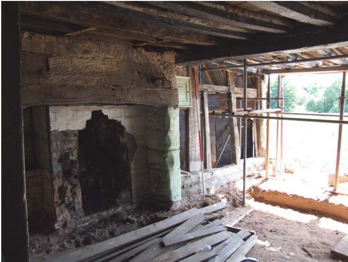
Plate 13: Frame T3 lower (scale 2-metres)
